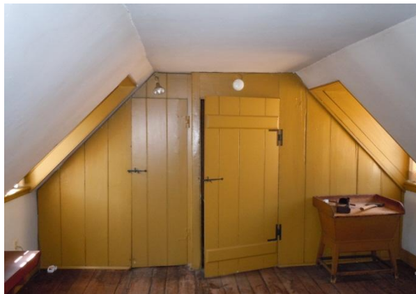
Figure 199, above. The painted wood board south wall of Room 304. (NPS, 2013)
