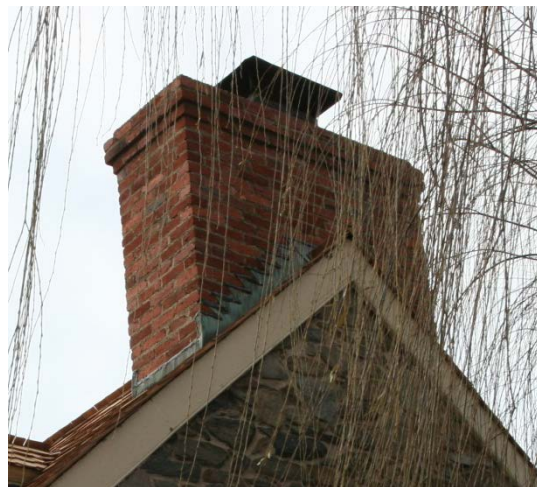
Figure 103. The north addition chimney was reconstructed in the 1950s restoration of the house. (NPS)
