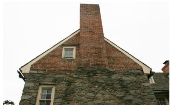
Figure 25. Chimney to stone transition on the east elevation of the main block. (NPS)
