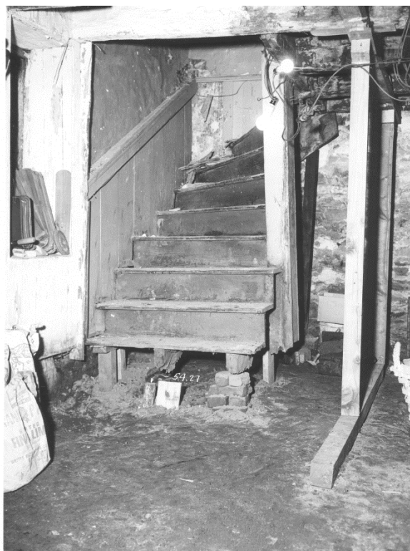
Figure 171. Stair 1 during NPS rehabilitation in 1956. (NPS)
