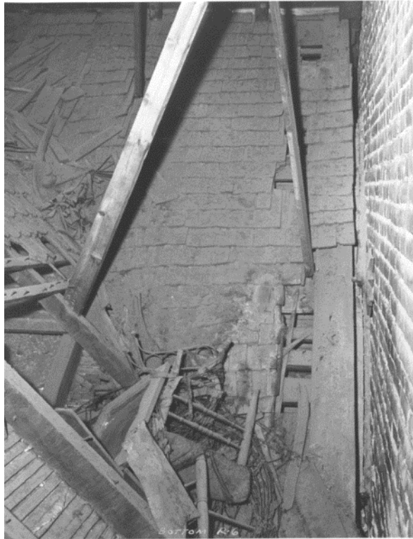
Figure 49. Area under the shed roof in 1956; note the brick wall of the adjacent west building. (NPS)
