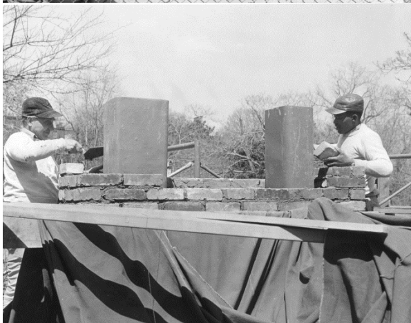
Figure 118. Chimney 2 during reconstruction. (NPS, 1957)
