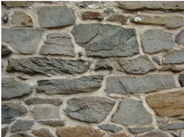
Figure 100. Bluestone masonry walls. (NPS)
