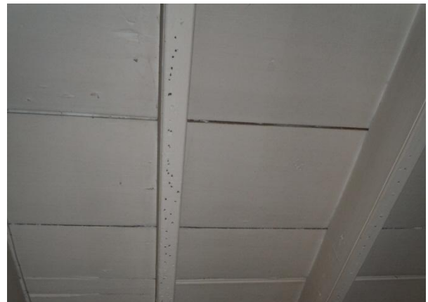
Figure 203, right. Exposed painted wood floor framing at ceiling in Room 201A would likely not have been exposed historically. Plaster was removed during 19050s restoration. (NPS, 2013)
