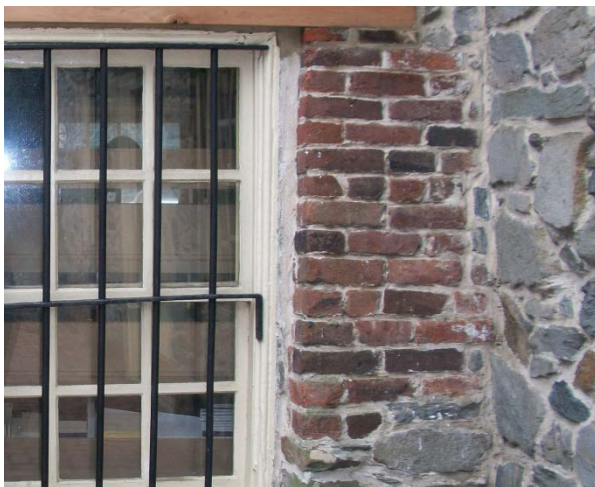
Figure 102. Brick patch on north elevation adjacent to W103. (NPS)
