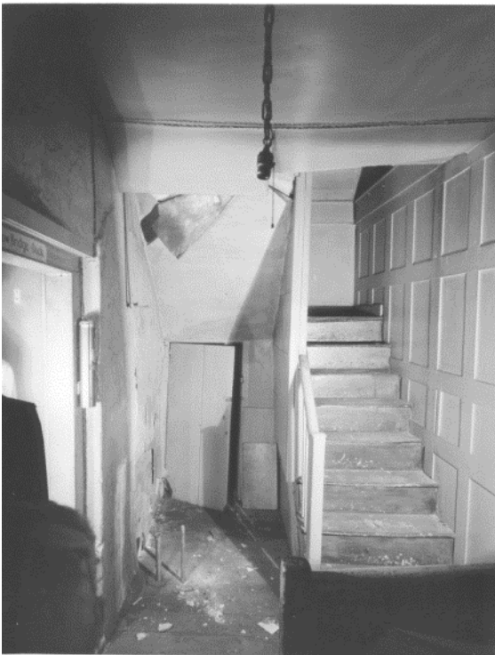
Figure 37. Room 201B, looking west to Stair 2. (NPS, 1955)
