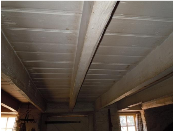
Figure 201, above. Exposed painted wood floor framing at ceiling in Room 102. (NPS, 2013)
