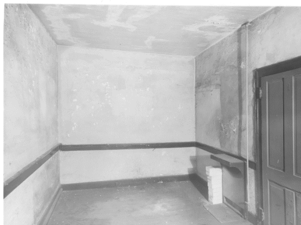
Figure 190. The depth of the north wall of Room 202 prior to the NPS restoration. (NPS, 1955)
