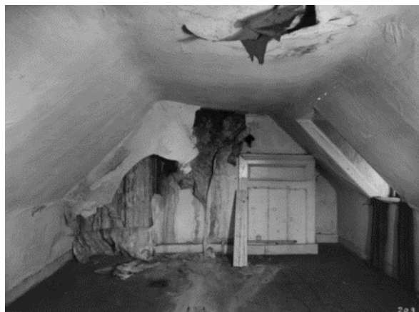
Figure 42. Room 304, looking north, in 1955. (NPS)
