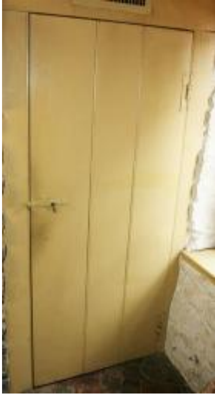
Figure 157. Typical board-and-batten wood door at D109. (NPS)
