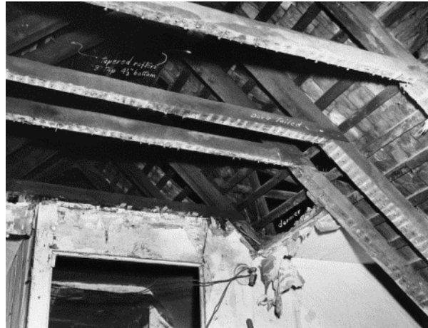
Figure 52. Exposed roof framing in 1956. (NPS)
