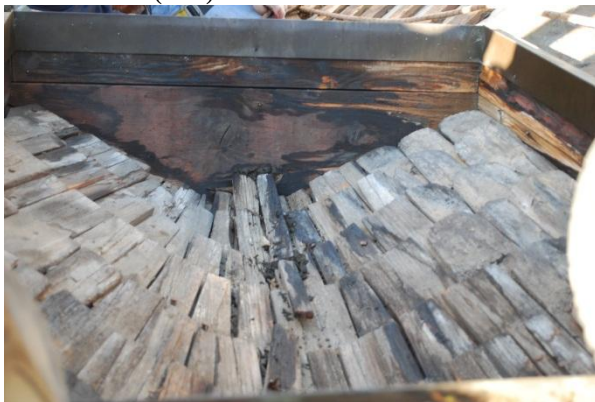
Figure 150. Historic shingles beneath skylight. (NPS, 2009)
