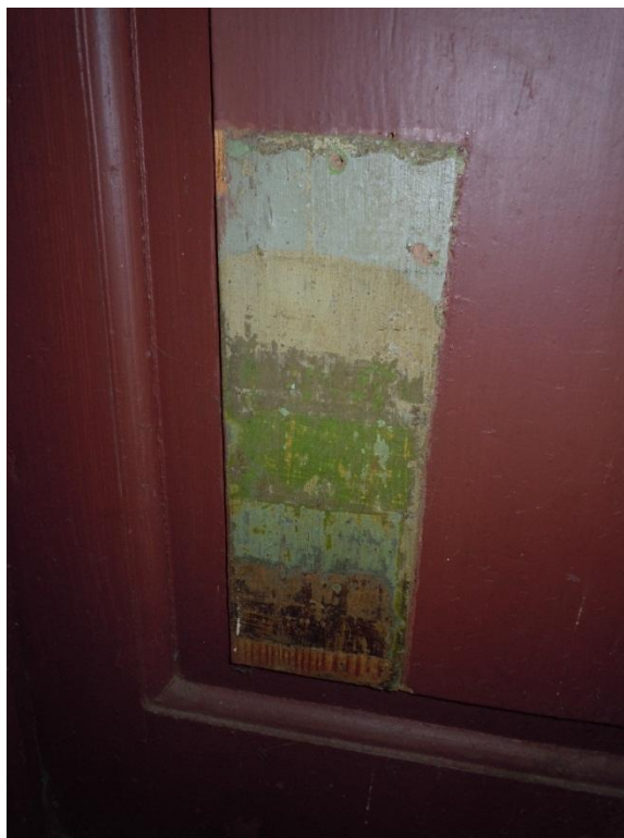
Figure 189. Historic paint exposures on wood paneling in Room 201B (not part of this HSR), which encloses Stair 1. (NPS, 2013)
