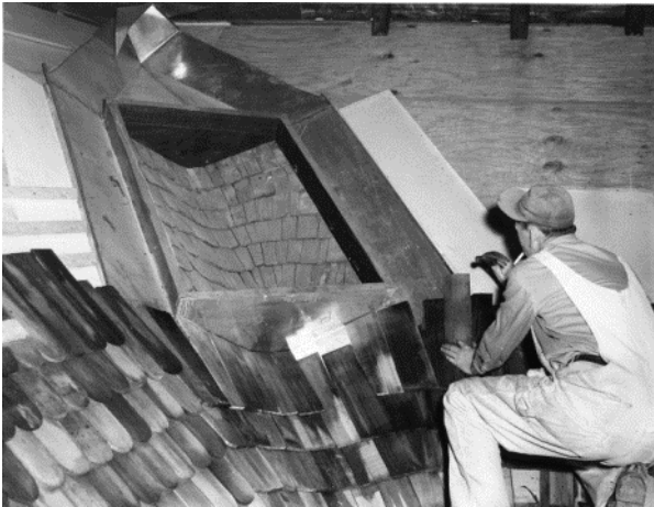
Figure 61, above. Installing a skylight over original roof shingles at the junction of the main block and the north addition, while the shed roof is still extant. (NPS, 1957)
