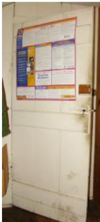
Figure 156. Board-and-batten door variation at D303 (back). (NPS)
