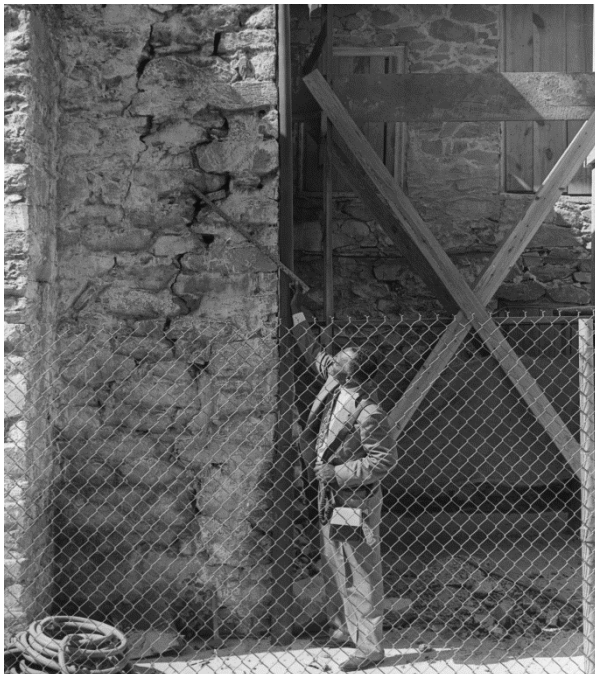
Figure 114. Bluestone masonry wall, west elevation. Some repointing is visible (upper left corner). (NPS)
