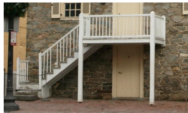
Figure 124. 1957 south elevation porch, constructed by the NPS, as seen in 2010.
