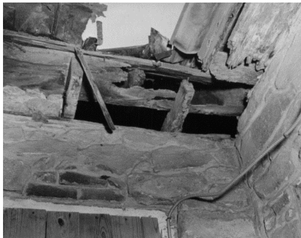
Figure 29. The cornices of the house were in disrepair when the NPS acquired the property, as seen in this 1955 photograph. (NPS)
