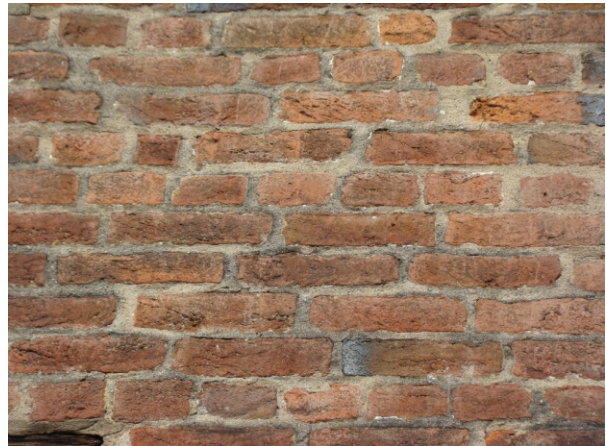
Figure 101. Brick in the east elevation gable. (NPS)
