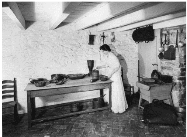
Figure 77. Room 102 after restoration was completed. (NPS, 1960)
