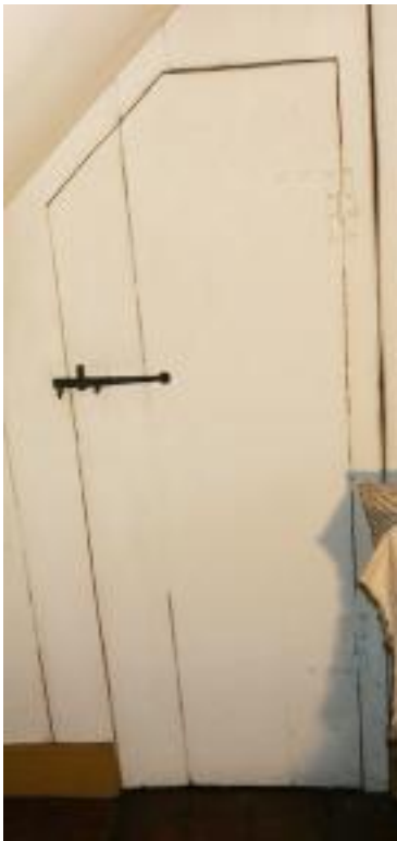
Figure 159. Original board-and-batten door at D306. (NPS)
