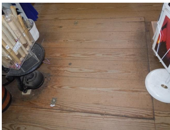
Figure 207. Wood floor in Room 101, with built-in door over archeological feature, was installed in the 1950s. (NPS, 2013)
