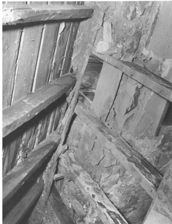
Figure 50. Roof sheathing in 1956. (NPS)
