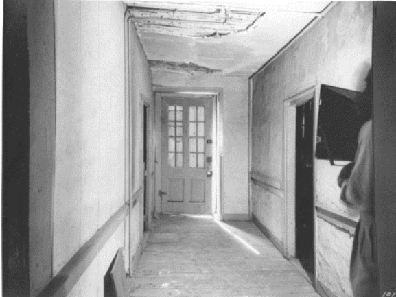
Figure 33. Room 201A, looking south to D2, in 1955. (NPS)
