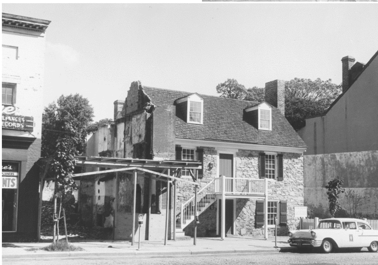
Figure 73. After the adjacent west building was removed, the shared wall was temporarily kept in place in order to properly reconstruct the west wall. (NPS, 1958)
