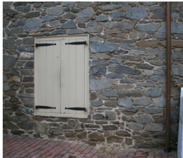
Figure 89. The stonework underneath W101 after repointing. (NPS, 2012)
