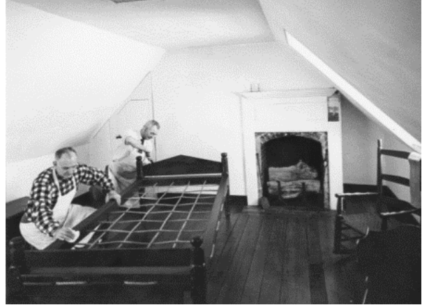
Figure 79. Room 304 after completion. (NPS, 1960)
