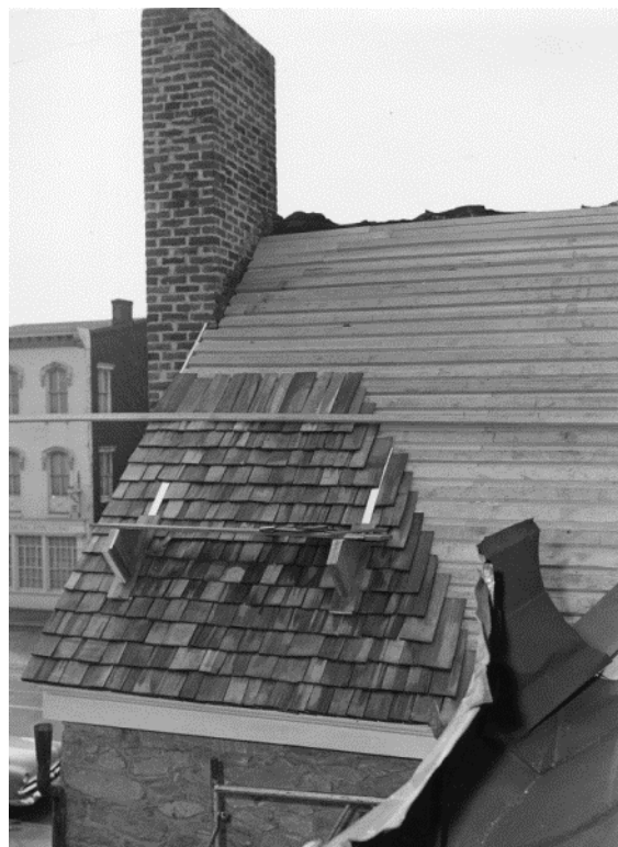
Figure 46. Reroofing the main block with square-butt wood shingles; note the former metal roof in the foreground. (NPS, 1956)
