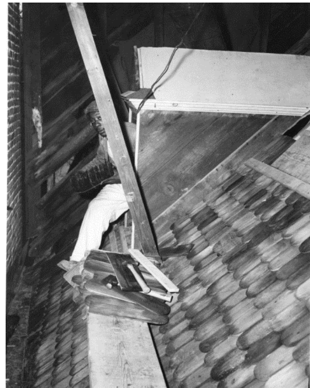
Figure 62, right. The installation of new wood roof shingles on the west slope of the north addition, while the shed roof is still extant. (NPS, 1957)
