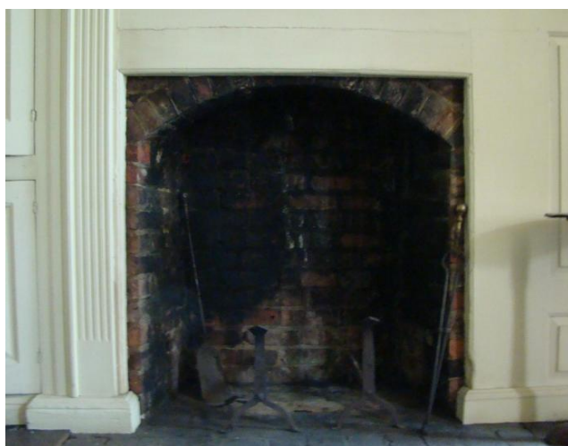
Figure 166, above. Fireplace D in Room 204. (NPS)
