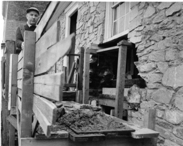
Figure 55. Repairing the stone masonry walls on the front elevation in 1957. (NPS)
