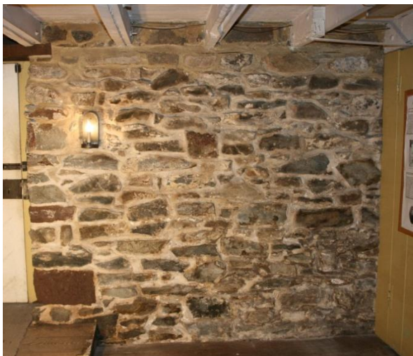
Figure 182. Unfinished blue stone walls in Room 101. (NPS)
