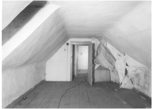
Figure 40. Room 303, looking west, in 1955. (NPS)
