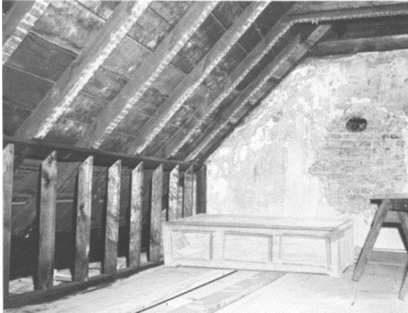
Figure 53. Room 303 in 1956, after lath and plaster was removed from the interior wall surfaces. (NPS)
