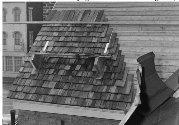
Figure 151. Roof replacement in 1956. (NPS)
