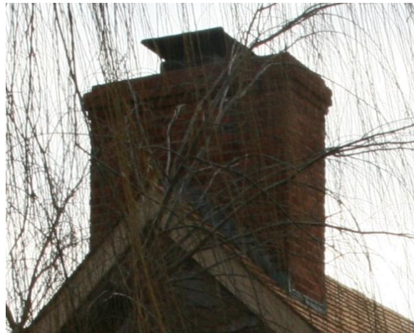
Figure 119. Chimney 2's partial cap today. (NPS)
