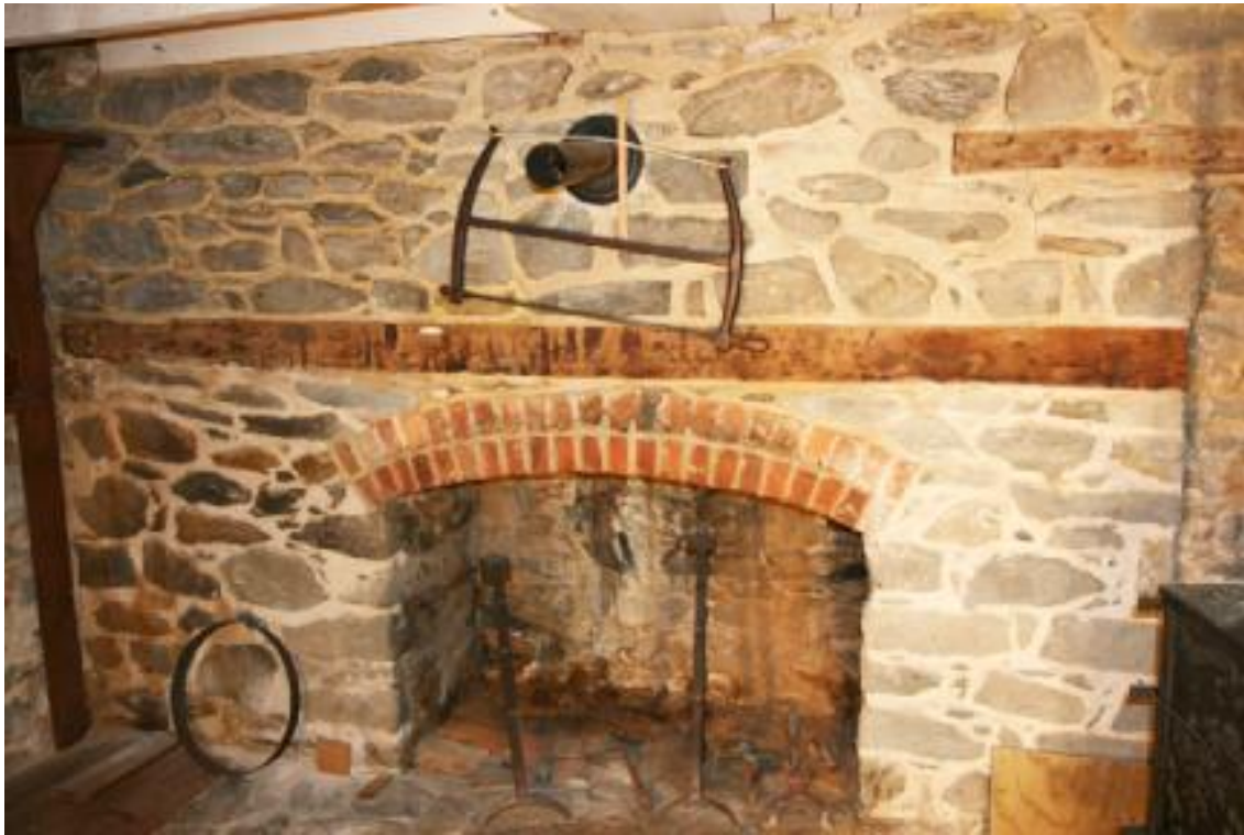
Figure 161. Fireplace A in Room 101. (NPS)
