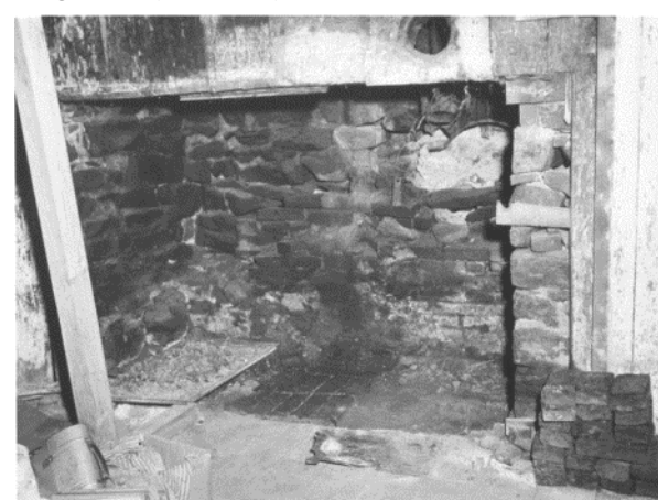
Figure 48, above. The fireplace in Room 102 in 1956. (NPS)
