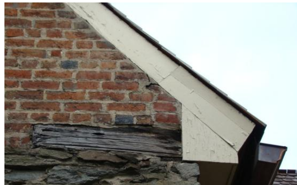
Figure 146. Detail of east elevation main block showing gable finish and trim.
