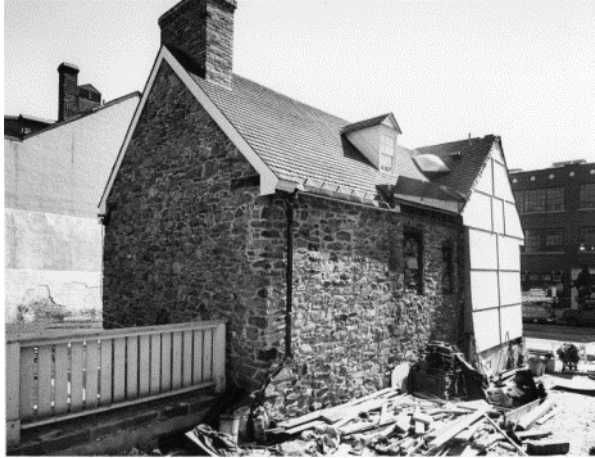
Figure 74. The west elevation of Old Stone House after the removal of the shared wall. (NPS, 1958)
