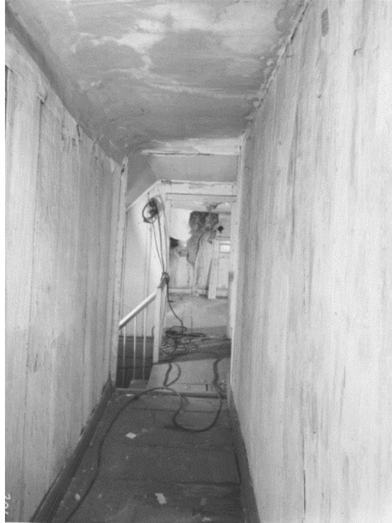
Figure 38. Room 301 looking north, in 1955. (NPS)
