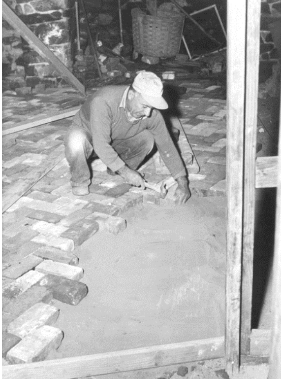
Figure 67. Laying brick over concrete slab-on-grade in Room 102 in 1957. (NPS)
