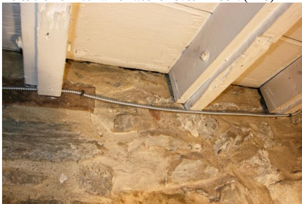
Figure 108. Sistered joists in Room 101.
