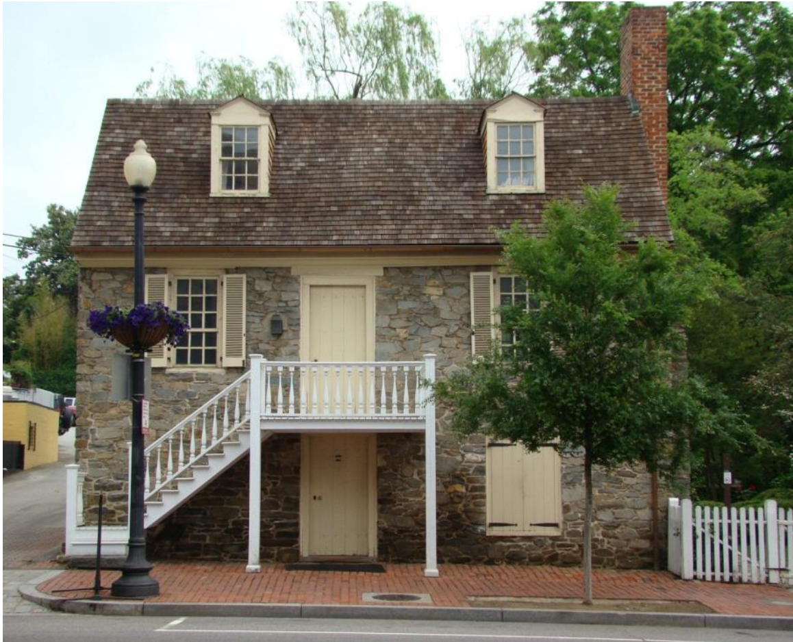
Figure 28. The dormer windows are symmetric, but do not align with the windows on the second floor. (NPS)
