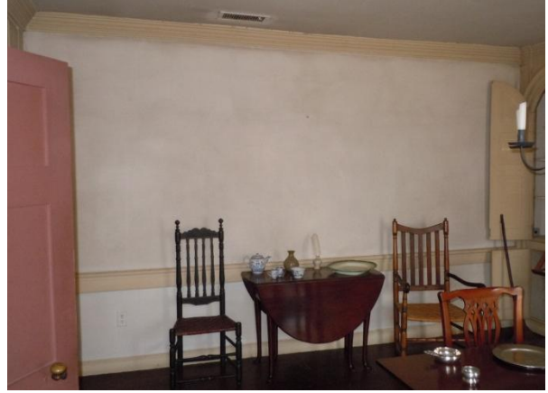
Figure 193. One of the plaster walls in Room 204. (NPS, 2013)
