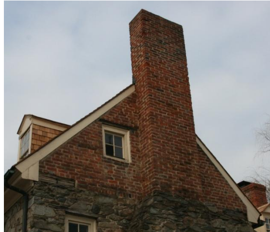
Figure 115. Brick running bond under east gable, main block. Note: this chimney is Chimney 1. (NPS)
