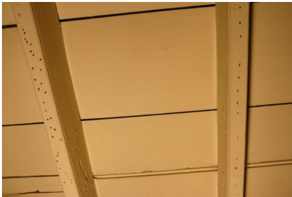
Figure 106. Joists in Room 201A exhibiting bead detail. Holes are from lath which was removed in 1957. (NPS)
