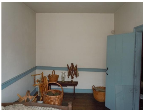
Figure 191. The depth of the north wall of Room 202 after the NPS restoration. (NPS, 2013)
