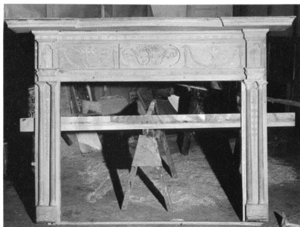
Figure 71, above. Room 203's fireplace surround removed for repair. (NPS, 1957)
