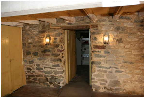
Figure 110. Room 101, looking north. Original exterior wall of the main block, now an interior load-bearing wall.
