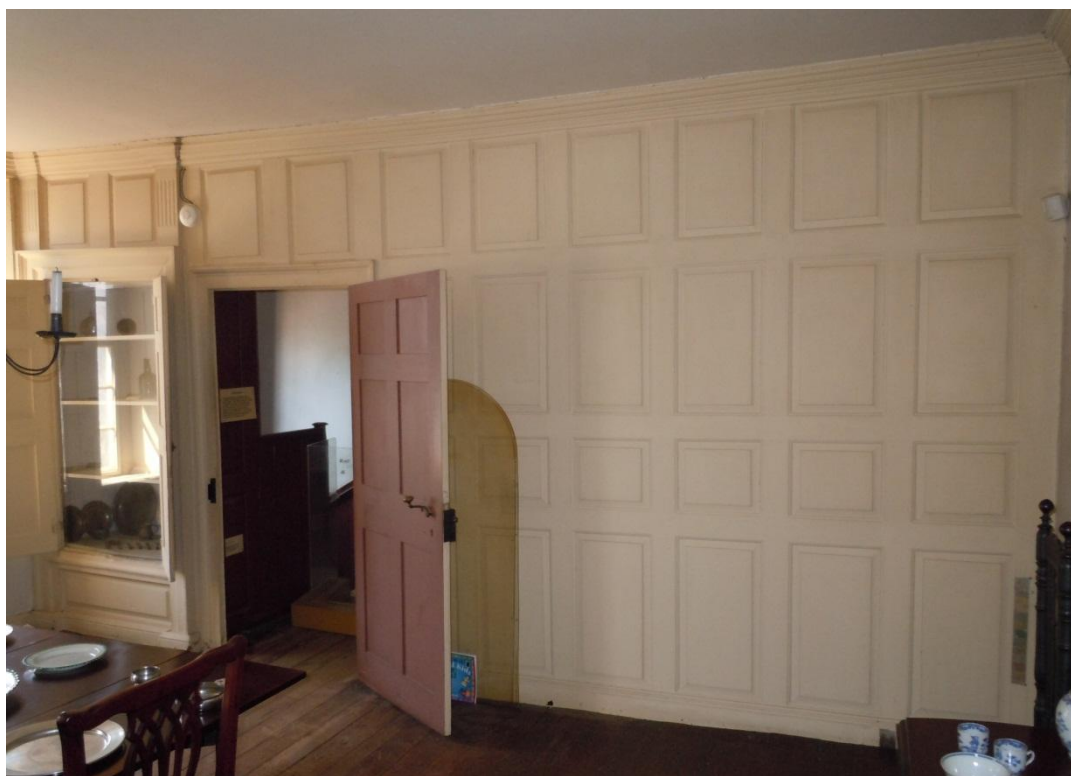
Figure 196. The painted wood paneled south wall of Room 204. (NPS, 2013)
