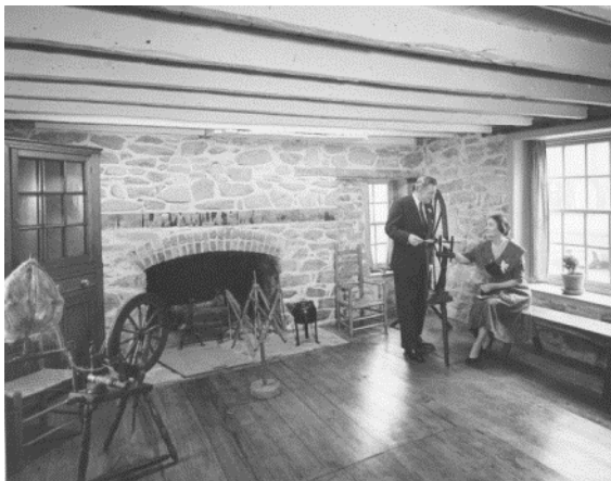
Figure 76. Room 101 after restoration was completed. (NPS, 1960).
