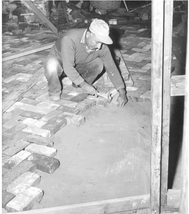
Figure 208, above. The herringbone brick floor of Room 102. (NPS, 2013).
