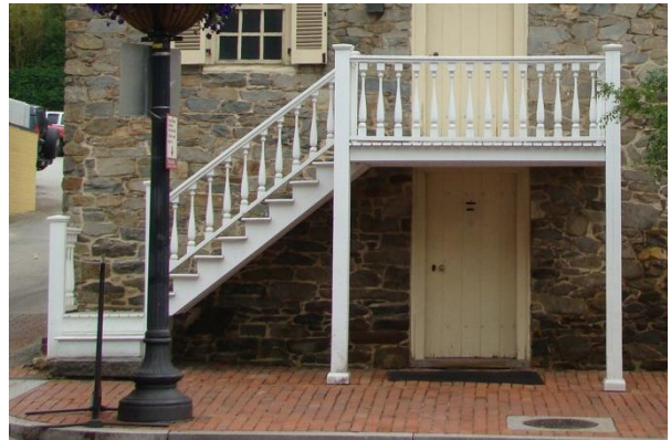
Figure 120. New porch and stair in 2012. (NPS)
