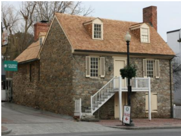
Figure 80. South and west elevations of the house after the new roofs were installed. (NPS, 2009)
