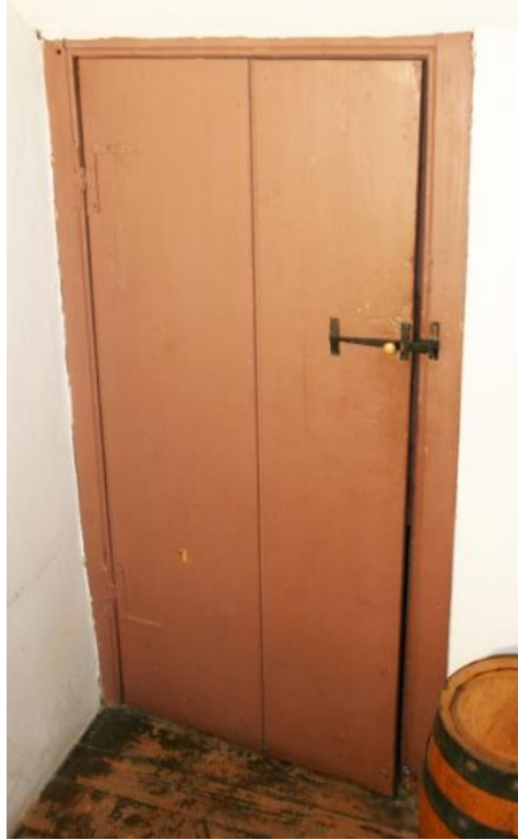
Figure 158. Original board-and-batten door at D205. (NPS)
