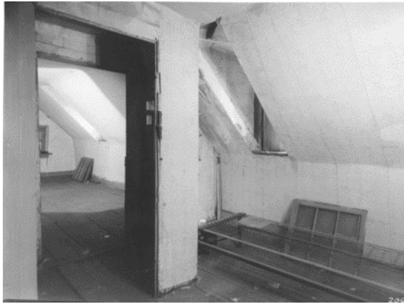
Figure 39. Room 302, looking east, in 1955. (NPS)
