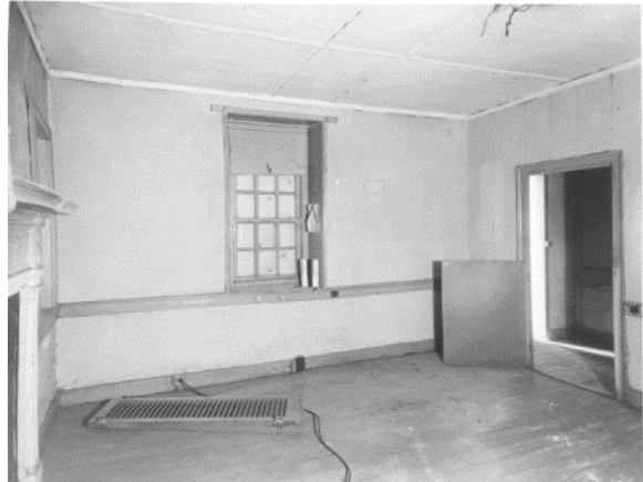
Figure 36. Room 203, looking south, in 1955. (NPS)
