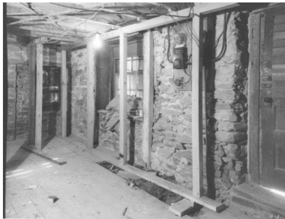
Figure 31. Room 101, looking south, in 1955. (NPS)
