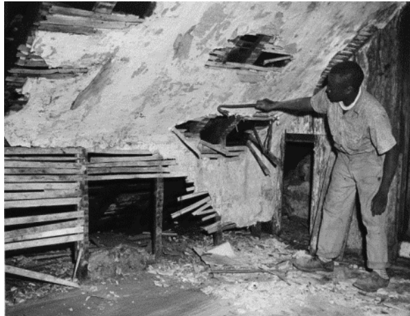
Figure 51. Removing plaster on the third floor in 1956. (NPS)
