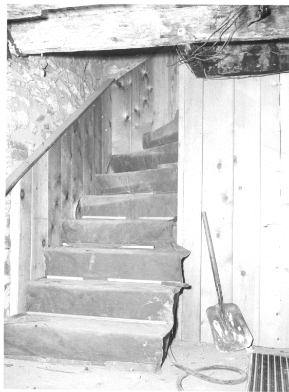
Figure 172. Stair 1 during rehabilitation 1957. (NPS)
