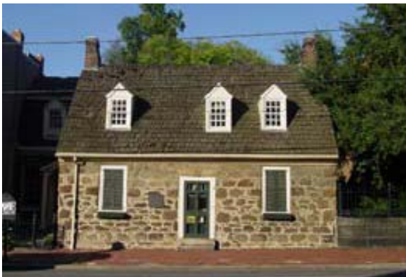
Figure 24. This ca. 1754 house in Richmond, VA provides a visual representation of how Old Stone House may have appeared if initially constructed as a one-and-one-half story structure. ( www.nps.gov/nr/travel/richmond/OldStoneHouse/htm )
