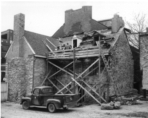
Figure 57. The north addition dormers being restored in 1957. (NPS)
