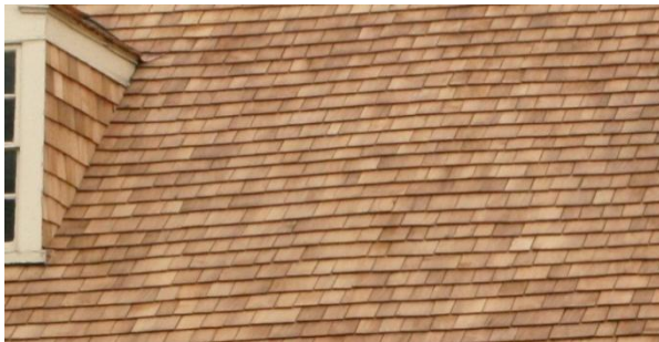
Figure 148. Square-butt shingles were installed on the main block in 2009. (NPS)
