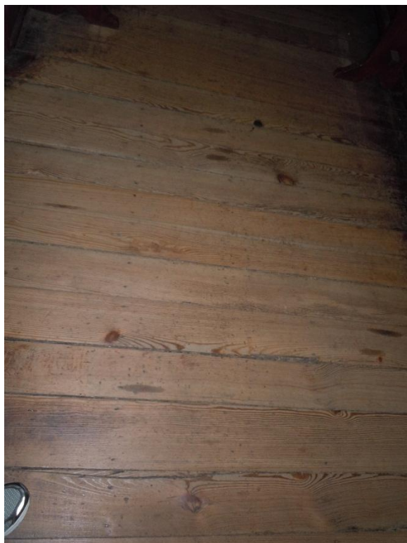
Figure 204. Random-width wood floor in Room 201A; note worn surfaces. (NPS, 2013)
