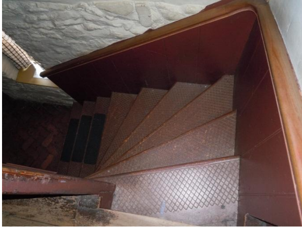
Figure 173, above. Detail of Stair 1 winder treads from the second floor. (NPS, 2013)
