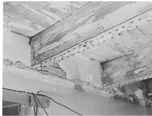
Figure 107. Joists in Room 203 exhibiting bead detail, over W7. (NPS, 1955)
