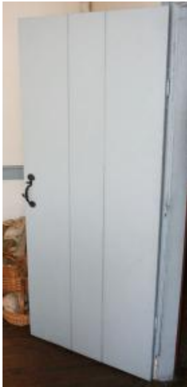
Figure 155. Typical board-and-batten wood door at D202. (NPS)
