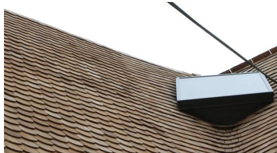
Figure 149. Round-butt shingles were installed on the north addition in 2009. The skylight covers historic shingles. (NPS)
