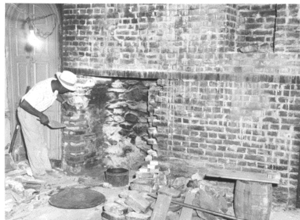
Figure 70. Repairing brick walls in Room 204 after interior wood paneling was temporarily removed. (NPS, 1957)
