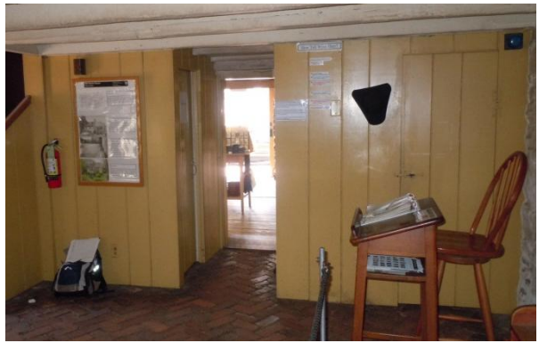
Figure 185. Painted wood board walls in Room 102, separating Rooms 103 and 104. (NPS, 2013)
