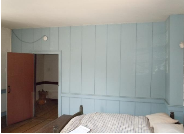
Figure 192. The painted wood board wall in Room 203. (NPS, 2013)
