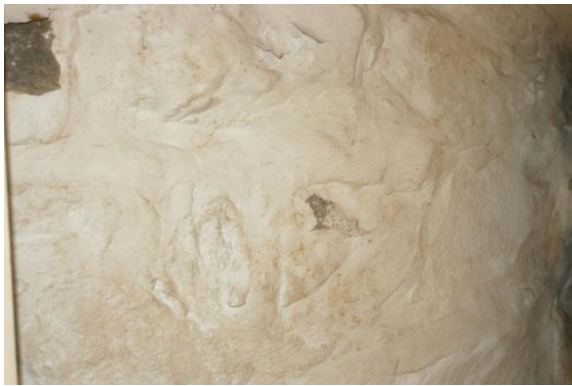
Figure 184. Whitewashed bluestone in Room 102. (NPS, 2013)
