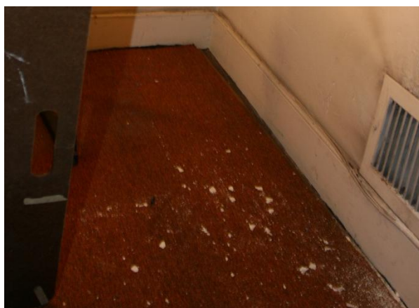
Figure 206. Carpet covers wood floors in Room 302. (NPS)
