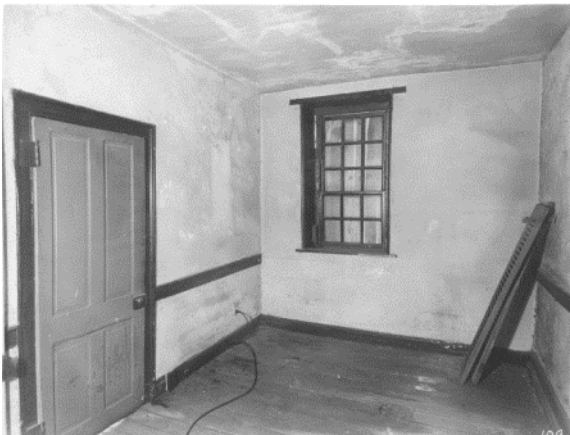
Figure 35. Room 202, looking south, in 1955. (NPS)
