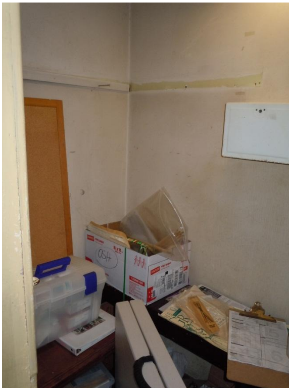
Figure 186. The interior of Room 103 with its plastered walls. (NPS, 2013)
