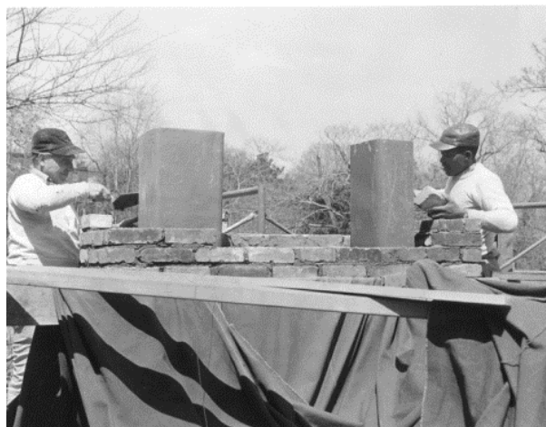
Figure 58. Reconstruction of the north addition chimney with terra cotta flue liners. (NPS, 1957)
