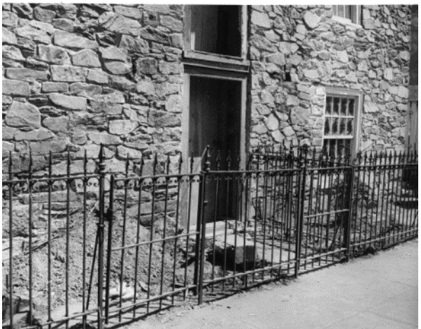
Figure 56. The front elevation after the porch and stair were removed. (NPS, 1957)
