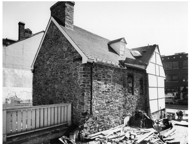
Figure 117, above. The west elevation after the demolition of the adjacent west building. The brick partition wall has been framed, but not clad with stone. (NPS, 1958)
