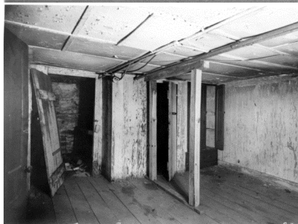
Figure 32. Room 101, looking west, in 1955. (NPS)
