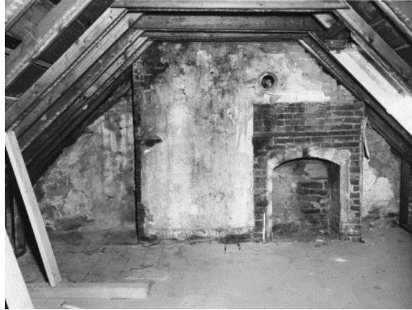
Figure 54. Room 304 in 1956, after lath and plaster was removed from the interior wall surfaces; note the removal of the fireplace surround. (NPS)
