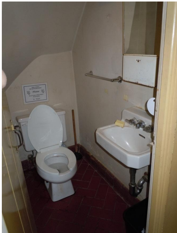
Figure 187. The interior of Room 104 with its plastered walls. (NPS, 2013)
