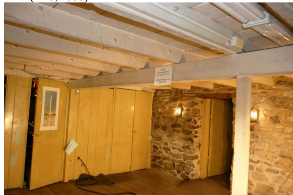
Figure 109. Room 101 joists and support system.
