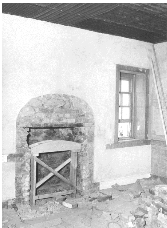
Figure 72, right. Room 203's fireplace without surround in place. (NPS, 1957)
