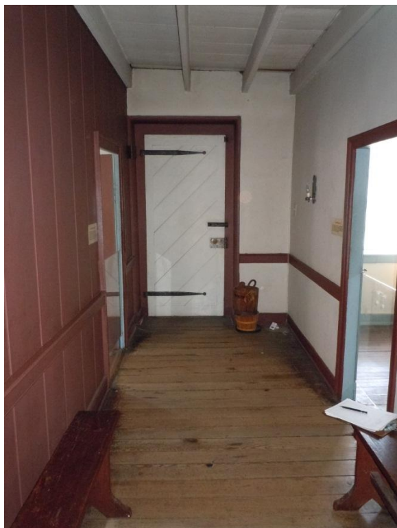
Figure 188. Room 201A includes plastered walls and painted board walls. (NPS, 2013)
