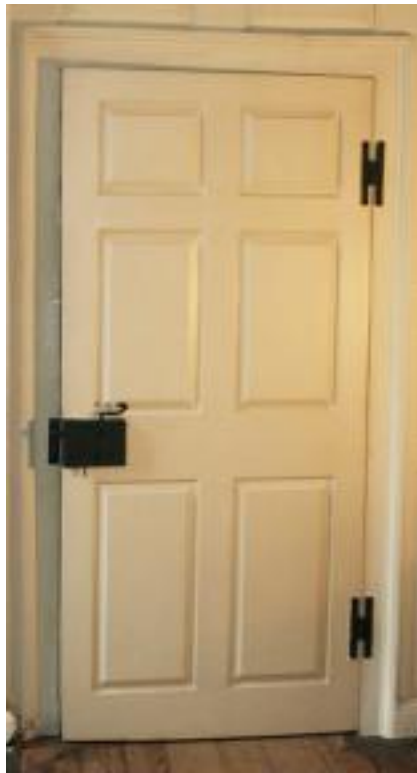
Figure 160. Replacement panel door at D204. (NPS)
