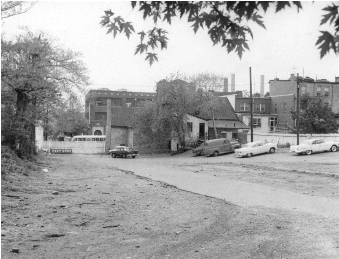
Figure 17. The rear of Old Stone House in 1956 showing the condition after it was purchased by the NPS. (NPS)
