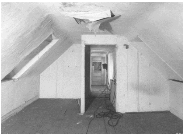
Figure 41. Room 304, looking south, in 1955. (NPS)
