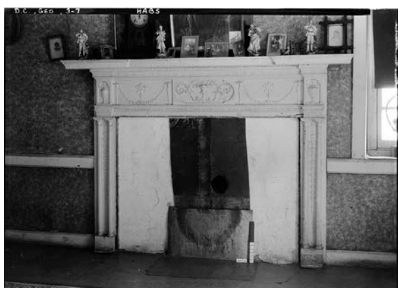
Figure 11. The fireplace in Room 203 in 1935. (HABS, Library of Congress)
