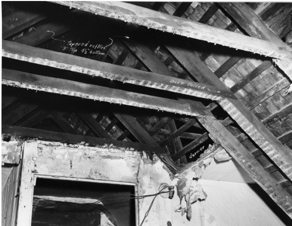
Figure 113. Roof framing exposed in Room 303, looking east. Note the random-width sheathing boards that appear to be in excess of 1'-0" widths. (NPS, 1956)
