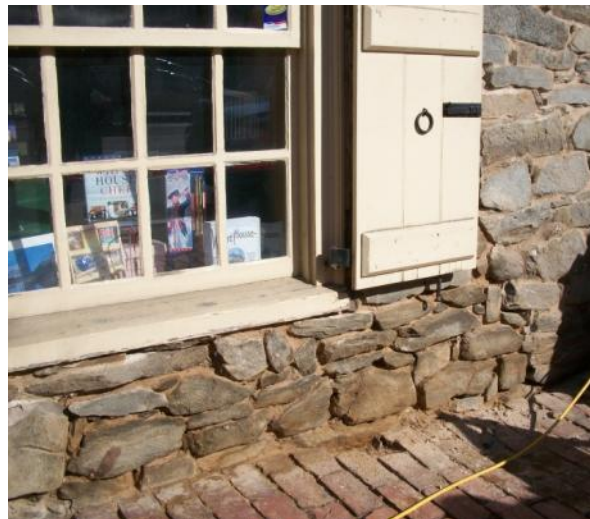
Figure 88. The stonework underneath W101 prior to repointing. (NPS, 2012)
