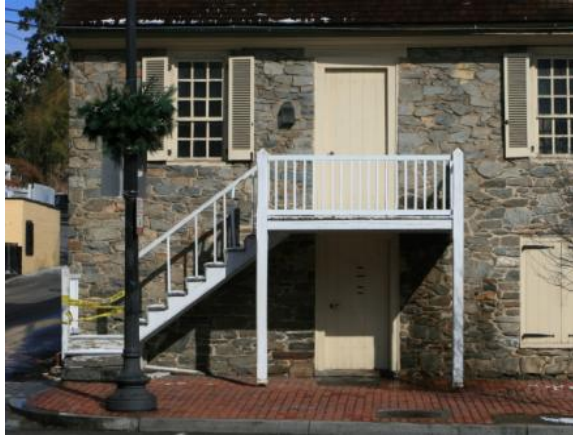
Figure 82. The front porch and stair prior to reconstruction. (NPS, 2011)
