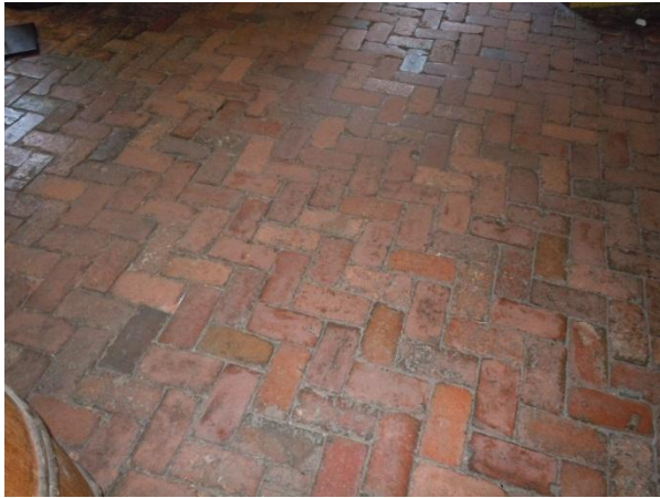
Figure 208, above. The herringbone brick floor of Room 102. (NPS, 2013).
