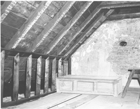
Figure 112. Roof framing exposed in Room 304, looking north. (NPS, 1956)
