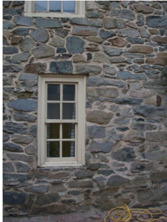
Figure 87. The same area after repointing work was completed. (NPS, 2012)
