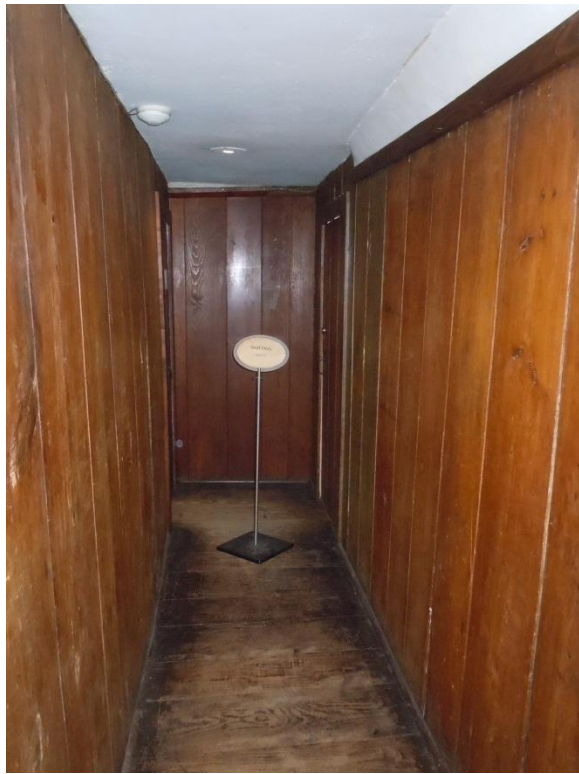
Figure 197. Unpainted wood board walls of Room 301. (NPS, 2013)
