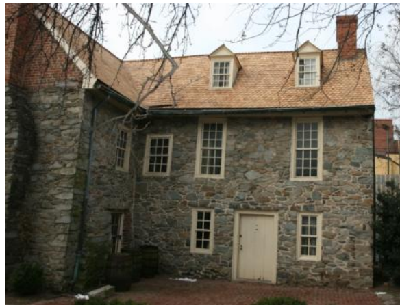
Figure 81. North and east elevations of the house after the new roofs were installed. (NPS, 2009)
