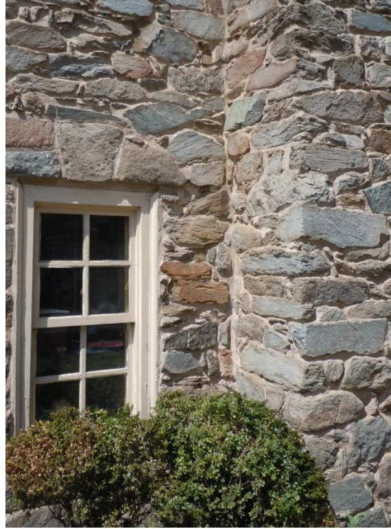
Figure 91. The same junction after repointing was completed. (NPS, 2013)
