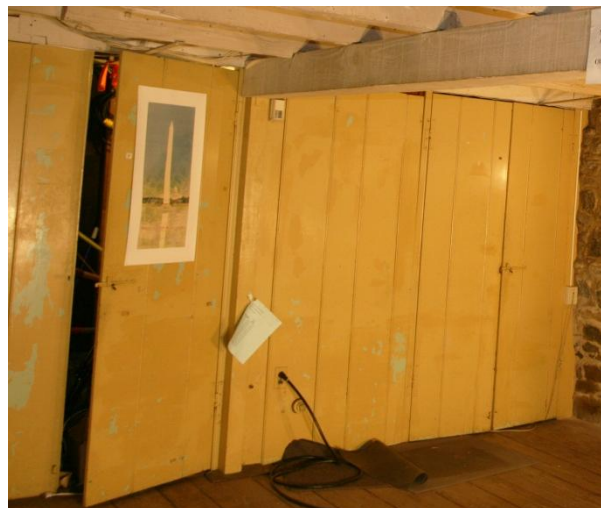
Figure 183. Painted wood board wall in Room 101 enclosing storage closets. (NPS)
