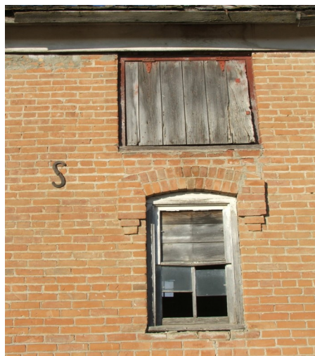
Above bottom window is a soldier brick arch above . A hayloft door is situated at the top of brick wall .
