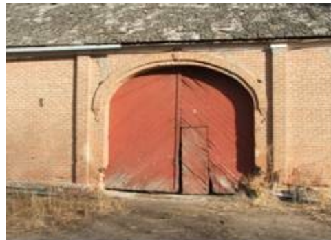
The west wall of west wing showing the arched doorway .
