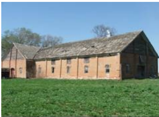
A NW, SE corner view of the barn.
