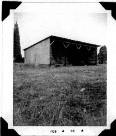
7. Front and side of 2nd Machinery Shed
