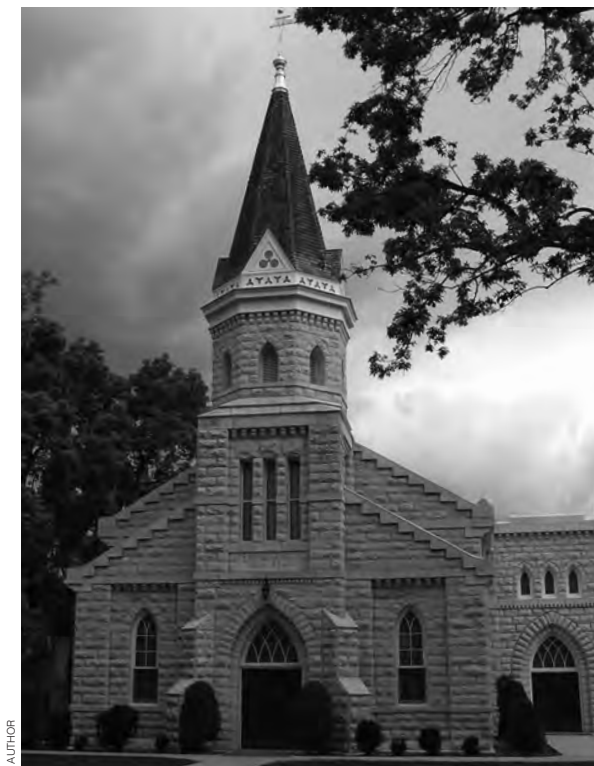
The Spring City Chapel was constructed of oolite limestone between 1902 and 1911.
