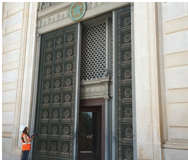
Steel Pocket Doors. Photo: OMES.
