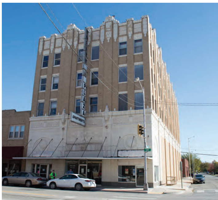
Hayes-Kennedy-Rivoli Theater Building. Photo: SHPO
