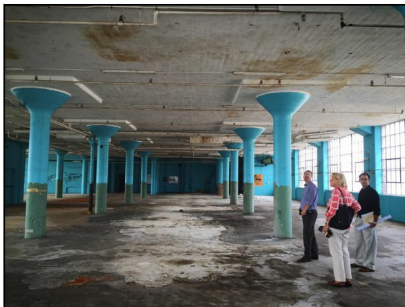
Members of the project team assess reuse options in an addition to Mill #1
