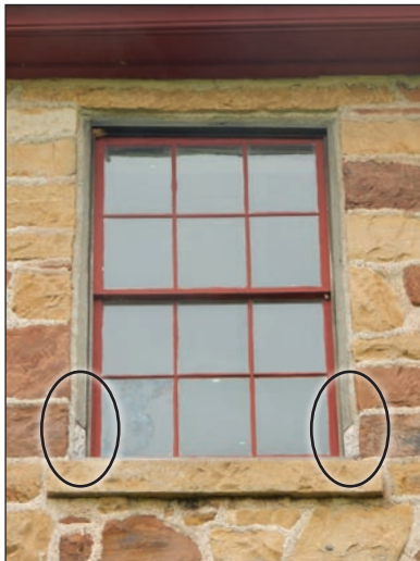
Figure 105: Window 205, second floor. Dutchman repairs (circled).
