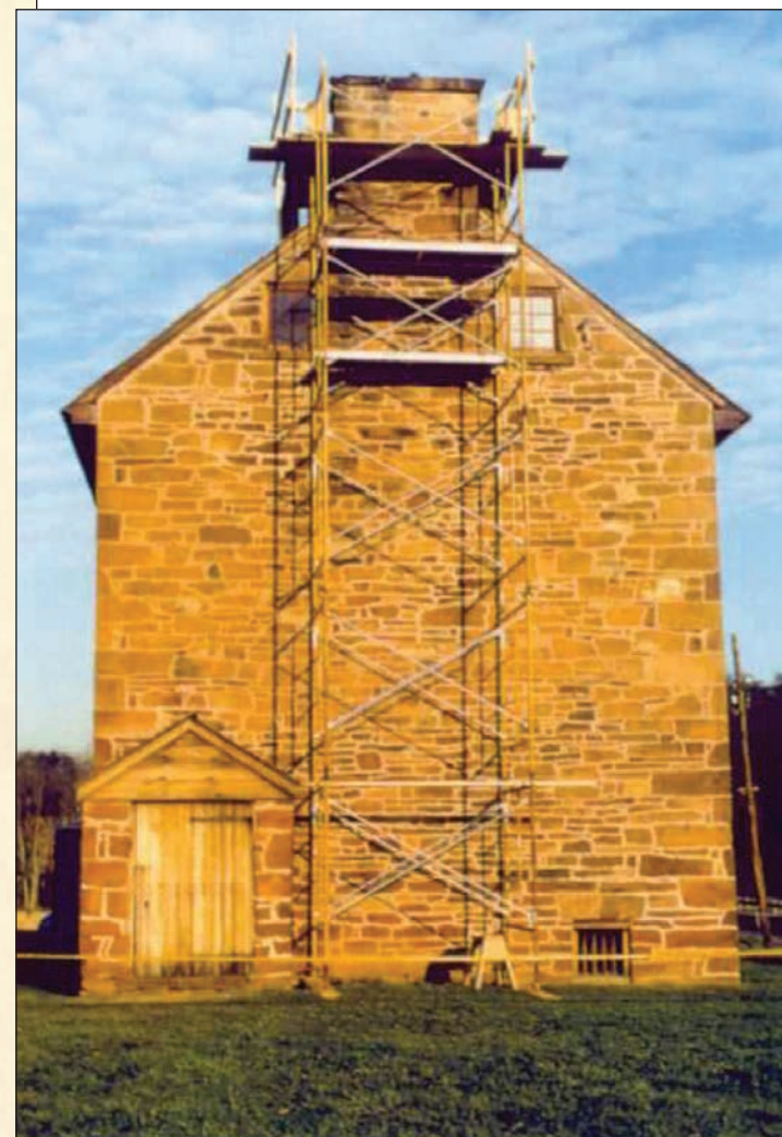
Figure 41: (left) Old Stone House chimney repair and reroofing project report, 1993; (above) Stone House west chimney prior to installation of blue stone chimney cap.
