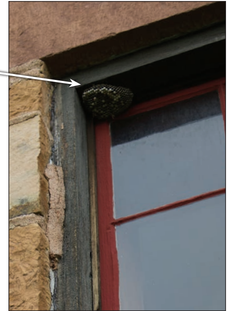
Figure 95: Window 102 insect nest detail.
