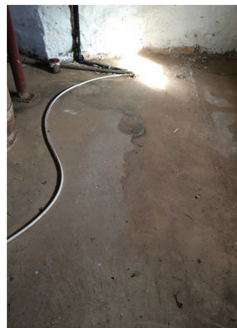
Figure 81: Concrete floor, basement, east side, 002.
