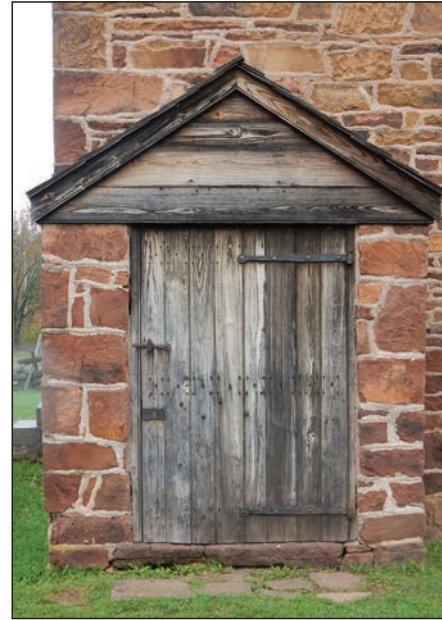
Figure 115: Door 001A, west elevation.
