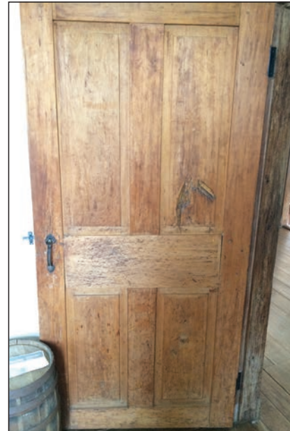
Figure 119: Dining Room door 103A.
