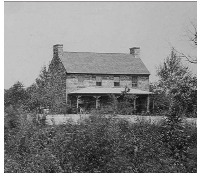
Figure 19: Stone House ca. 1903 with front porch, south facade.
