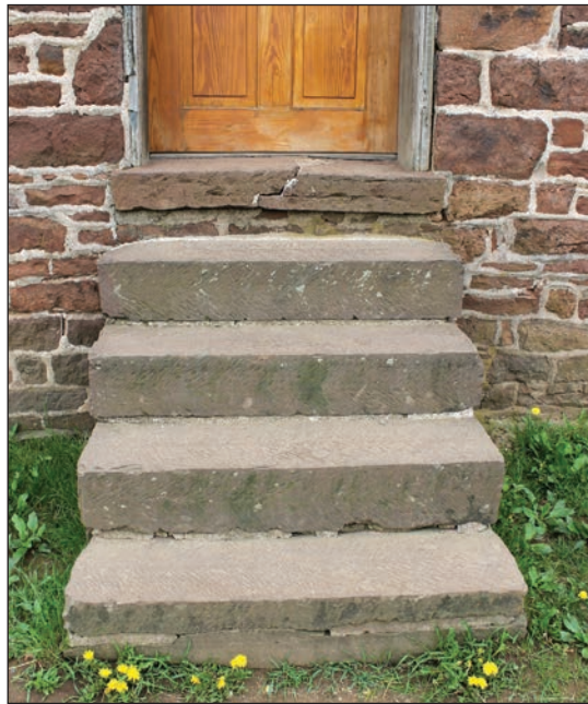
Figure 90: North exterior stairs.
