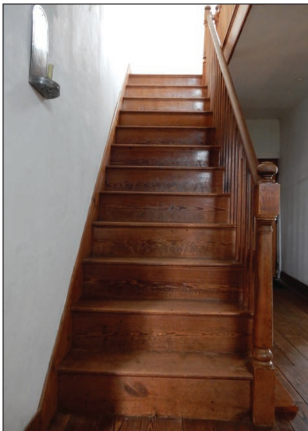
Figure 120: First floor stairs.
