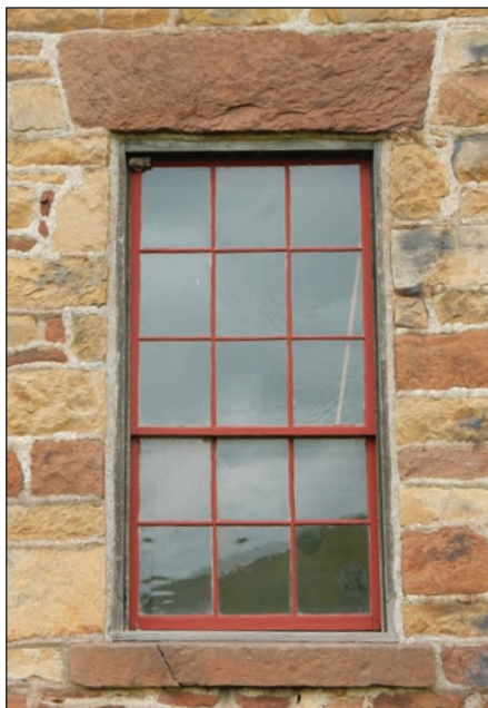
Figure 97: Window 104, first floor, north elevation.
