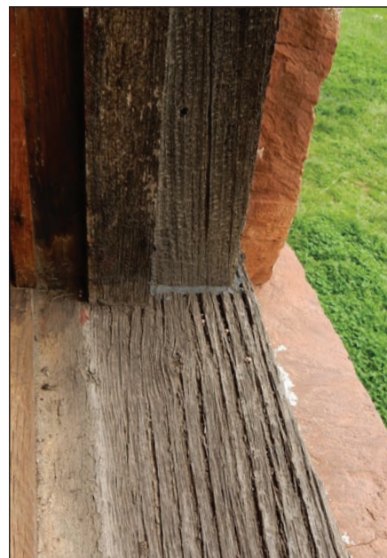
Figure 100: First floor window 102 representative of sill condition of south elevation windows 101, 102, and 103. Require linseed oil application.
