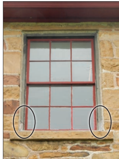
Figure 106: Window 206, second floor. Dutchman repairs (circled).
