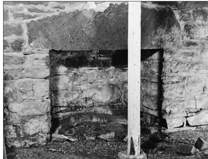
Figure 21: Column and footing in basement.
