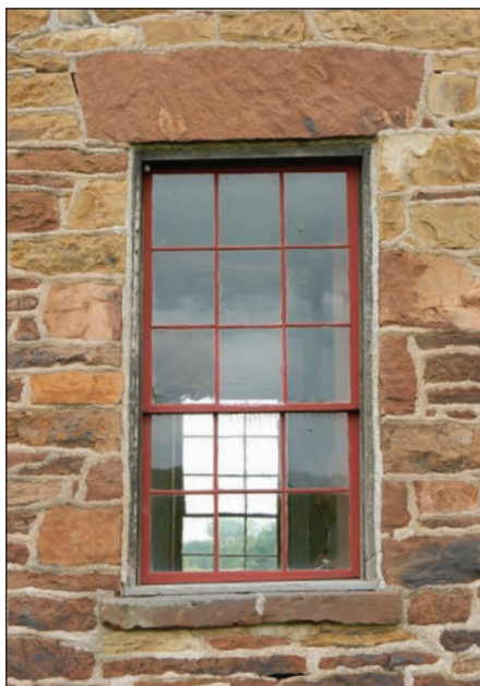
Figure 99: Window 106, first floor, north elevation.
