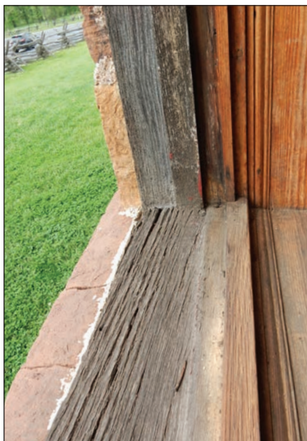
Figure 100: First floor window 102 representative of sill condition of south elevation windows 101, 102, and 103. Require linseed oil application.
