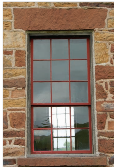
Figure 98: Window 105, first floor, north elevation.
