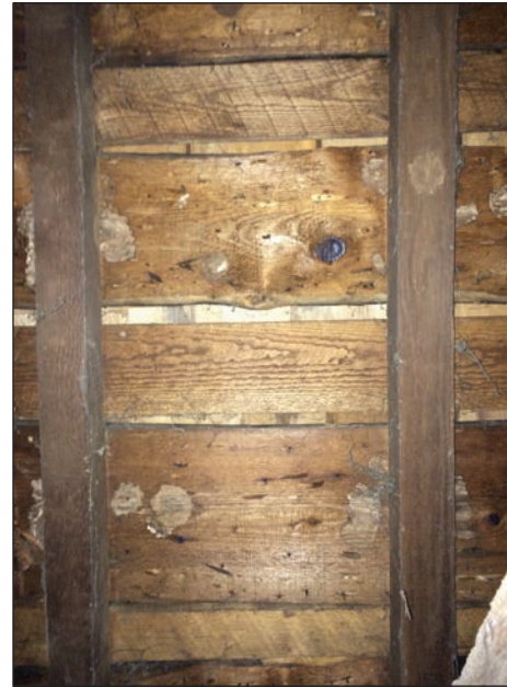
Figure 60: Sheathing and shingles.
