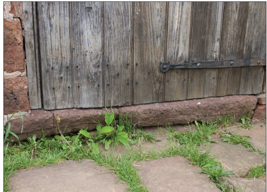
Figure 78: Threshold of door 001A, from west elevation to basement.
