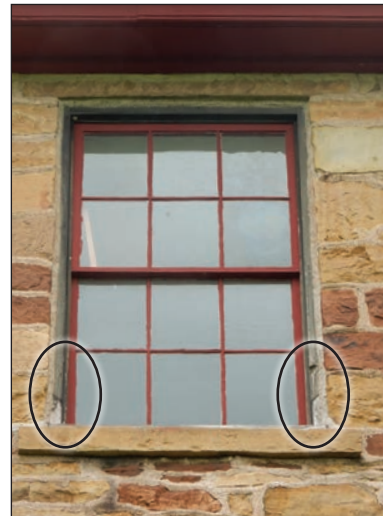
Figure 107: Window 207, second floor. Dutchman repairs (circled).
