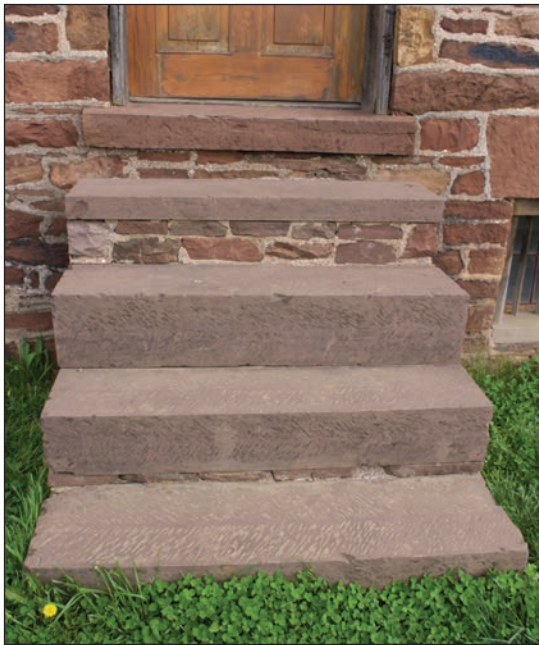
Figure 89: South exterior stairs.
