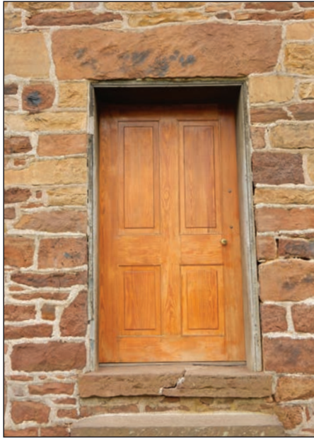
Figure 113: Door 101B, north elevation.
