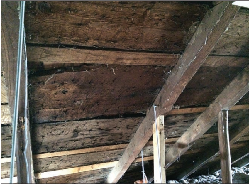
Figure 59: Sheathing, shingles and shoring of the roof of the Stone House.
