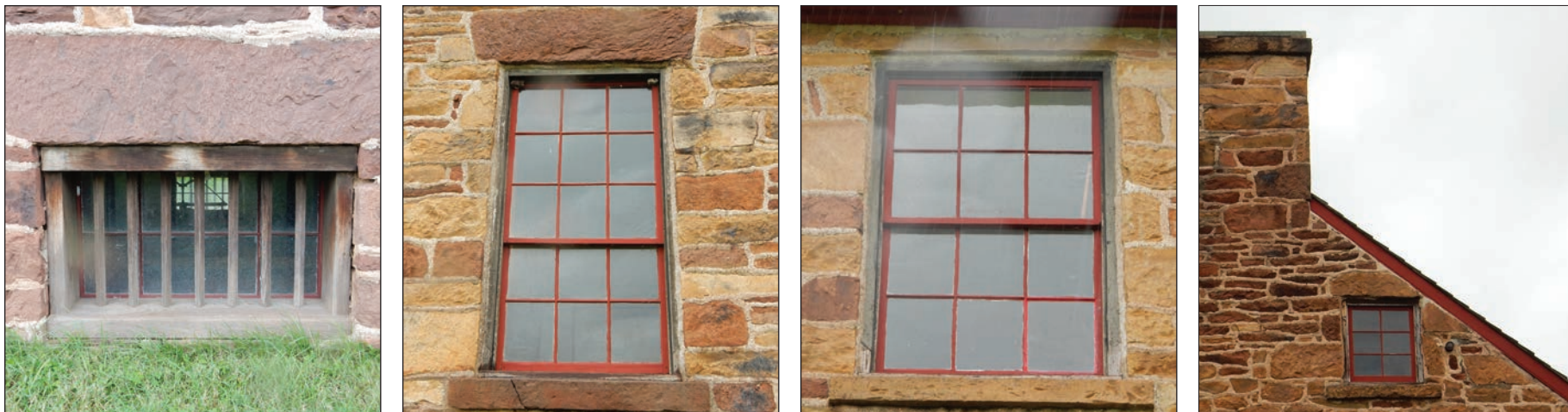
Figure 48: (left to right) Basement window, first floor window, second floor window, and attic window.
