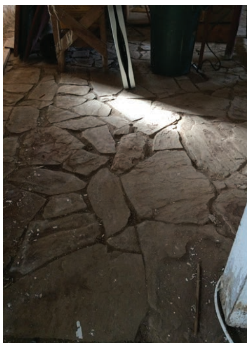
Figure 80: Stone floor, basement, west side, 001.
