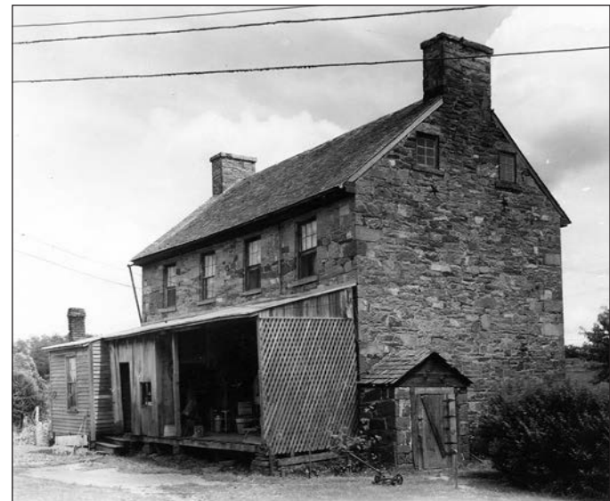
Figure 20: Stone House ca. 1940 with 1902 kitchen addition and porch, north facade.
