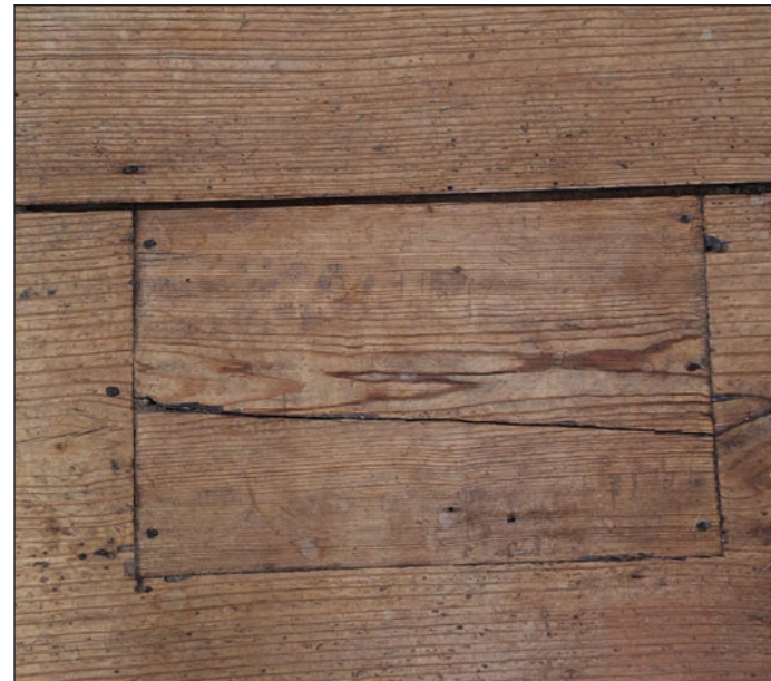
Figure 86: Location of former vent register in Bedroom 202.
