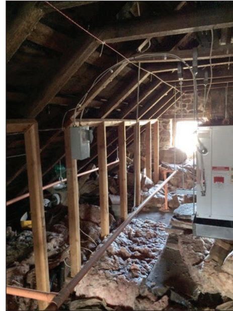
Figure 62: 2015 east gable end with rafter bracing.
