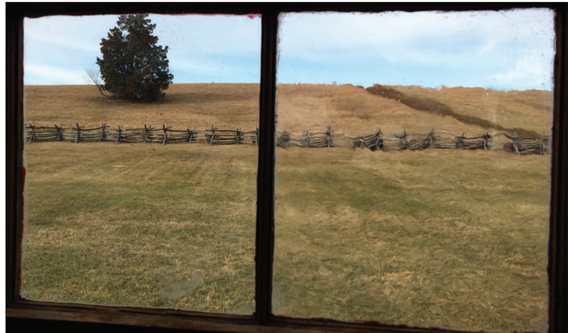
Figure 39: Reproduction (left) vs. antique (right) glass.
