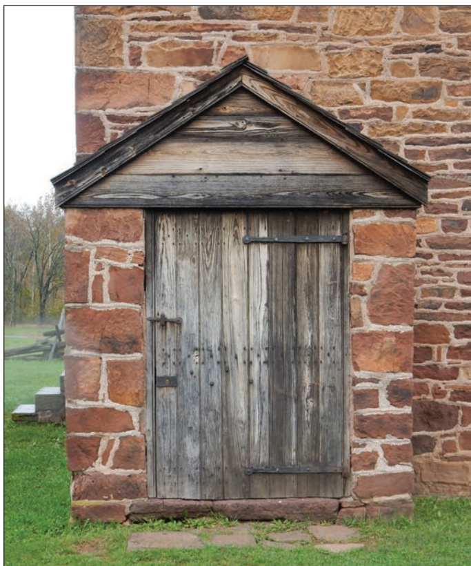
Figure 49: Basement entry at northwest corner of Stone House.
