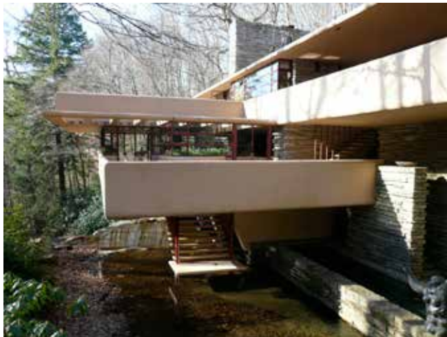
Figure 5: Fallingwater's reconstructed stairs to the stream. The stairs between the east living-room terrace and pottery terrace are also visible
