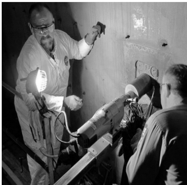
Figure 15: Removing a 5-inch diameter concrete core from a lower part of one of the legs.
