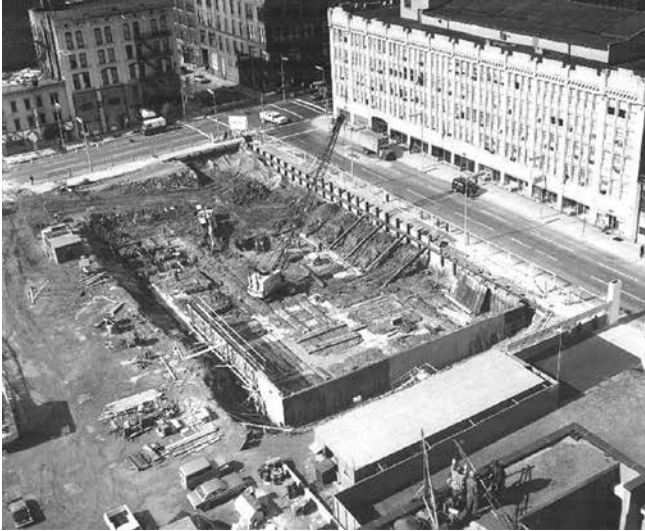
Figure 1: Construction begins on Fiberglass Tower and Plaza, Toledo, Ohio
