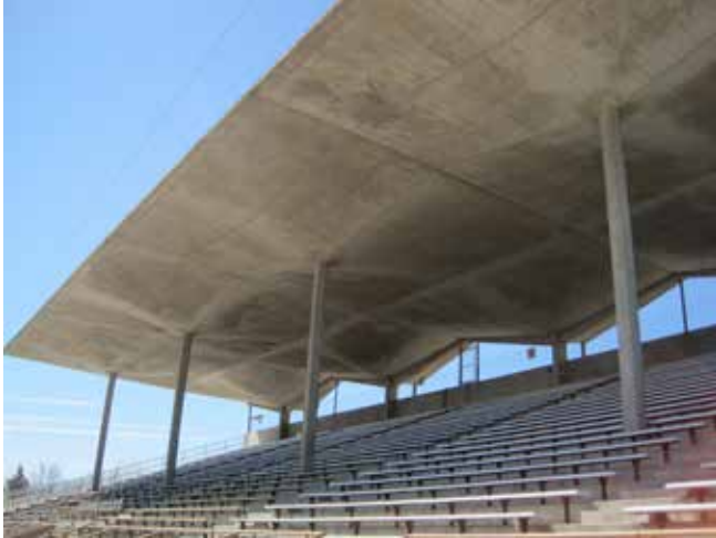
Figure 7: Grant County Fairground Grandstand, Underside of Shell. Photo by the author, 2014
