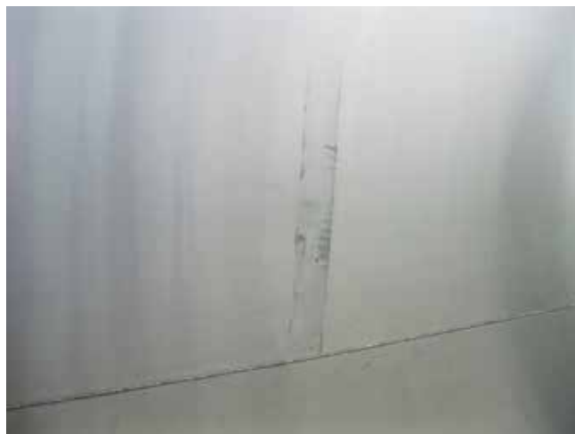
Figure 3. Vertical blemish within panel section (west face) shown within the dashed line
