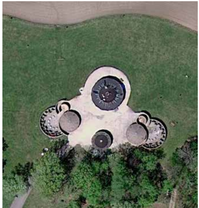
Figure 9: Aerial view of Lower Trout Lake Bath House Complex, Lake Orion, Michigan. The complex consists of two circular bath houses with open air changing areas and showers and enclosed toilets. A large concession building is closest to the water and there is a small pump house, now unused. A contact station is located close to the park entrance
