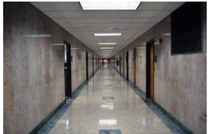
Figure 7: Interior view of the Hull building showing size of hallways
