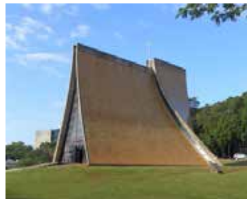
Figures 15: Exterior of Luce Chapel, 1963
