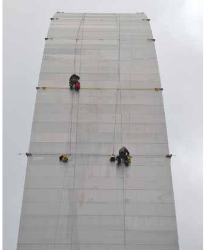
Figure 1: View of custom IRA system
