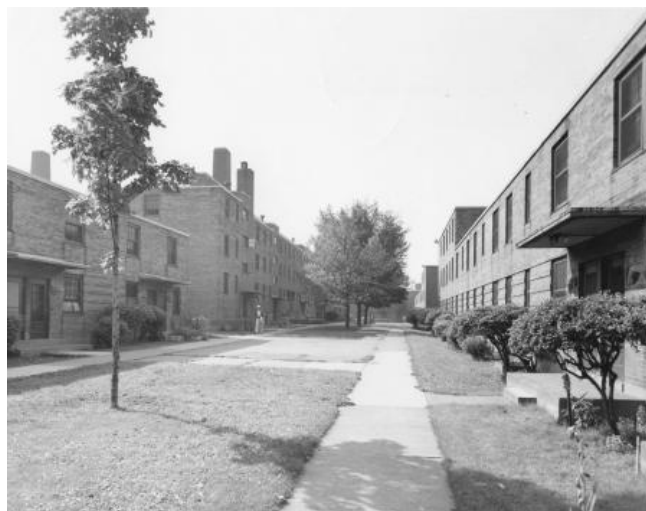
Figure 7: Willert Park Courts, outdoor spaces. Source: Buffalo Municipal Housing Authority, Center for Urban Planning, SUNY at Buffalo, date unknown
