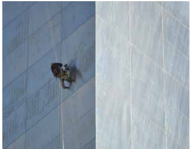
Figure 2: Overall view of the access at the intrados
