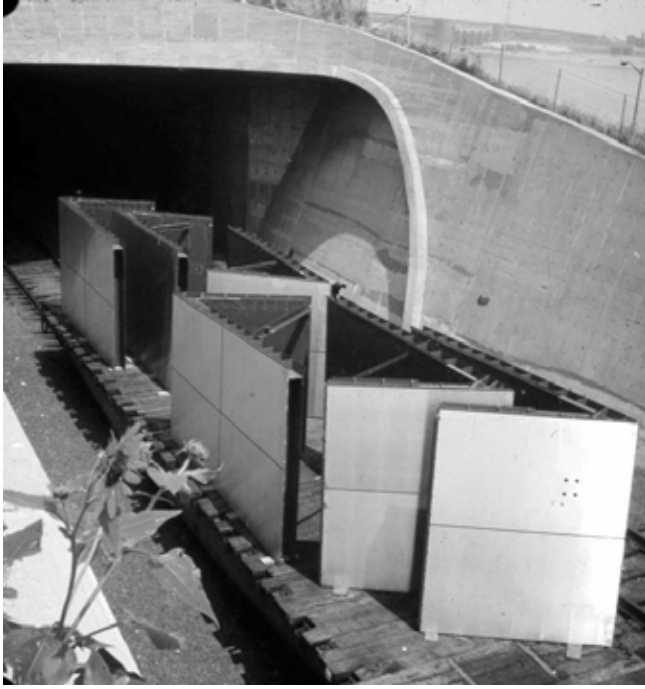
Figure 5: Arch station L-shaped sections transported by railcar to the job site, JEFF archives, image VREF-08677
