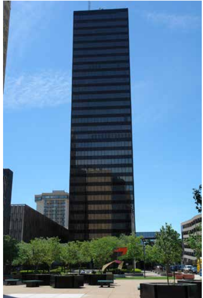
Figure 3: Construction begins on Fiberglass Tower and Levis Square in 2012, Toledo, Ohio. QEA, 2012
