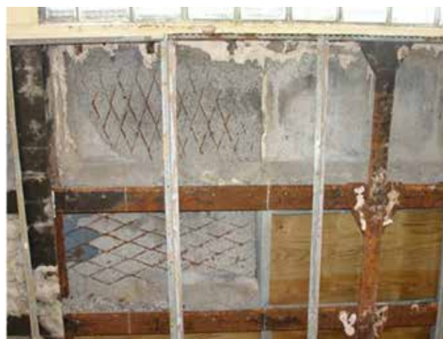
Figure 7: back side of concrete panels as viewed from the interior
