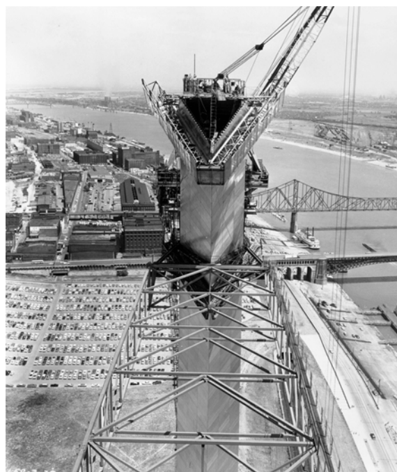
Figure 11: View of the stabilizing strut installed during construction to resist overturning and deflection of the cantilevered Arch legs, JEFF archives, image V106-4119
