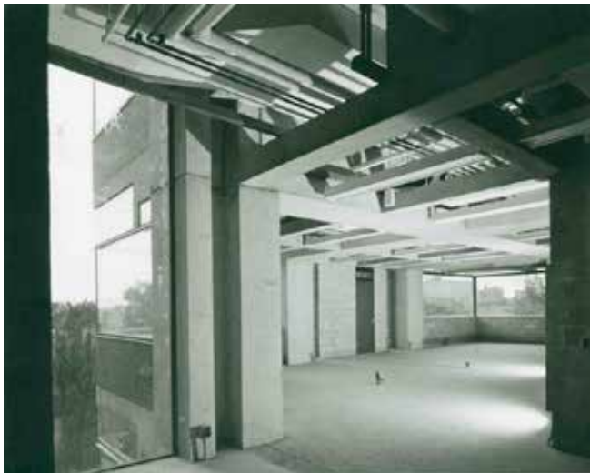
Figure 5: View from connector across typical lab floor before construction of partitions © 1961 (Penn Architectural Archives)
