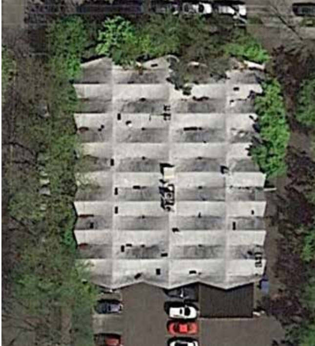
Figure 1: Shannon & Wilson Office Building, Aerial View Map data ©2015 Google Imagery ©2015 , DigitalGlobe, U.S. Geological Survey
