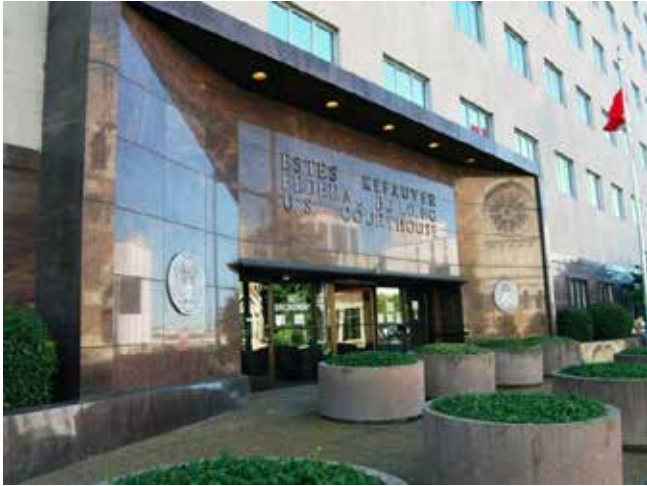
Figure 3: Entrance to the Kefauver Building
