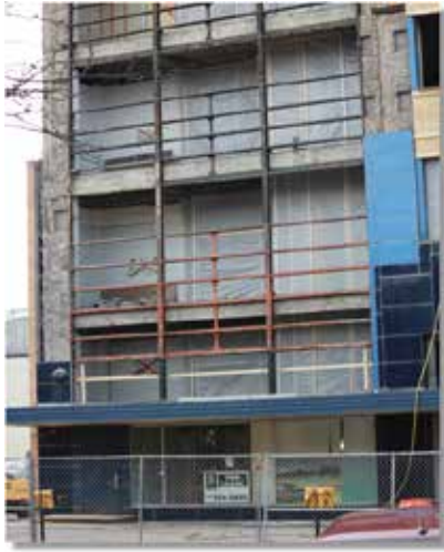
Figure 2: existing steel girt framing system
