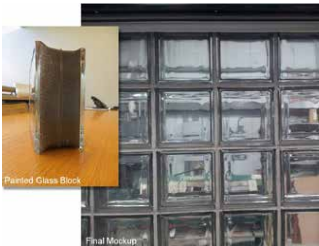
Figure 12: mockup of glass block with custom paint edging
