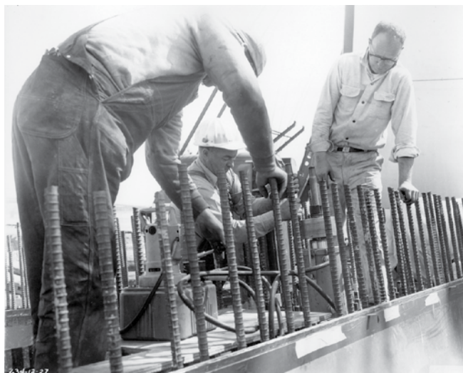
Figure 7: Applying tensile stress to the post-tensioning bars, 1963, JEFF archives, image V106-3974
