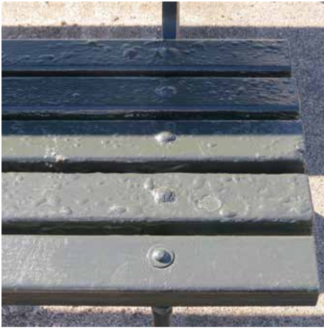
Figure 3: Replaced slat with washer under bolt due to enlarged bolt hole. Photograph by author
