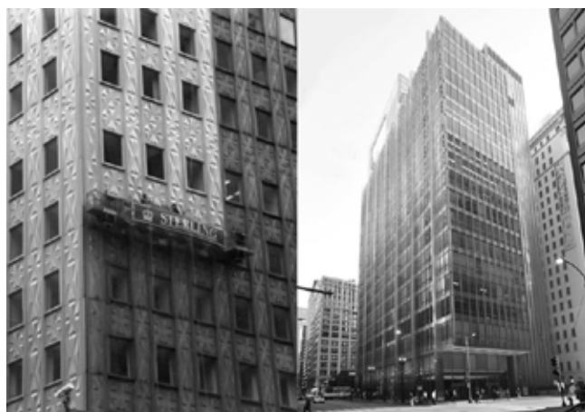
Figures 4 and 5: The Socony-Mobil building in New York, undergoing cleaning in 1995 (left); the Inland Steel Building in Chicago (right).
