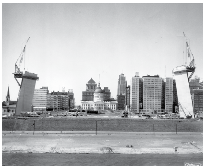
Figure 8: The Arch legs under construction with the creeper cranes in place, late summer 1963, JEFF archives, image V106-4034
