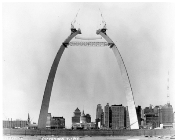
Figure 10: The Arch nears completion with the stabilizing strut in place, September 9, 1965, JEFF archives, image V106-4124
