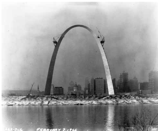
Figure 13: Cleaning the Arch and removing the creeper cranes, February 7, 1966, JEFF archives, image V106-4147
