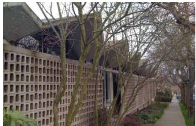
Figure 2: Shannon & Wilson Office Building, Exterior. Photo by the author, 2014
