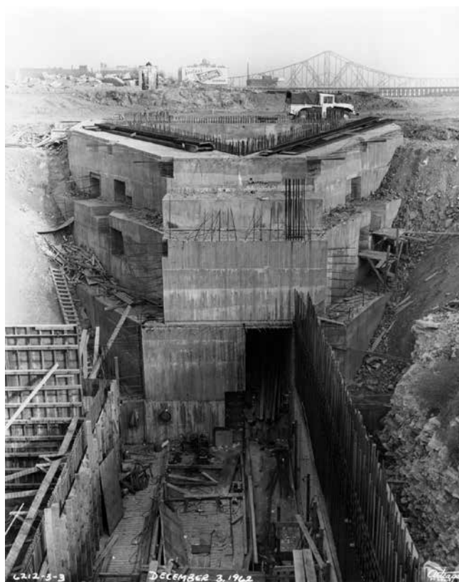
Figure 4: The north leg foundation nears completion, December 3, 1962, JEFF archives, image V106-3938
