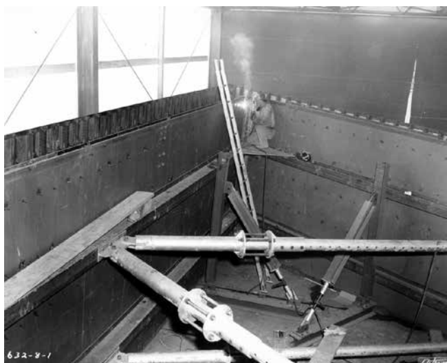
Figure 3: Shop assembly of the Arch stations, showing internal temporary framing for placement and installation, JEFF Archives, image V106-35946
