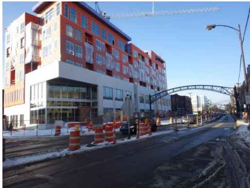
Windows and roof heights are at different levels than surrounding buildings.
