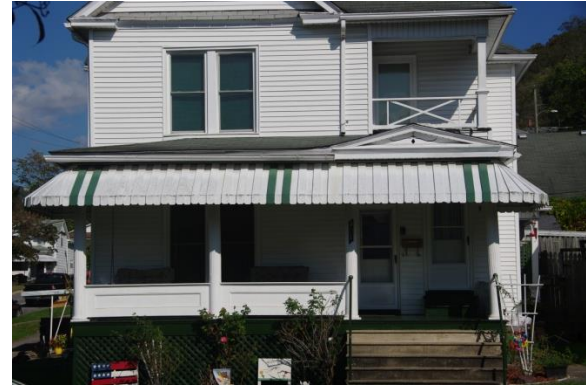
Residential building with one-story porch and inset balcony.
