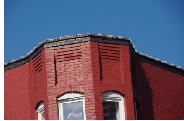
Brick Corbeling and Coping
