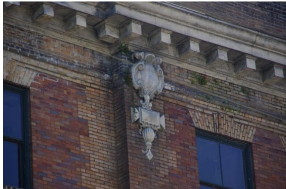
Jack Arch Lintel, Cartouche, and Modillion Cornice
