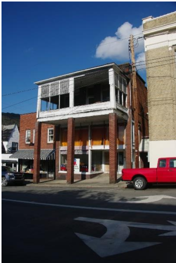
Raised porch on commercial building
