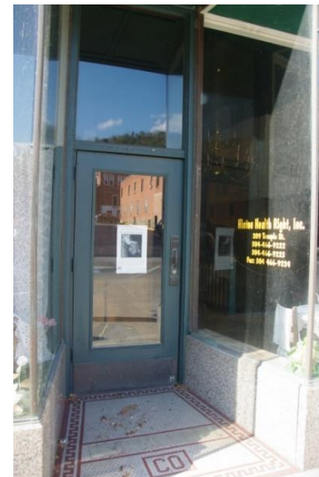
Commercial Door with Large Transom
