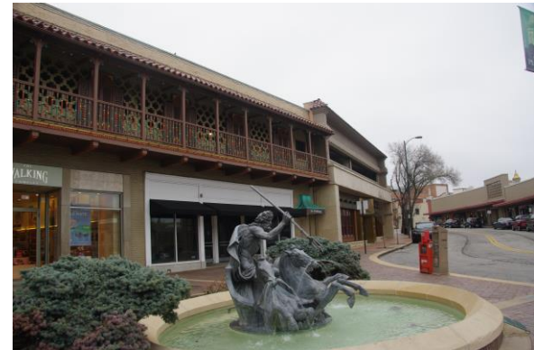
Even Parking Garage Openings Align with Porches and Windows.
