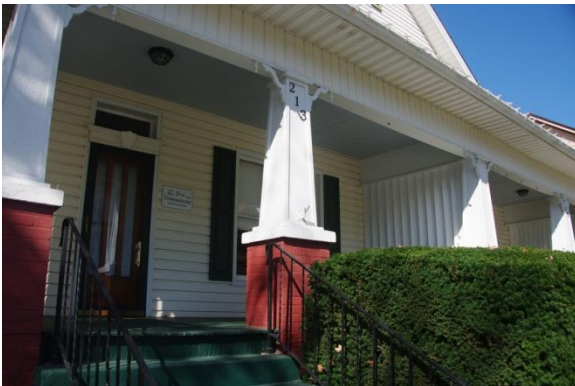
Battered Columns on Piers
