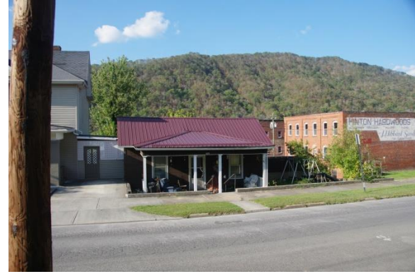
Example of inappropriate infill in the Hinton Historic District. The house's massing and materials are not compatible with the streetscape.
