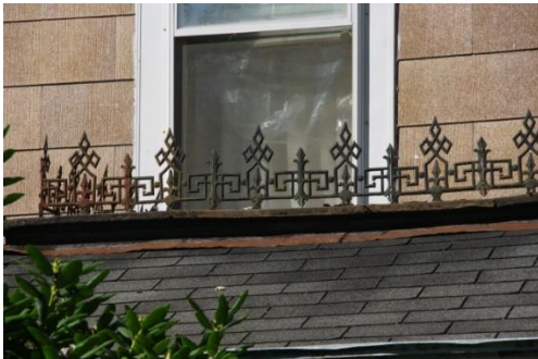
Iron Cresting On Roof
