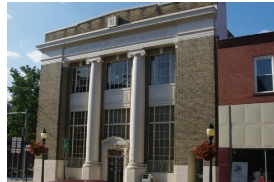
Ionic Columns and Plinths at Base
