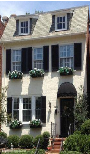
Appropriate Location and Size of Boxes
