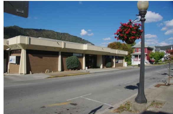
Example of inappropriate modern infill in the Hinton Historic District. The building's massing is not compatible with the streetscape
