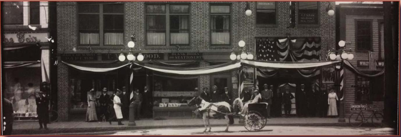
Historic storefronts in the Rochester Historic District.
