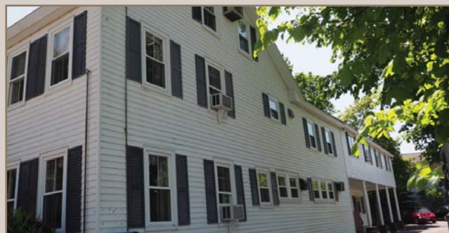
Simple painted wood siding for the rear addition is appropriate.
