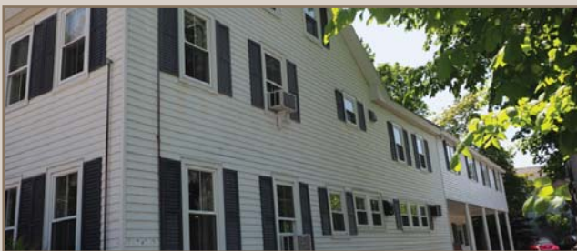
The second story cantilever distinguishes new from old construction.
