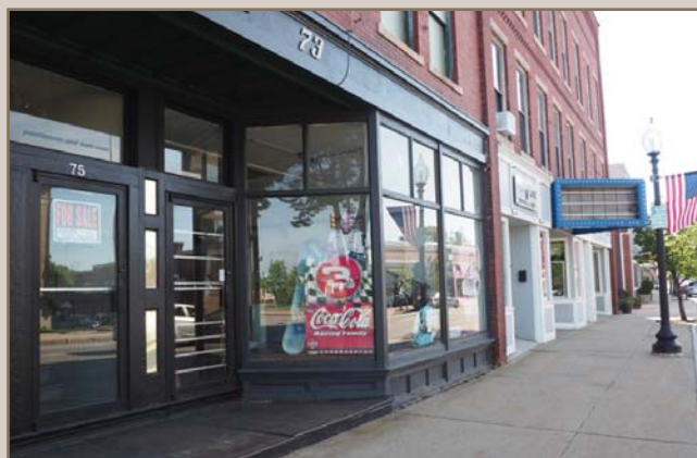
Historic storefronts with recessed commercial entries.
