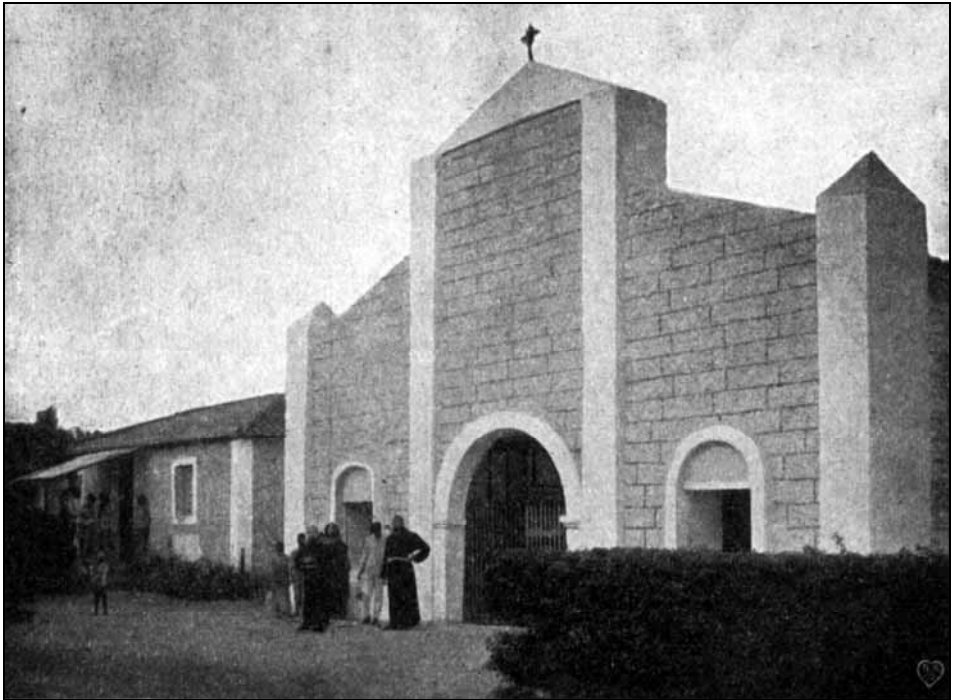
Figure 17. The front facade of the church after the heightening of the roof. 60
