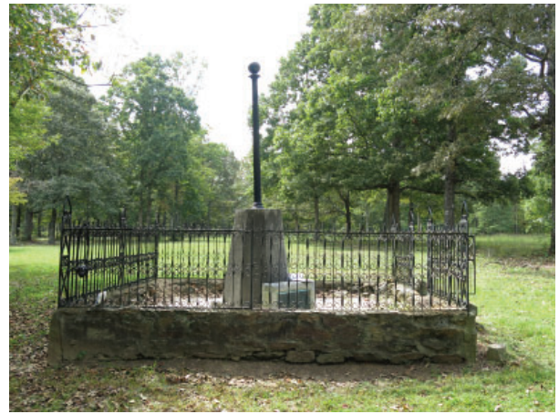
Figure 74: North elevation of enclosure, facing south-southeast, 25 September 2017.
