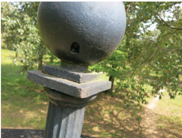
Figure 73: Detail of cast iron column capital and mounting of cast iron ball, 25 September 2017.
