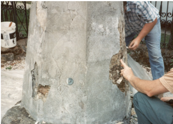
Figure 50. Photograph of the Washington Light Infantry Monument during removal of 1979-1980 plaster finish, facing north, 1993. Source: Cowpens National Battlefield Archives.
