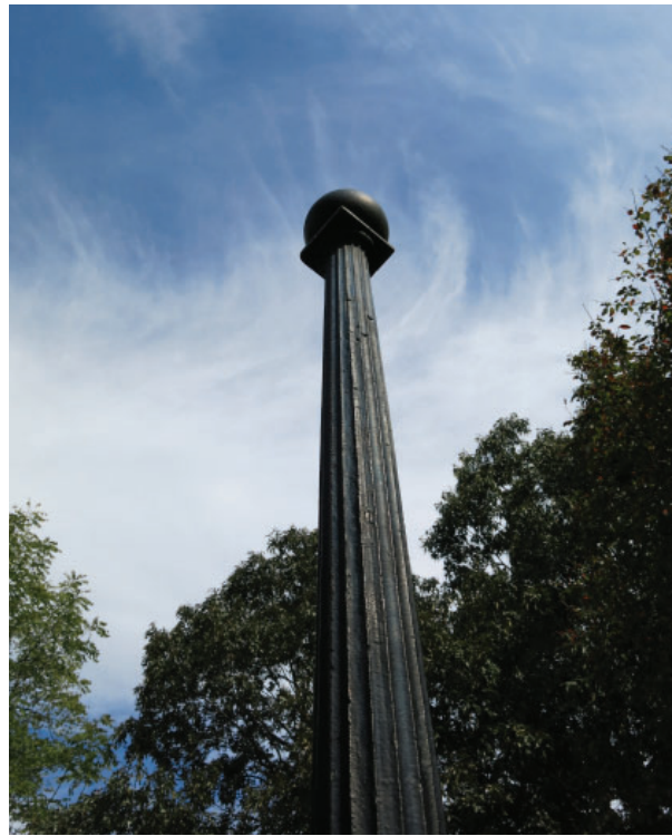
Figure 70: View of cast iron column shaft, 25 September 2017.
