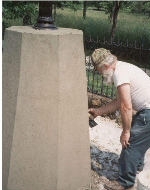
Figure 52. Photograph of the Washington Light Infantry Monument during installation of new stucco, facing north, 1993. Source: Cowpens National Battlefield Archives.
