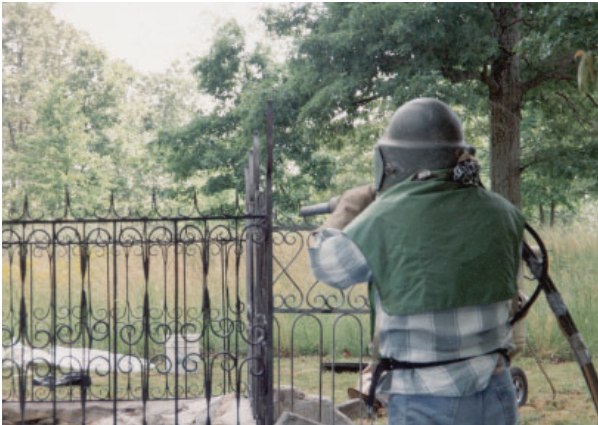
Figure 54. Photograph of the Washington Light Infantry Monument during abrasive blasting of iron fence, facing north-northeast, 1993. Source: Cowpens National Battlefield Archives.
