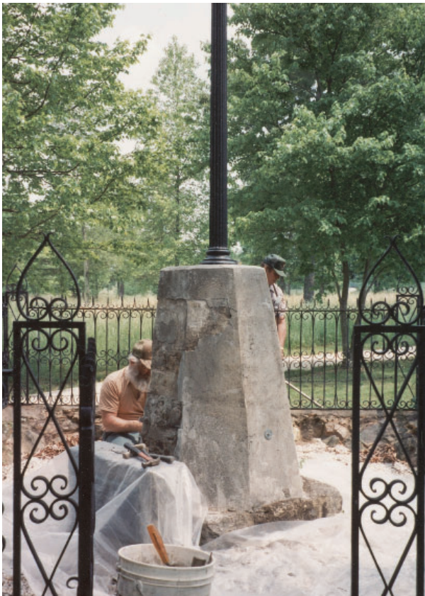
Figure 49. Photograph of the Washington Light Infantry Monument during removal of 1979-1980 plaster finish, facing east-southeast, 1993. Source: Cowpens National Battlefield Archives.
