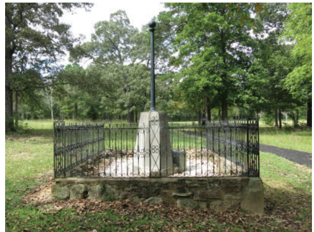
Figure 75: East elevation of enclosure, facing west-northwest, 25 September 2017.
