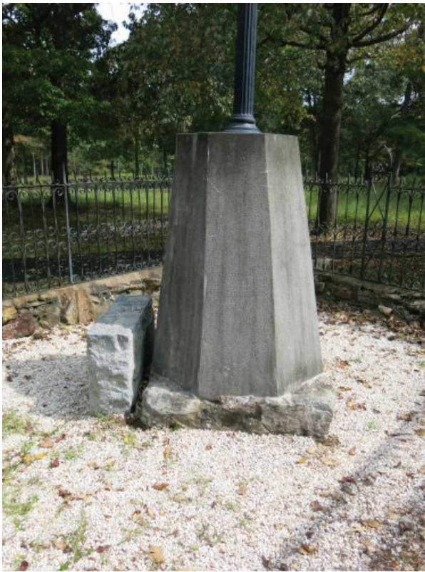
Figure 66: Southwest elevation of monument, facing northeast, 25 September 2017.
