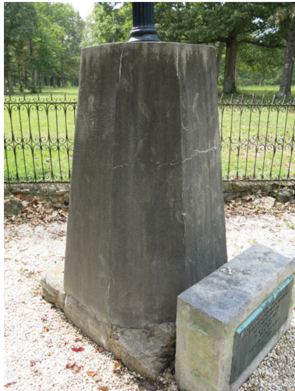
Figure 64. North elevation of monument, facing south, 25 September 2017.
