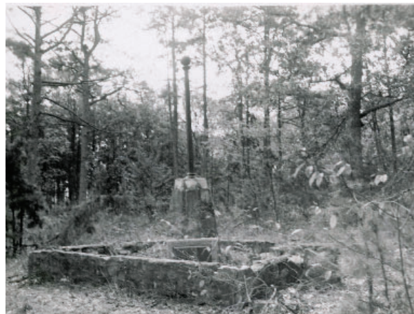
Figure 38. Photograph of the Washington Light Infantry Monument, facing south-southeast, 1975. Note the removal of the iron fence and marble cap as well as the general appearance of deterioration. Source: Kings Mountain National Military Park Archives, Box 3B, c 93.
