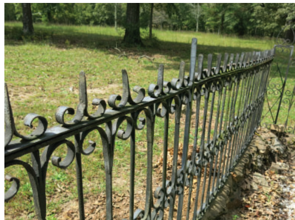
Figure 80: Detail of typical conditions at iron fence, 25 September 2017.
