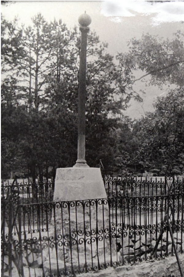
Figure 27. Photograph of the Washington Light Infantry Monument, facing northeast, c.1932-1936. This photograph appears to have been taken during or immediately following the 1930s repair campaign; note the apparent stucco residue on the lower part of the cast iron column. Source: Washington Light Infantry archives.
