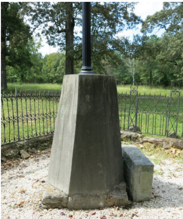
Figure 63. Northeast elevation (historic front) of monument, facing southwest, 25 September 2017.
