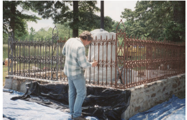
Figure 56. Photograph of the Washington Light Infantry Monument during priming of iron fence, facing northwest, 1993. Source: Cowpens National Battlefield Archives.
