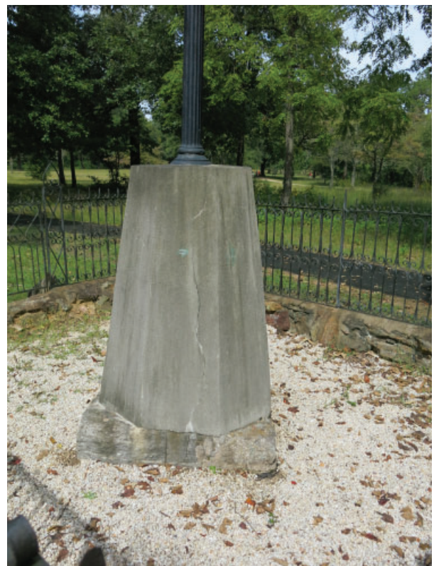
Figure 68: Southeast elevation of monument, facing northwest, 25 September 2017.
