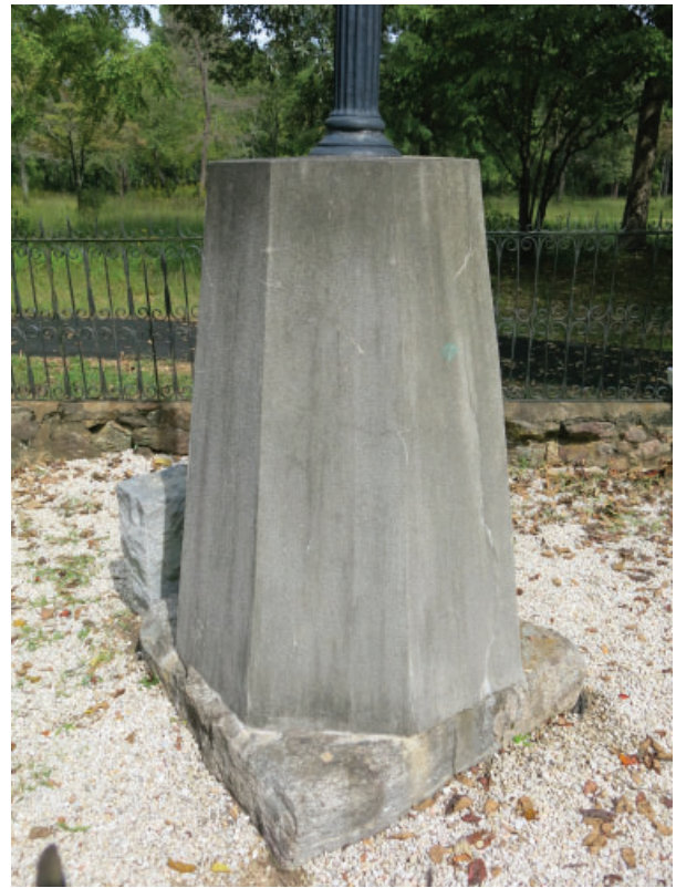
Figure 67: South elevation of monument, facing north, 25 September 2017.
