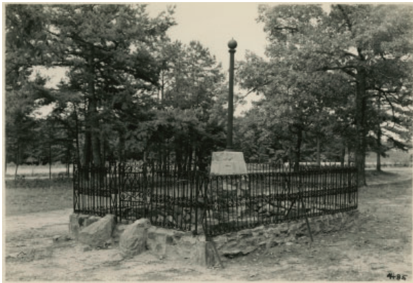
Figure 28. Photograph of the Washington Light Infantry Monument, facing northeast, 1936. Green River Road is visible beyond the trees while the dirt cutoff road is just beyond the fenced enclosure. Note the stucco patches, new marble cap, and new ball on the monument and the damaged condition of the iron fence atop the new stone wall. Source: Kings Mountain National Military Park Archives, Box 3A, 136-4485.
