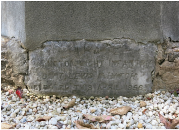
Figure 61. Marble plaque on northeast elevation (historic front) of monument base, facing southwest, 25 September 2017.
