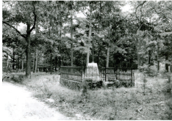
Figure 37. Photograph of the Washington Light Infantry Monument, facing southeast, 1972. The dirt cutoff road is visible at left. Source: Kings Mountain National Military Park Archives, Box 3B, c 234, no. 12 of 37.
