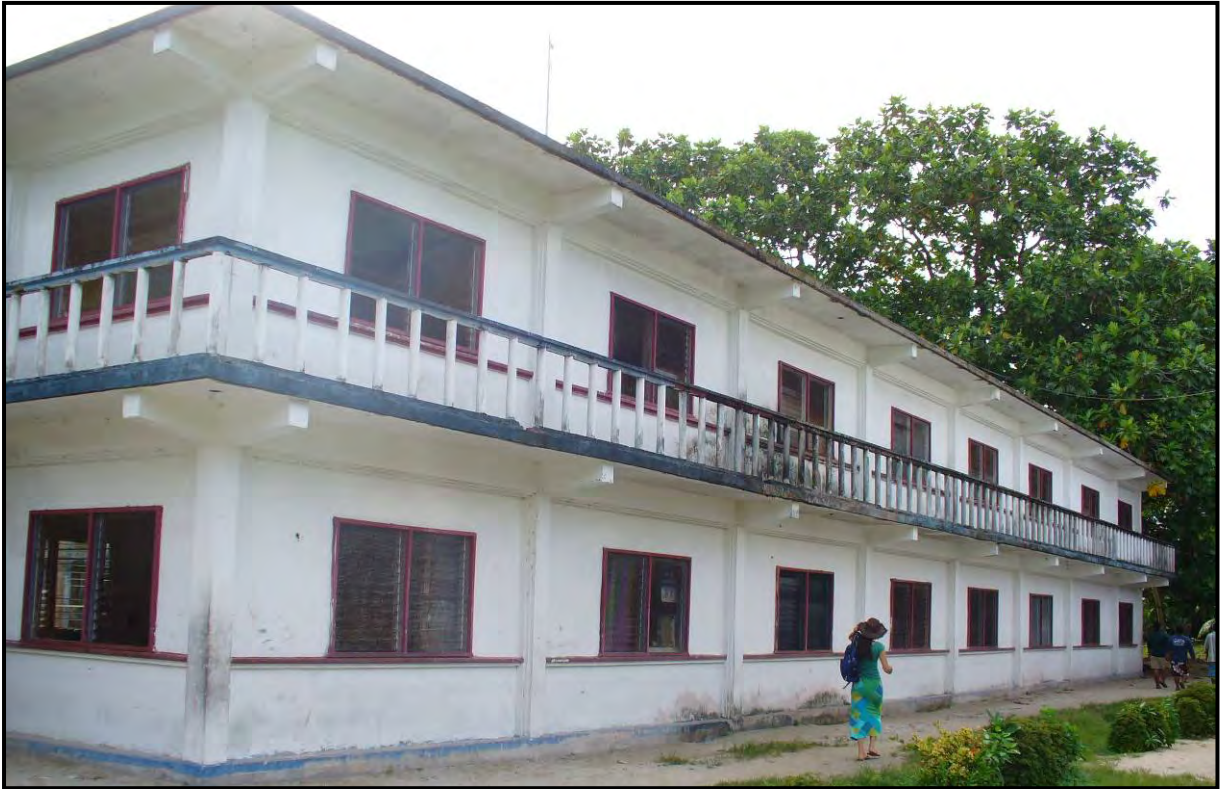
Fig 17: The school building on Moch
