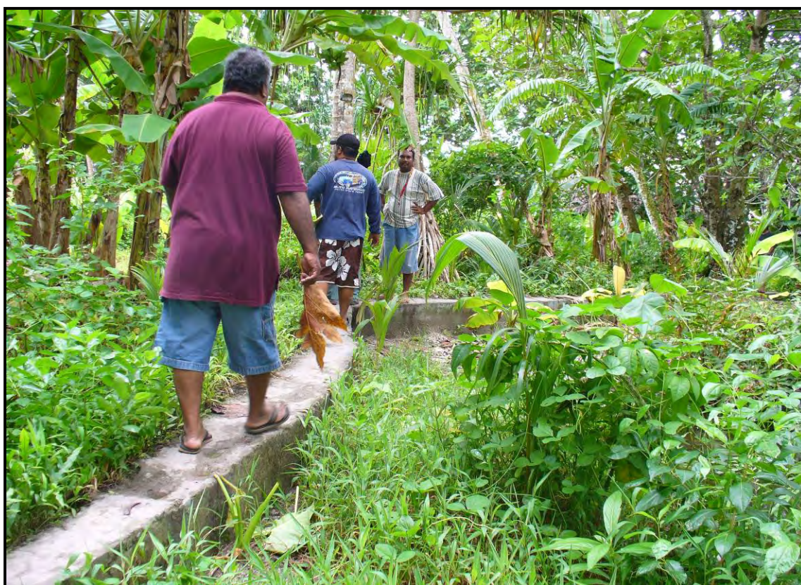
Fig 15: Concrete wall protecting the central taro patch from saltwater inundation
