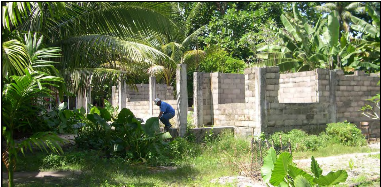
Fig 18: Concrete house construction
