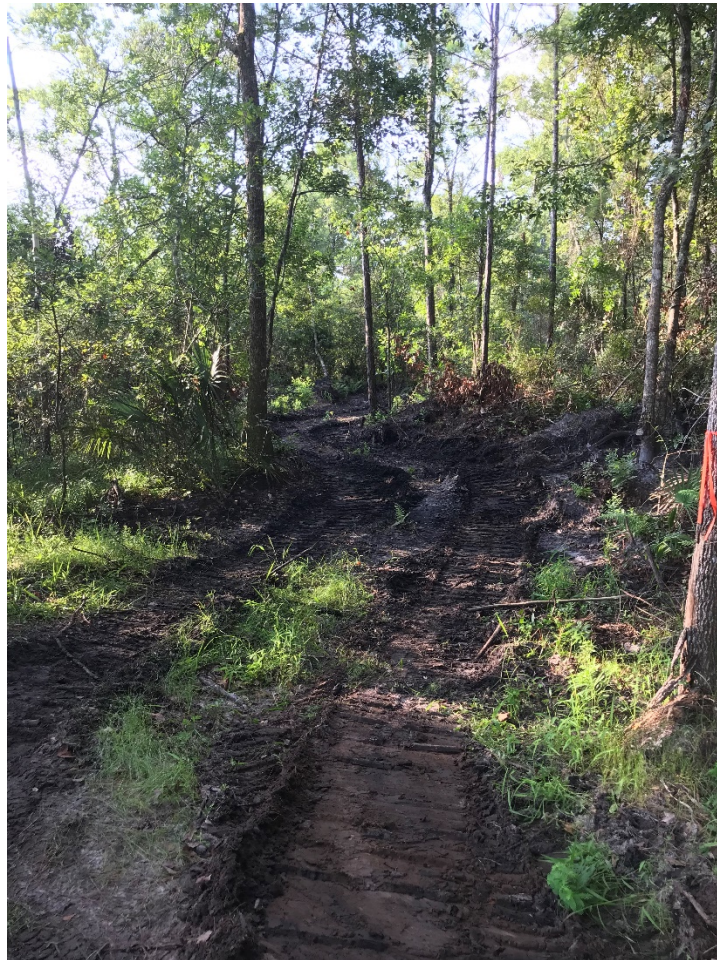
Photograph 1: Dozer Line near the billboard; before
