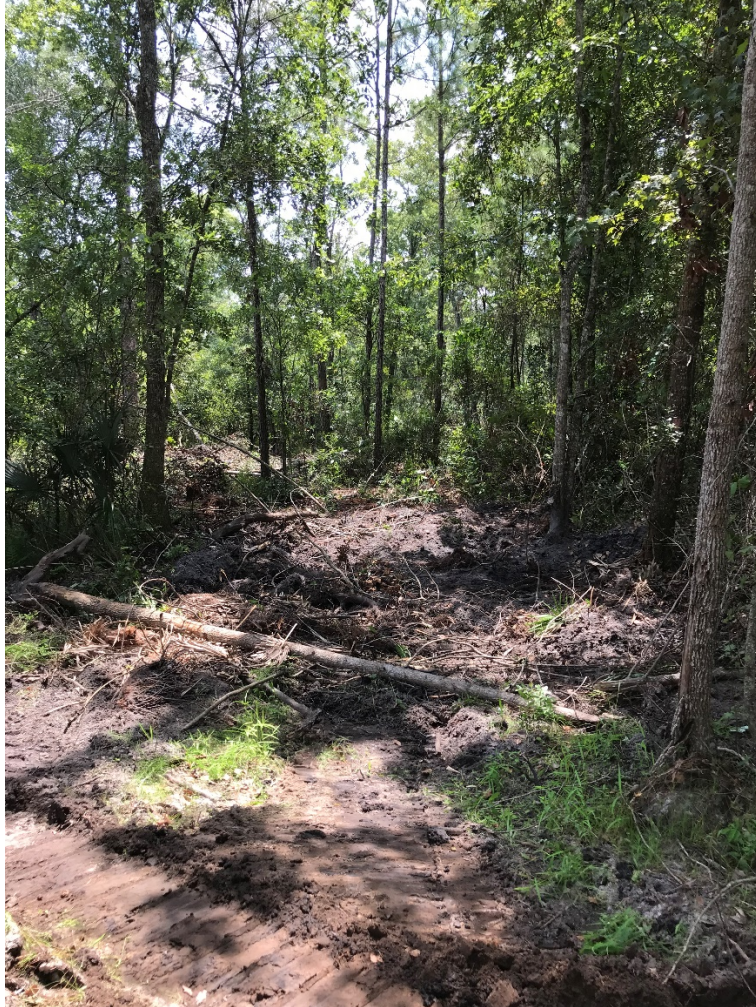
Photograph 2: Repair/Rehab to Dozer Line; After
