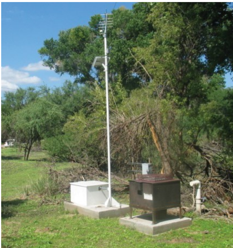
Groundwater monitoring wells at Tumacácori National Historical Park.
