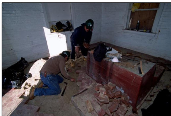
Figure 68. A concrete and brick pedestal was still extant in the building prior to its move. Photo: Cape Hatteras National Seashore Archives, 01/19/99.
