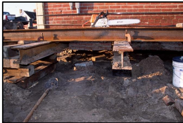
Figure 28. Wood cribbing supports the main beams, which support the needle beams, which support the oil house. Photo: Cape Hatteras National Seashore Archives, 03/04/99.
