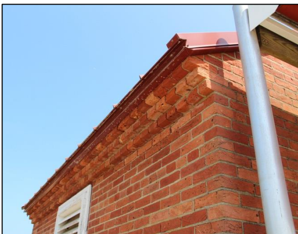
Figure 76. The projecting brick stepped cornice is original and character defining. Photo: HPTC, 05/12/16.
