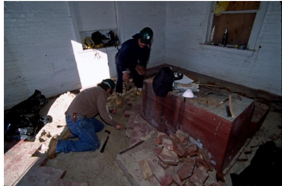
Figure 26. The concrete foundation located in the center of the Oil House was the base for a generator used by the USCG. Cape Hatteras National Seashore Archives, 01/19/99.
