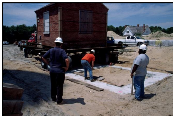
Figure 30, above. Locating the Oil House above the reinforced concrete footing. Photo: Cape Hatteras National Seashore Archives, 08/05/99.
