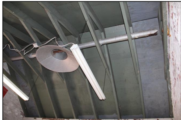
Figure 83. The roof framing is exposed on the interior of the building. Photo: HPTC, 05/11/16.
