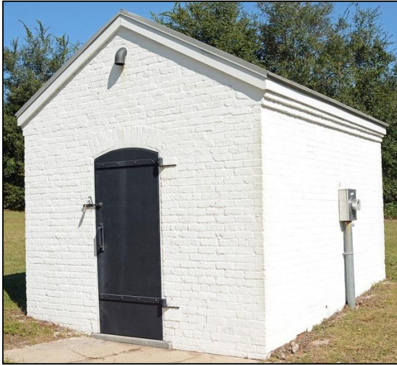
Figure 64. The restored 1890 Amelia Island Oil House with exterior door, strap hinges, and pintels. Photo: https://en.wikipedia.org/wiki/Amelia_Island_Light . Accessed 06/29/16. Cropped by author.
