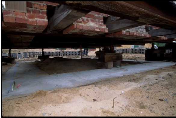
Figure 31. Lowering the Oil House to a precise height. Photo: Cape Hatteras National Seashore Archives, 08/19/99.
