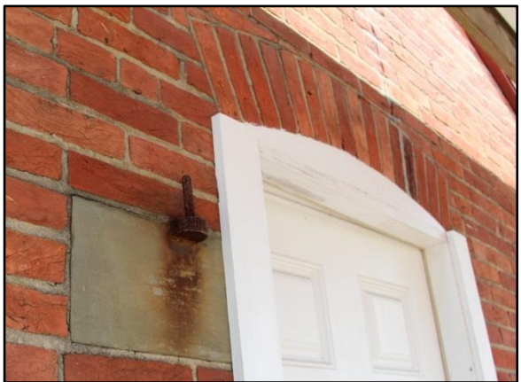
Figure 54. A brick jack arch located at the exterior door entrance. Note also the slate embedded into the wall which holds a historic pintel for the original door. Photo: HPTC, 05/12/16.
