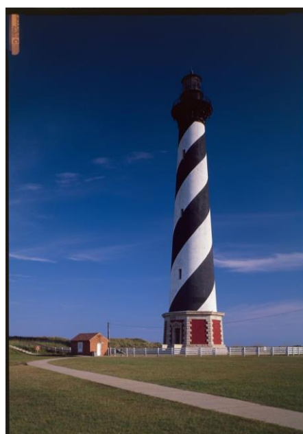
Figure 17. The exterior of the oil house in 1989. Photo: HABS, https://www.loc.gov/item/nc0432/ .
