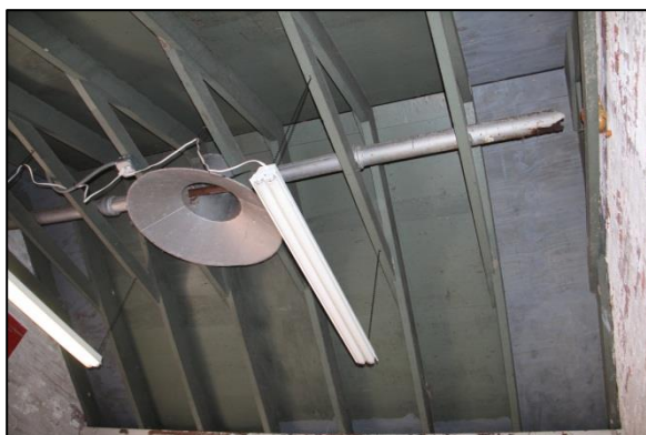
Figure 67. Metal components leftover from the Oil House's use as an auxiliary power generator. Photo: HPTC, 05/12/16.
