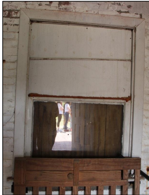
Figure 60. The interior of W102. Photo: HPTC, 05/12/16.
