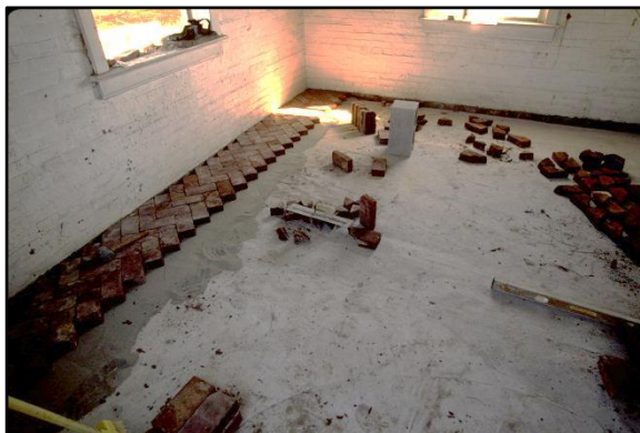
Figure 49. The new concrete slab poured atop fill and supporting the brick finish floor. Photo: Cape Hatteras National Seashore Archives, 10/02/99.
