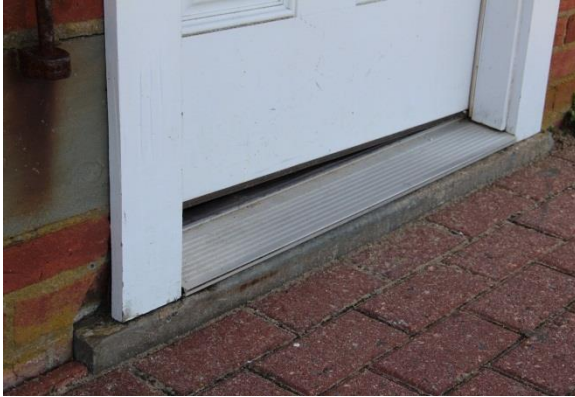
Figure 55. The slate door threshold is covered with a modern metal threshold. Note the slate block embedded in the exterior wall and metal pintel. Photo: HPTC, 05/12/16.
