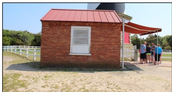
Figure 74, right. Neutral drainage around the Oil House. Photo: HPTC, 05/12/16.
