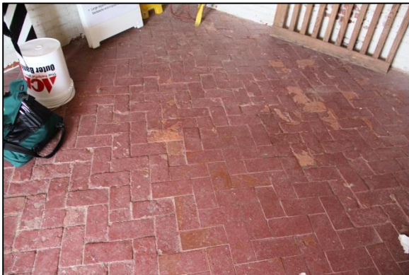
Figure 82. Character-defining brick floors were re-laid and patched after the building's move. Photo: HPTC, 05/12/16.
