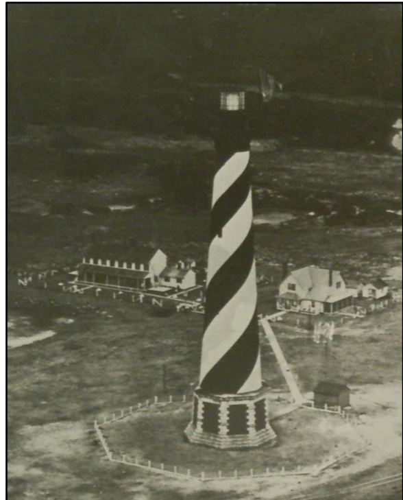
Figure 10. The south and east elevations of the oil house in 1932, from an Army Air Corps plane. No windows are yet located in the oil house. Photo: Hatteras National Seashore Archives. Cropped by author.
