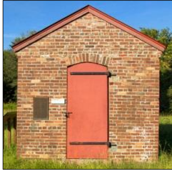
Figure 65. The restored 1890 Sapelo Island Oil House with exterior door, strap hinges, and pintels. Photo: https://vanishingcoastalgeorgia.com/2012/09/17/sapelo-island-lighthouse-1820-oil-house-1890/ . Accessed 06/29/16. Cropped by author.
