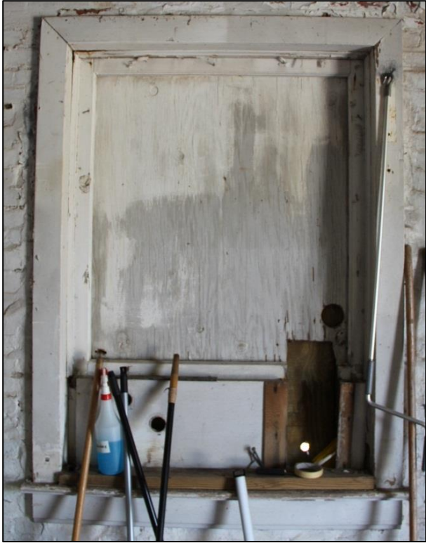
Figure 69. Simple interior wood trim at one of the windows. Photo: HPTC, 05/12/16.
