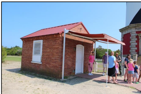
Figure 39. The Oil House from the northwest corner. The Lighthouse is located to the south. Photo: HPTC, 05/12/16.
