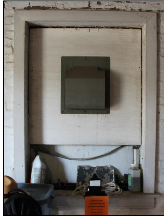
Figure 62. The interior of W103. Photo: HPTC, 05/12/16.
