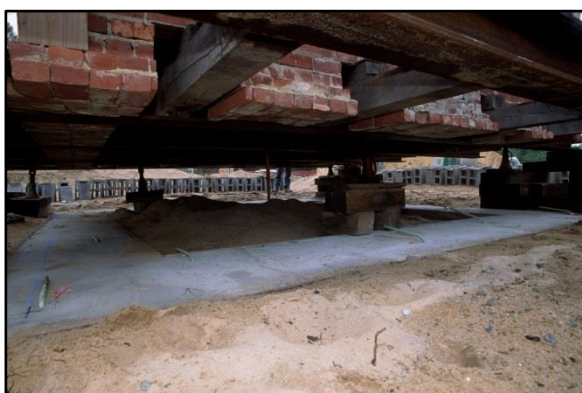
Figure 47. The Oil House positioned over the new continuous reinforced concrete footing. Concrete block is lined up in the background ready to be laid between the footing and the historic brick walls above. Photo: Cape Hatteras National Seashore Archives, 08/19/99.
