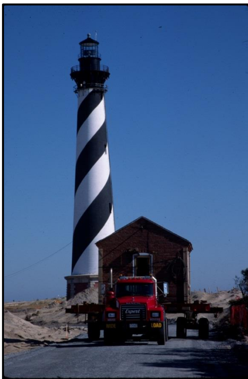
Figure 29, left. The Oil House travels to its temporary holding site, until the lighthouse can be moved. Photo: Cape Hatteras National Seashore Archives, 03/04/99.
