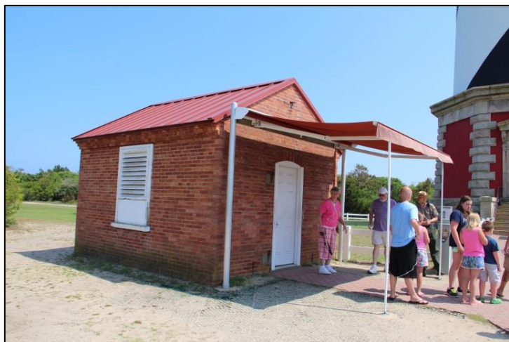
Figure 75. The Oil House retains its character-defining shape and mass. The modern awning, replacement door, and plywood window infill are not character-defining features. Photo: HPTC, 05/12/16.
