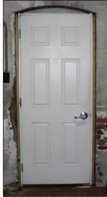
Figure 70. The new exterior door has not been trimmed out on the interior. Photo: HPTC, 05/12/16.
