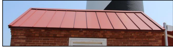
Figure 80. The projecting brick stepped cornice and standing-seam metal roof are character-defining features. Photo: HPTC, 05/12/16.
