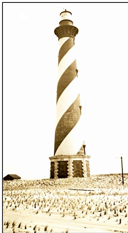
Figure 12. The Lighthouse and part of the Oil House, March 15-18, 1937. Photograph included as part of "A Field Investigation at Cape Hatteras Lighthouse" by Charles W. Porter, Assistant [illegible]. Photo: Cape Hatteras National Seashore Archives.
