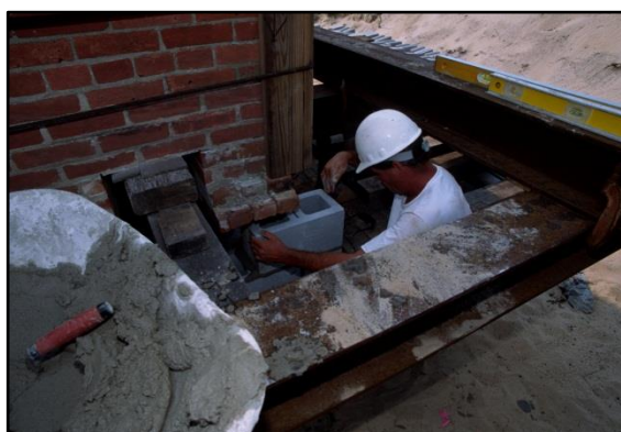
Figure 48. Concrete block being laid between the new concrete footing and the historic walls above. Photo: Cape Hatteras National Seashore Archives, 08/19/99.
