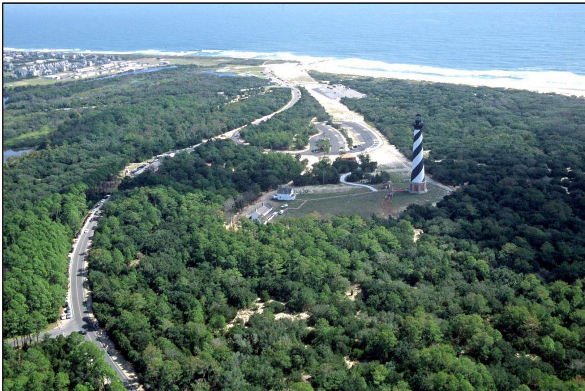
Figure 34. The light station about a year after the move project is complete. Photo: Cape Hatteras National Seashore Archives, 09/00.
