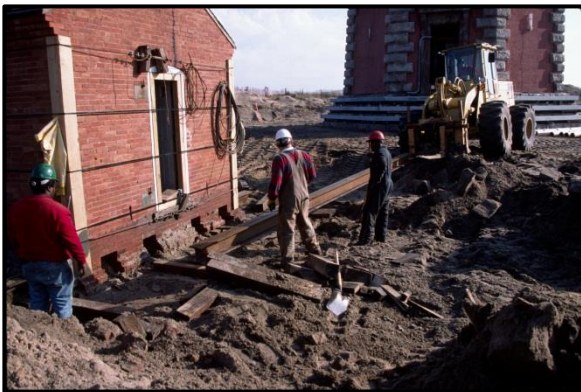
Figure 27. A steel needle beam is slid into place under the Oil House. Note the extra stabilization measures at the door opening, corners, and steel cables around the building. Photo: Cape Hatteras National Seashore Archives, 03/04/99.
