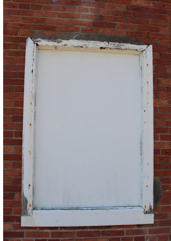
Figure 56, right. The ca. 1930s window openings have steel lintels covered with wood trim and wood sills. Photo: HPTC, 05/12/16.
