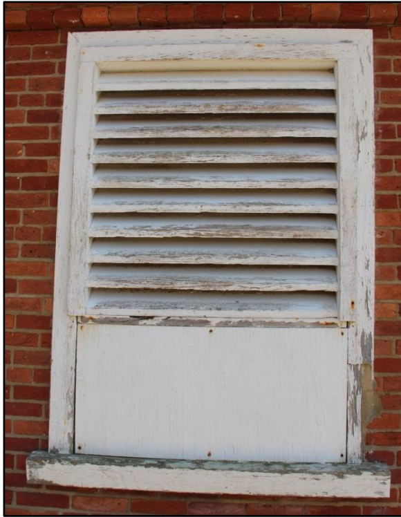
Figure 61. The exterior of W103. Photo: HPTC, 05/12/16.
