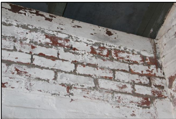
Figure 53. The interior faces of the exterior walls have been painted. Note the presence of Portland cement-based mortar. Photo: HPTC, 05/12/16.
