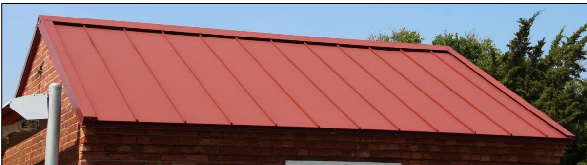
Figure 66. The standing-seam metal roof atop the Oil House was installed sometime since July 2005. Photo: HPTC, 05/12/16.
