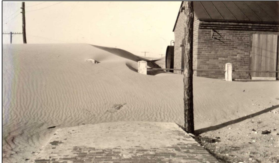
Figure 11, right. The condition of the Oil House in ca. 1934. Windows had been added by this time, but the original door and roof covering remained. Photo: Cape Hatteras National Seashore
