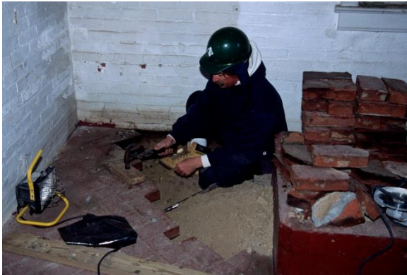
Figure 25. Systematic removal of the brick floor on the interior of the Oil House. Photo: Cape Hatteras National Seashore Archives, 01/19/99.
