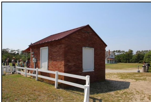
Figure 40. The Oil House from the southeast corner. Photo: HPTC, 05/12/16.
