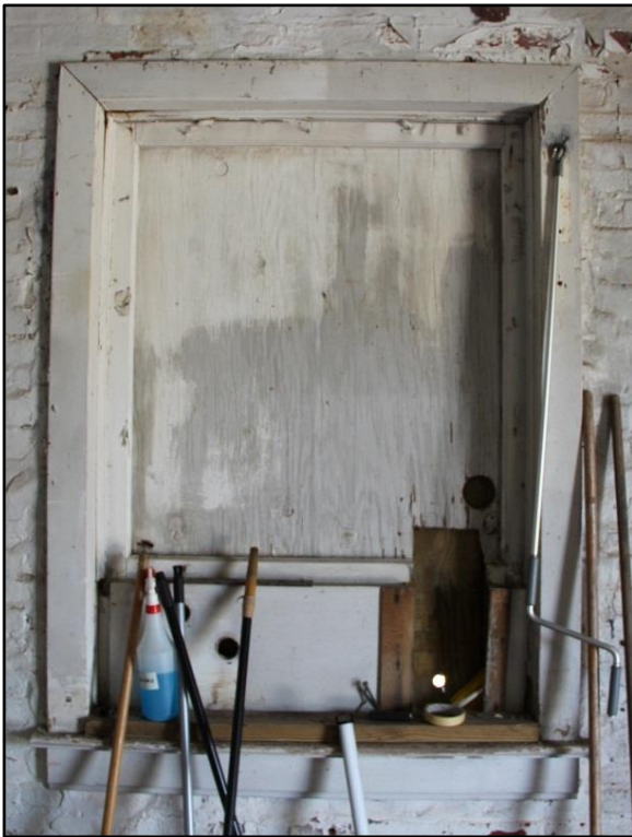
Figure 59 The interior of W101. Photo: HPTC, 05/12/16.
