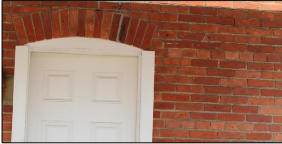
Figure 79. The brick arch over the door opening and common-bond brickwork are original and character defining. Photo: HPTC, 05/12/16.
