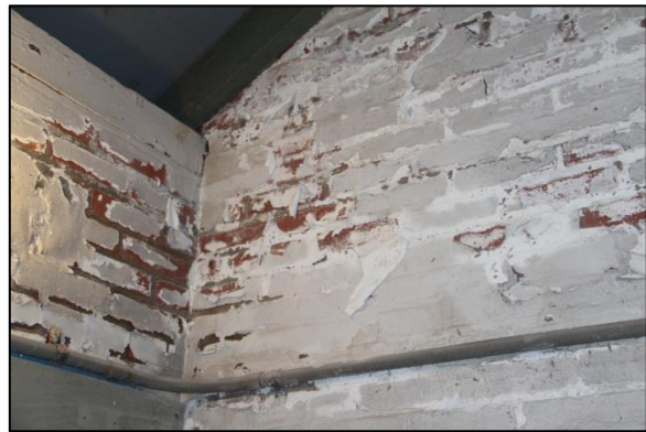
Figure 81. Painted brick walls seen on the interior of the building. Photo: HPTC, 05/12/16.
