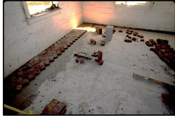
Figure 32. Relaying the historic brick over a new concrete slab and sand layer. Photo: Cape Hatteras National Seashore Archives, 10/02/99
