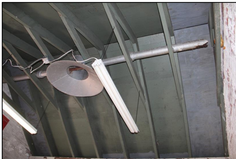
Figure 50, right. The ca. 1950 roof frame is exposed on the interior of the Oil House. Photo: HPTC, 05/12/16.
