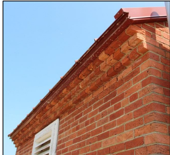
Figure 52, right. The brick cornice at the top of the exterior walls. Photo: HPTC, 05/12/16.
