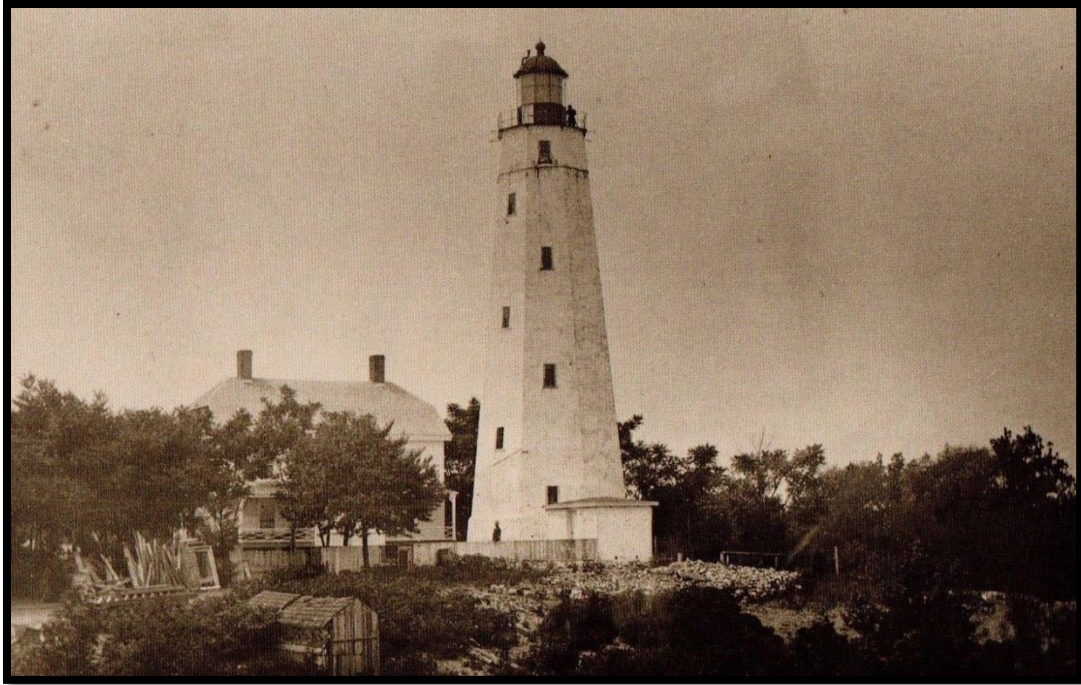
Figure 4.23: Sandy Hook lighthouse in an early-20th-century photograph, note the oil storage building to the east of the lighthouse. Courtesy of the National Park Service, Gateway National Recreation Area.
