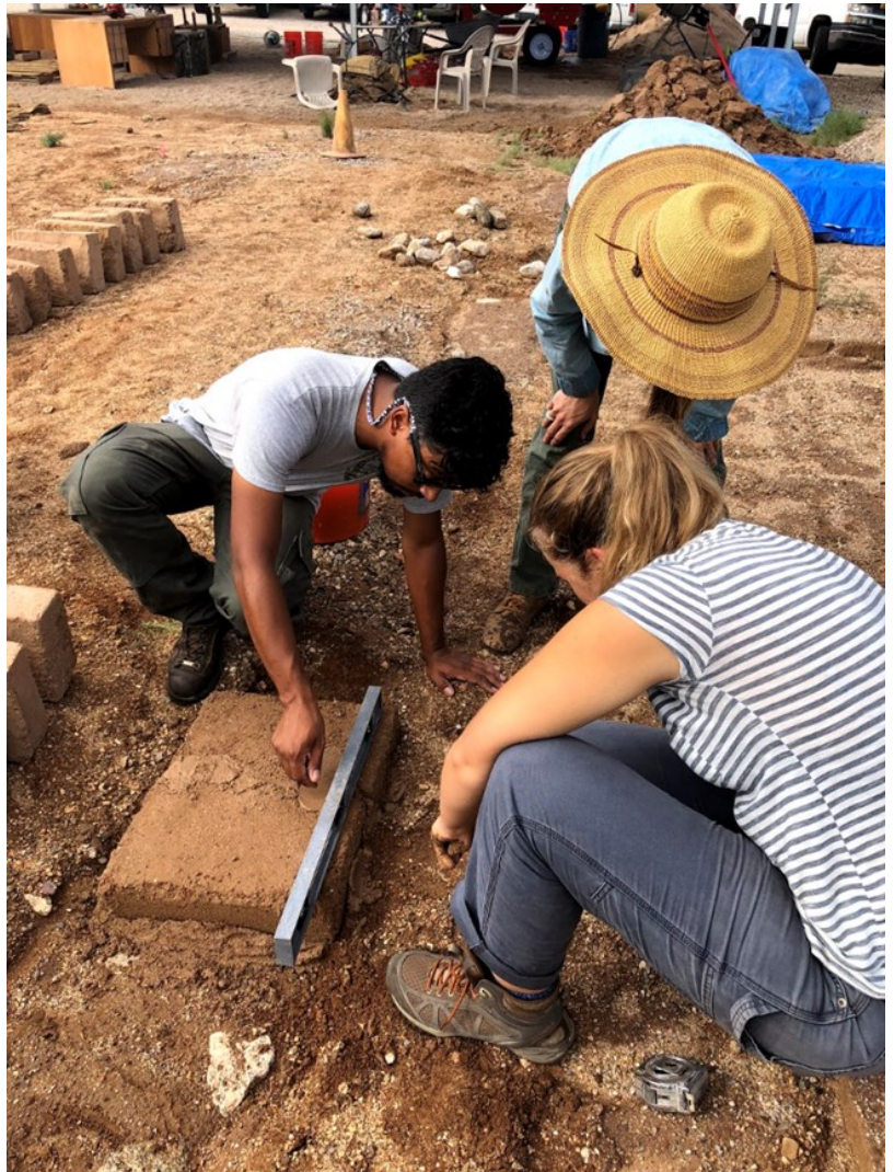
In the project's first phase, participants learned to make adobe bricks.
