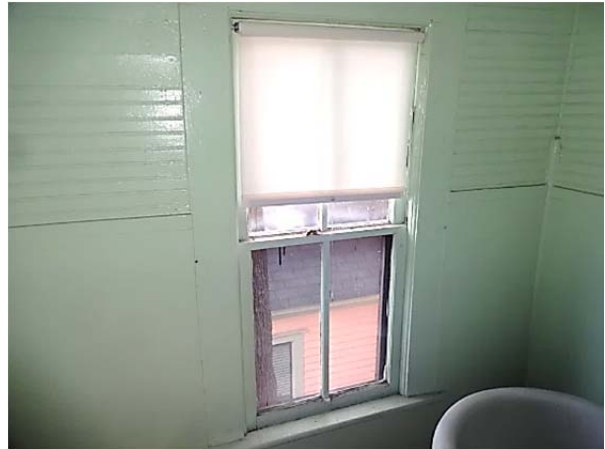
FIGURE 75. Overview of the bathroom window.
