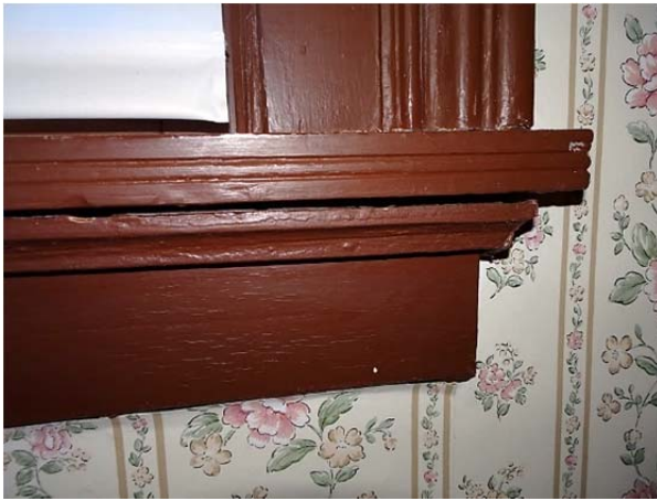
FIGURE 60. Typical wood stool and apron below window).
