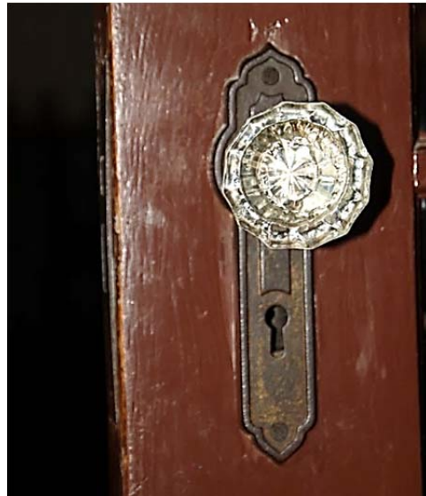
FIGURE 98. Mortised latch set with glass knob at French door.
