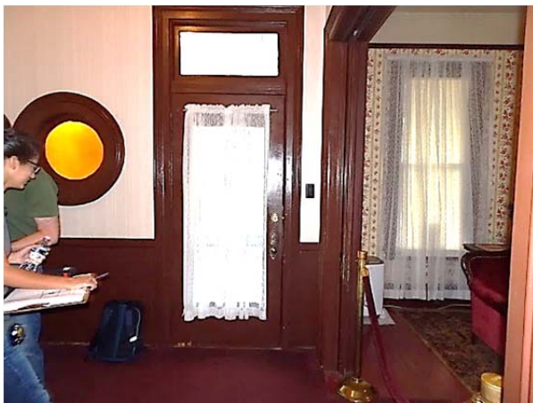
FIGURE 81. Overview of main entrance door.
