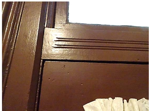
FIGURE 83. Detail of wood transom bar at main entrance door.
