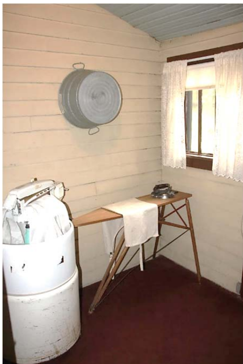
FIGURE 120. Clapboard siding inside the first-floor back porch.
