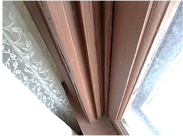
FIGURE 68. Window jamb with parting strips separating the jamb into pockets.
