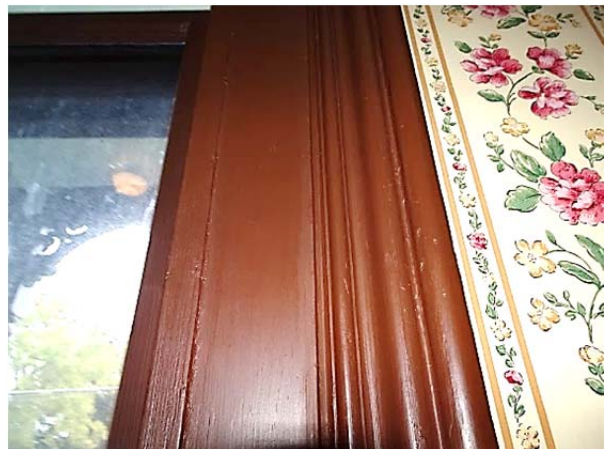
FIGURE 69. Casing with parting bead at first floor windows on the north elevation.
