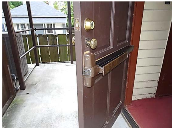
FIGURE 92. Hardware on second-floor rear exit door.
