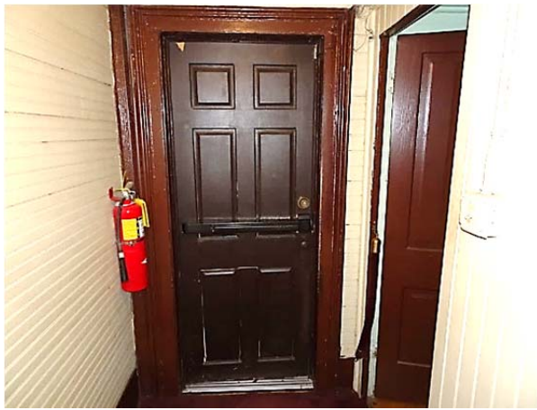
FIGURE 93. Hardware at second-floor exit at south elevation.
