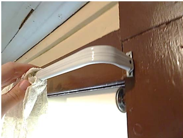
FIGURE 67. Curtain rod anchored to wood trim.
