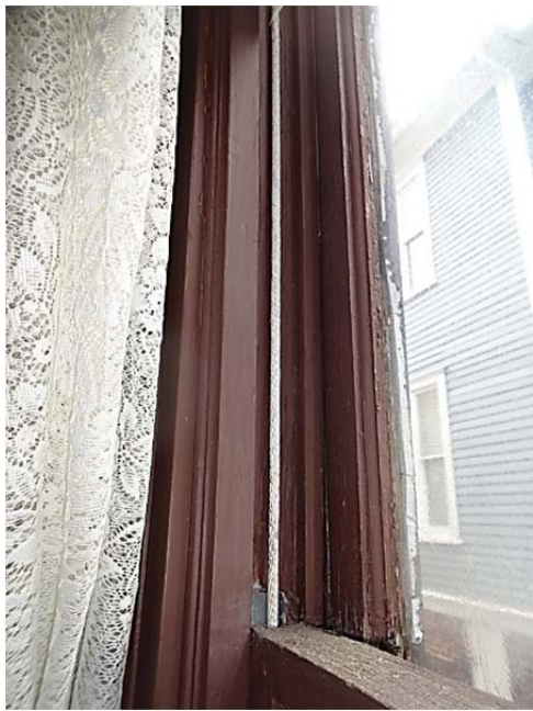
FIGURE 74. Typical two-over-two window opening jamb.
