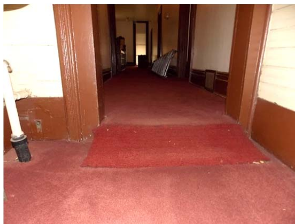
FIGURE 154. Carpeted ramp at upstairs rear porch.
