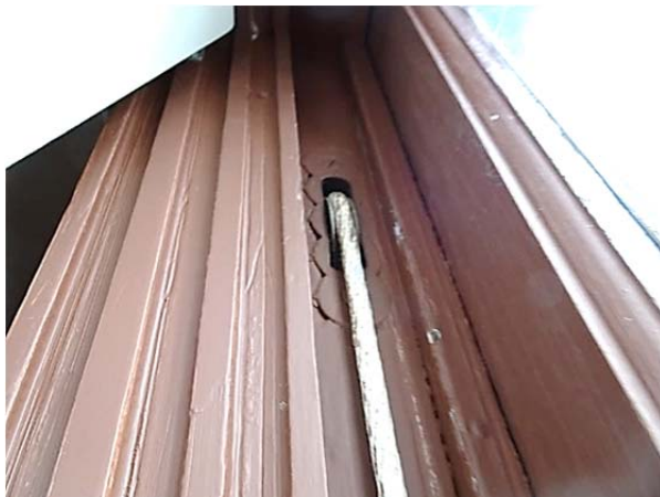
FIGURE 72. Window jamb at the second-floor north elevation. Note the addition grooved trim piece.
