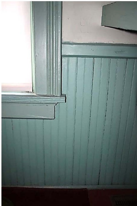
FIGURE 115. Double-beaded wainscot and chair rail in the kitchen.
