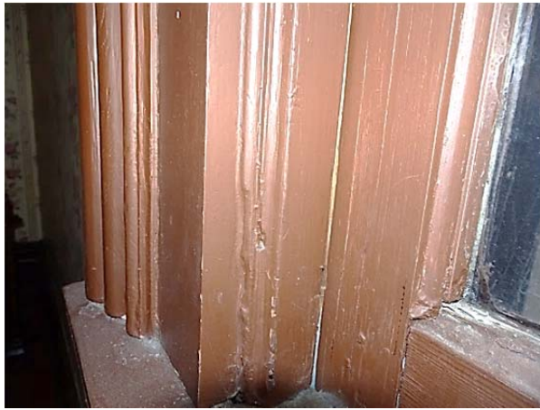
FIGURE 70. Window casing and jamb with bead molding sash stop.
