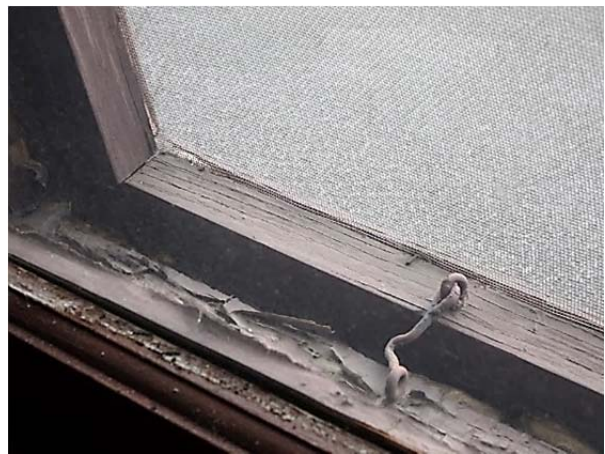
FIGURE 176. View from the interior looking at the exterior portion of the window sash.
