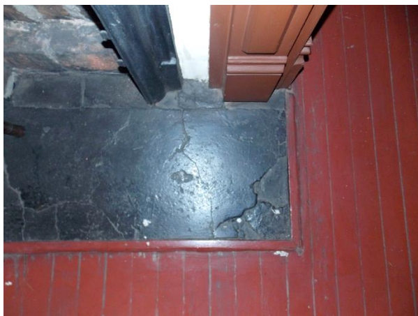
FIGURE 143. Cementitious fireplace hearth in Martin, Jr.'s and A.D.'s room.
