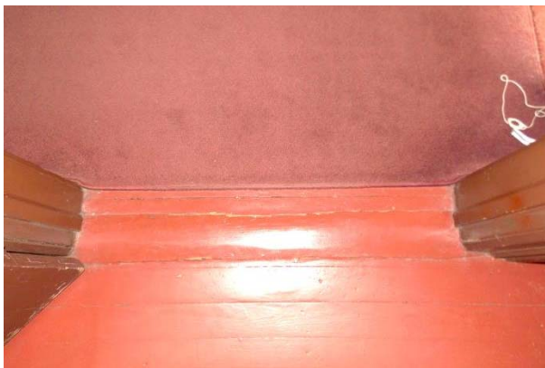
FIGURE 146. Typical historic threshold.
