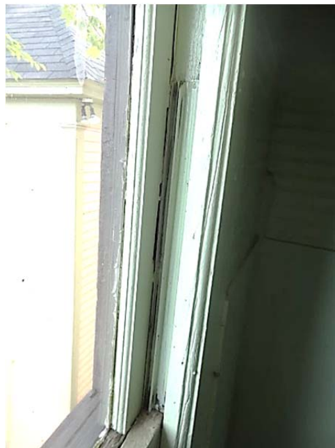
FIGURE 76. Sash pocket showing the aluminum sash track. Note that there is no sash chord. This window is likely not original.
