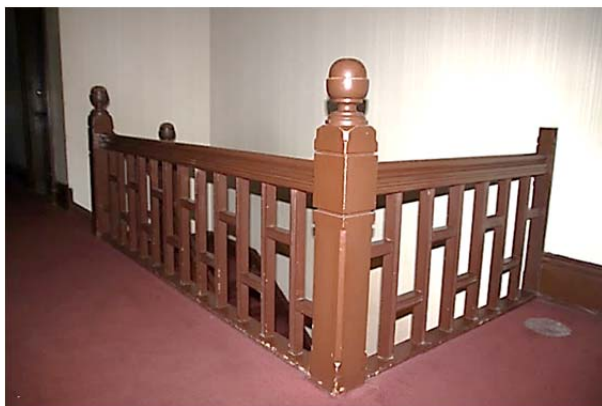
FIGURE 124. Railing and newel posts at the stair on the second floor.
