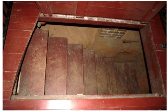
FIGURE 147. Floor scuttle and wood stair to basement.
