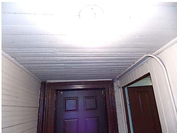
FIGURE 121. Single- and double-beaded board walls and ceiling at the second-floor back porch. Note vertical orientation of the beaded board on the right (west wall).
