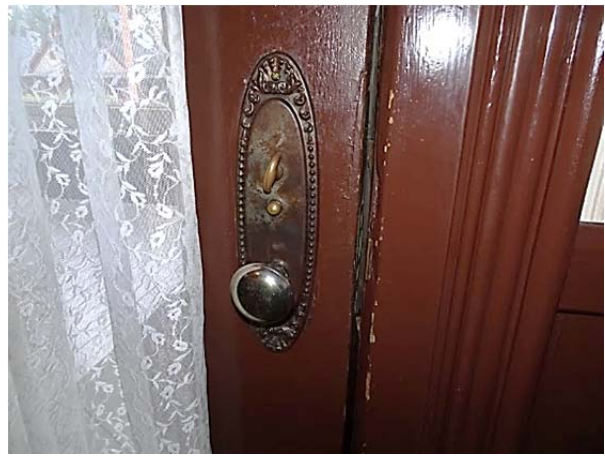
FIGURE 82. Main entrance – door knob and oval escutcheon plate.
