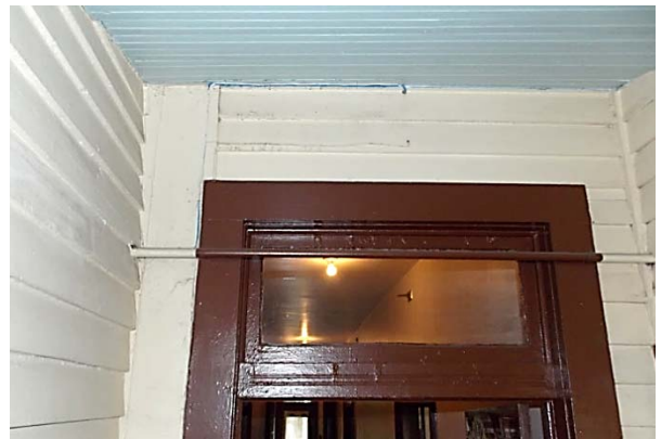
FIGURE 119. Clapboard siding and beaded wood ceiling at back porch.
