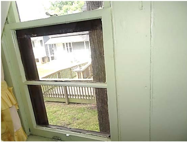
FIGURE 77. Lower sash of first-floor bathroom window.
