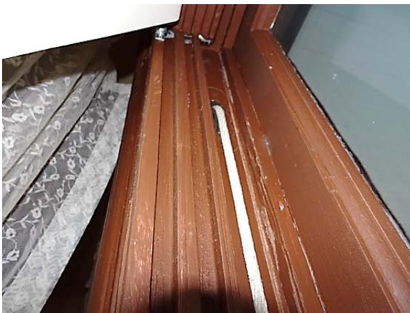
FIGURE 61. Typical rope chord at lower sash track.
