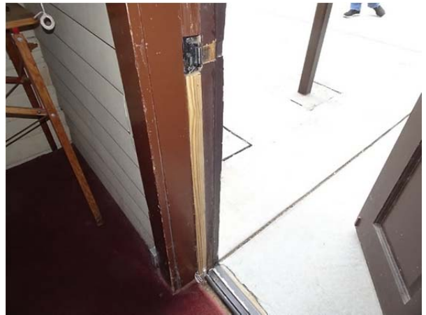
FIGURE 188. Unpainted dutchman repair to exterior door jamb, first floor rear hall.
