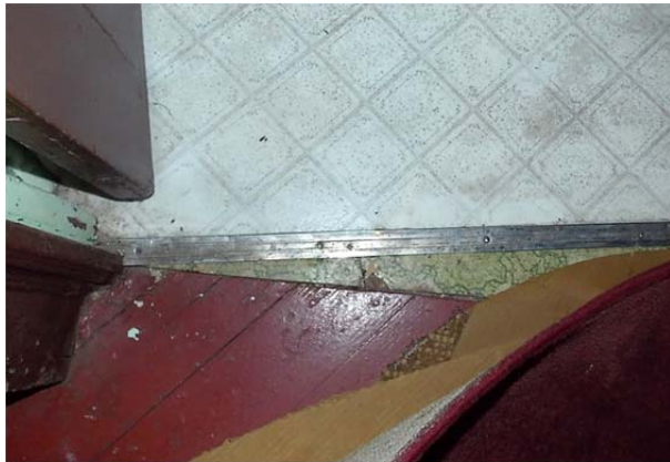
FIGURE 155. Exposure of older linoleum at bathroom.
