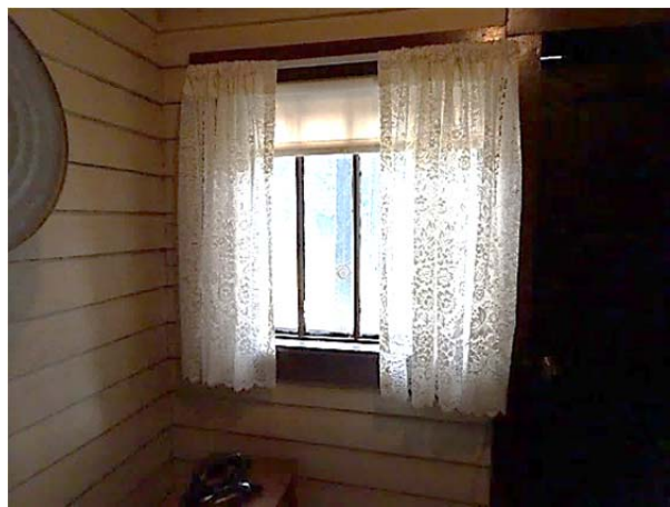
FIGURE 59. Overview of the multi-light fixed window at the south elevation.
