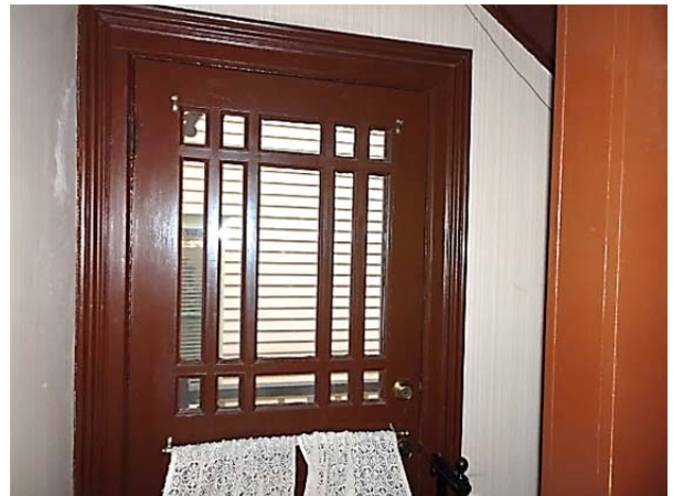
FIGURE 87. Multi-light glazed panel at side entrance door.
