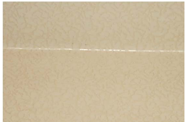
FIGURE 57. Typical wallpaper at ceiling and frieze.
