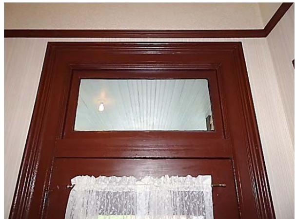
FIGURE 84. Overview of transom above main entrance door.
