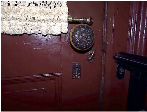
FIGURE 89. Brass hardware at side entrance door.
