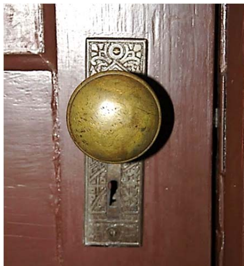
FIGURE 107. Mortised latch set with plain brass knob.
