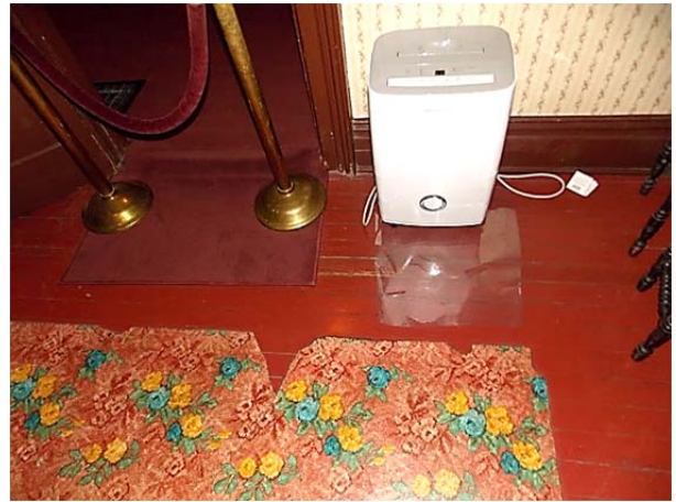
FIGURE 204. Deteriorated edges of vinyl floor cloth.
