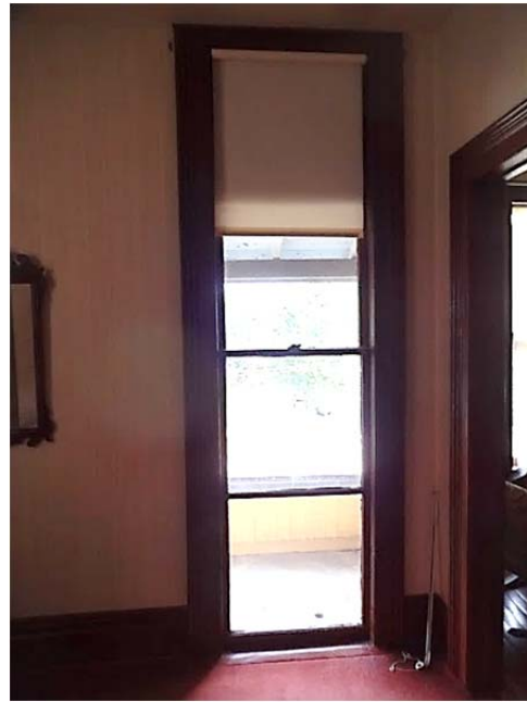
FIGURE 79. Second-floor hall window. Window provides access to balcony when sash is raised.
