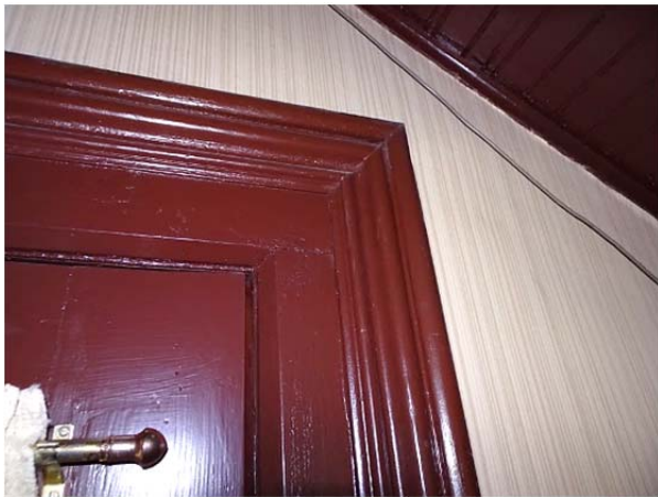
FIGURE 80. Typical bead mold casing at west side and main entrance doors.
