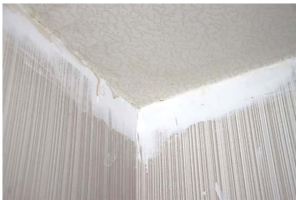
FIGURE 157. Joint compound repair at structural repairs.
