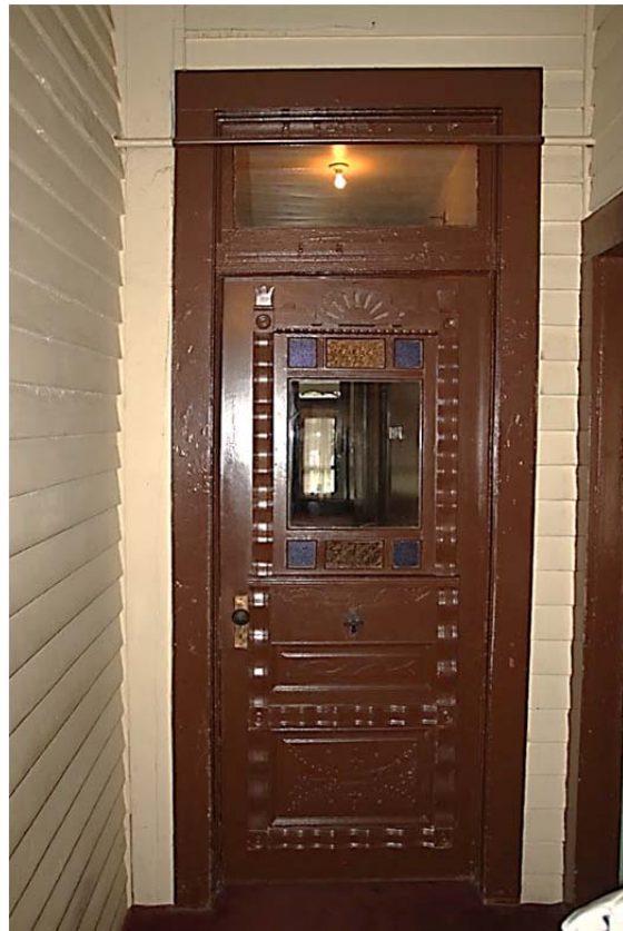
FIGURE 99. Door to central hall from back porch.
