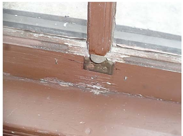
FIGURE 63. Typical surface-mounted brass lift at bottom rail.
