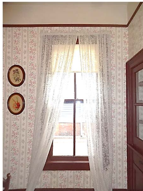
FIGURE 73. Typical two-over-two single-hung window unit.
