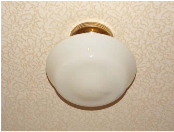
FIGURE 213. Typical non-original pendant fixture.
