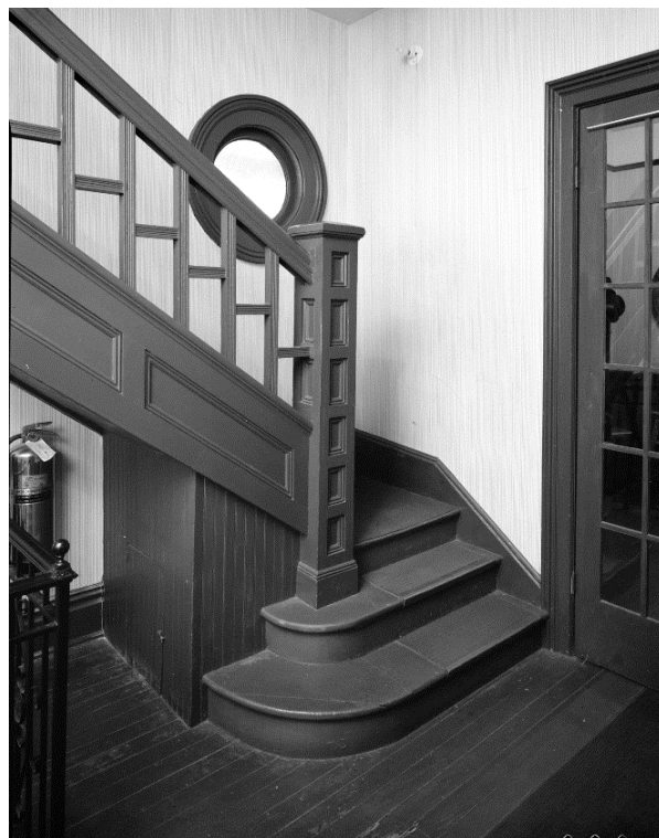
FIGURE 8. Staircase and newel post, circa 1983. (Source: HABS, HABS GA-1171-8)
