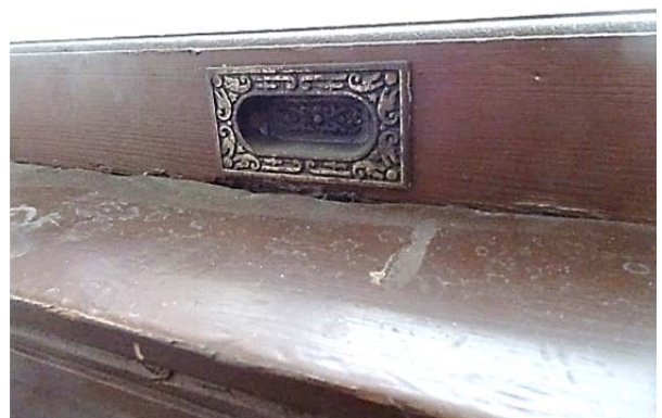
FIGURE 64. Decorative brass inset lift pocket at bottom rail.
