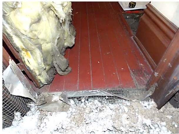
FIGURE 167. Access door to low attic from Martin Jr. and A.D.'s bedroom.
