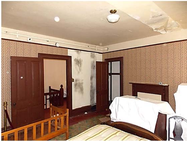
FIGURE 34. Overall view of birth room (S-4).
