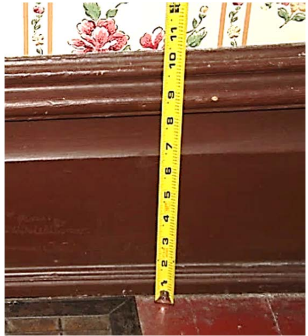
FIGURE 110. Typical wall base.
