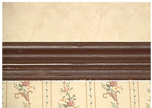
FIGURE 112. Picture rail matching cap molding.
