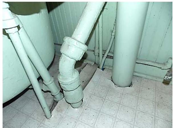
FIGURE 205. Sheet vinyl flooring in the first-floor bathroom.
