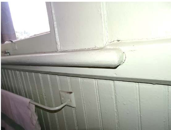
FIGURE 78. Detail of the window stool and chair rail.
