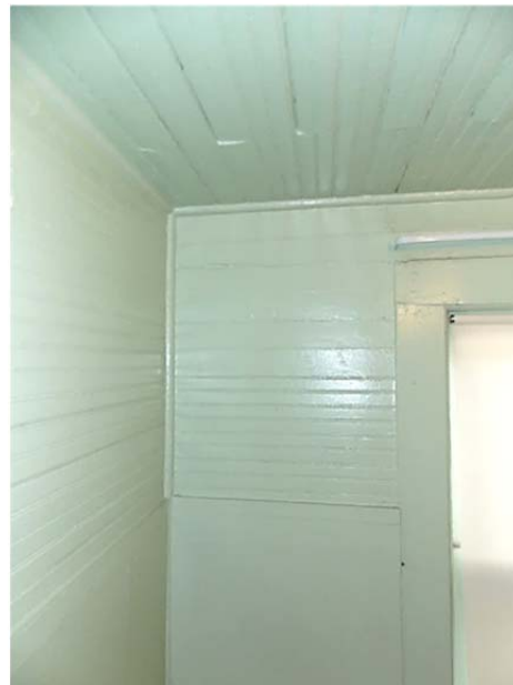
FIGURE 116. Beaded tongue-and-groove wall and ceiling panels in the first-floor bathroom.
