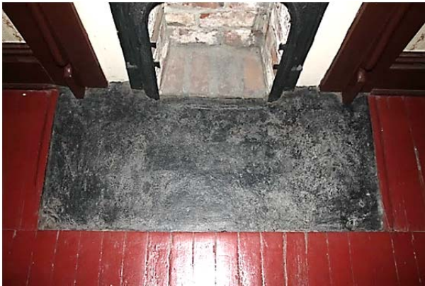
FIGURE 131. Hearth at Williams-King bedroom.
