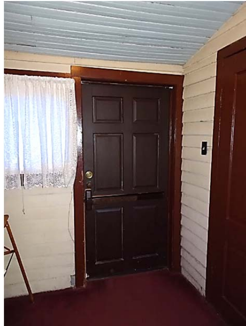
FIGURE 91. First-floor exit at south elevation.
