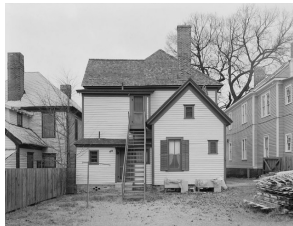
FIGURE 9. Location of compressor units at the rear of the Birth Home, 1989. (Source: HABS, HABS GA-1171-4)
