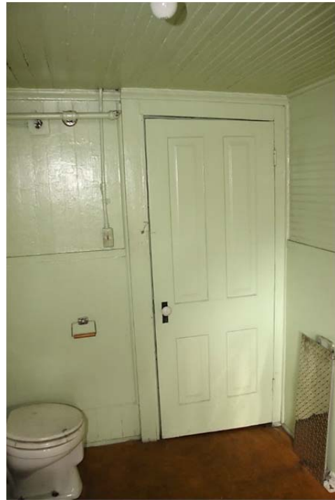
FIGURE 118. Beaded tongue-and-groove ceiling and wall paneling with gypsum board wainscot at the second-floor bathroom.
