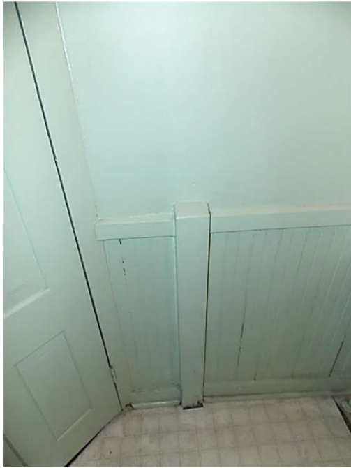
FIGURE 117. Beaded tongue-and-groove wainscot in the first-floor bathroom.
