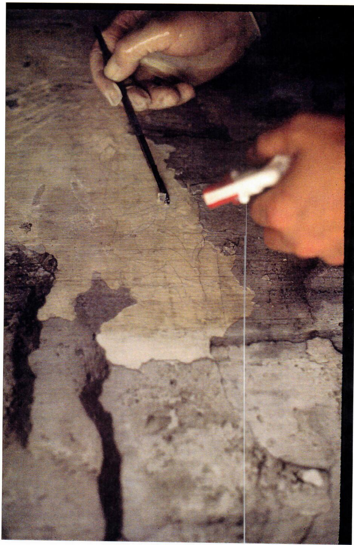
Detail of sample block on South Wall, S.E. room, 2nd floor. White wash coating which covers equestrian figure being mechanically removed.
