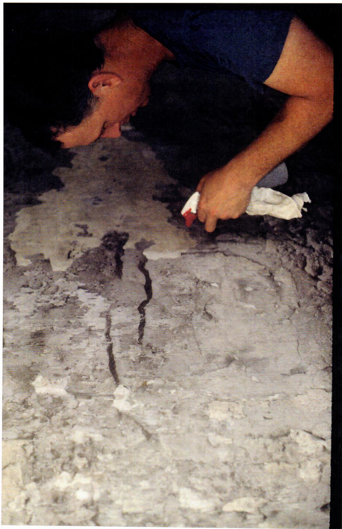
Detail of sample block on South Wall, S.E. room, 2nd floor. Graffiti bearing plaster being misted with distilled water to reveal obscure inscriptions
