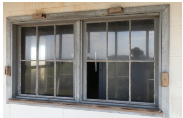
Figure 19. View of pair of six-light sash that replaced an earlier window before World War II.
