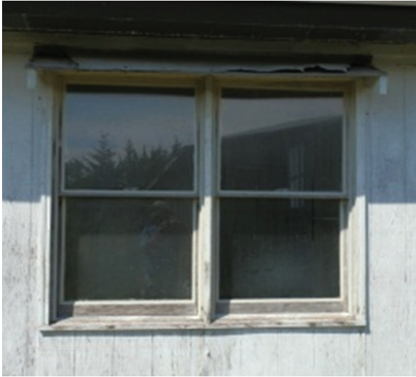
Figure 20. View of one-over-one windows that replaced earlier windows in the rear addition and on the east side of Room 104.
