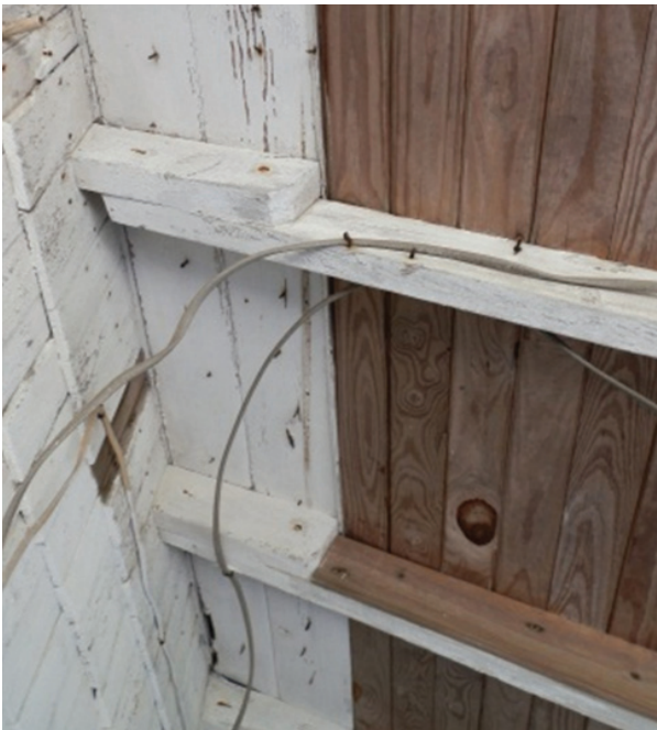
Figure 3. Detail view of rafter ends at rear of main block of house.
