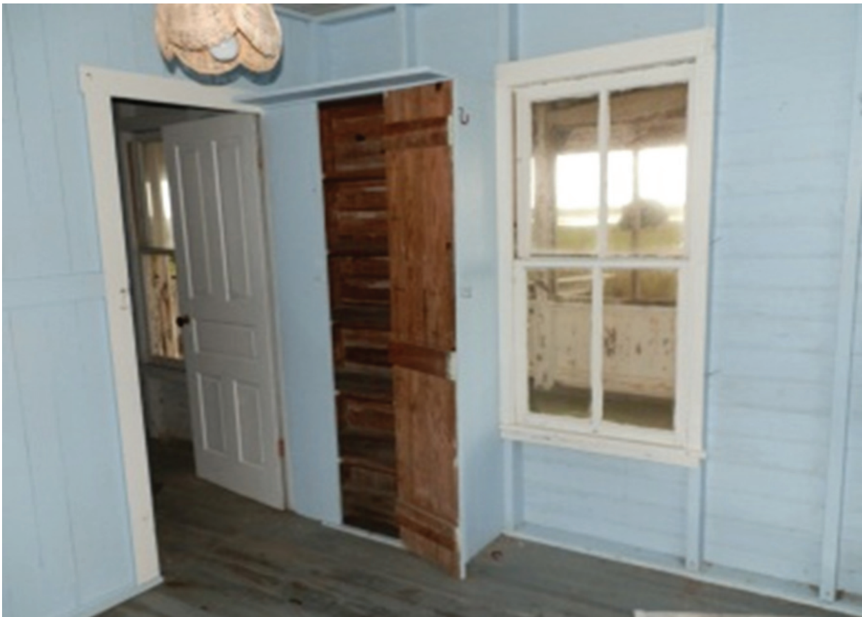
Figure 51. View northwest in Room 104.
