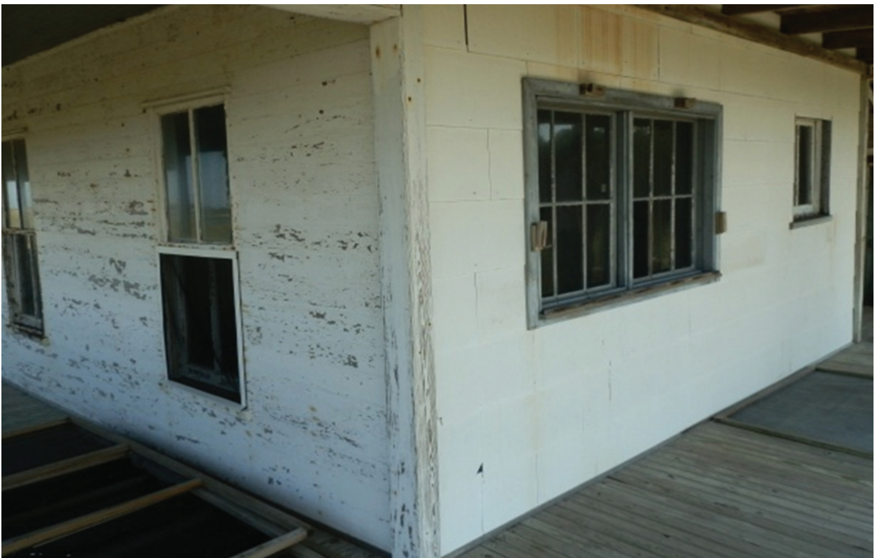
Figure 12. View of horizontally laid, flush siding (left), typical of original exterior siding, and added cement-asbestos siding that covered the historic house and its early additions.
