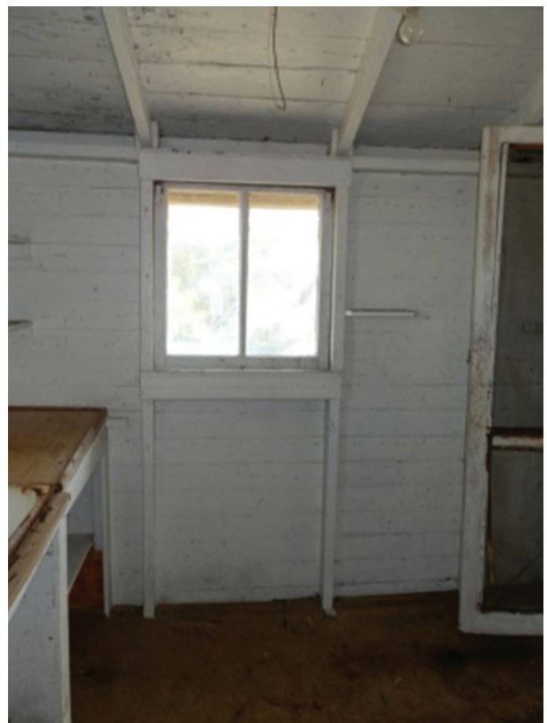
Figure 57. View of window on south wall of kitchen.
