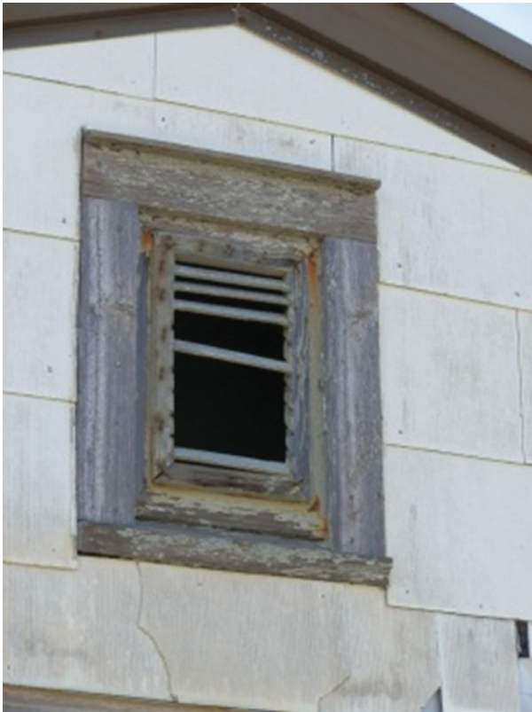
Figure 21. View of gable vent on east side of house.
