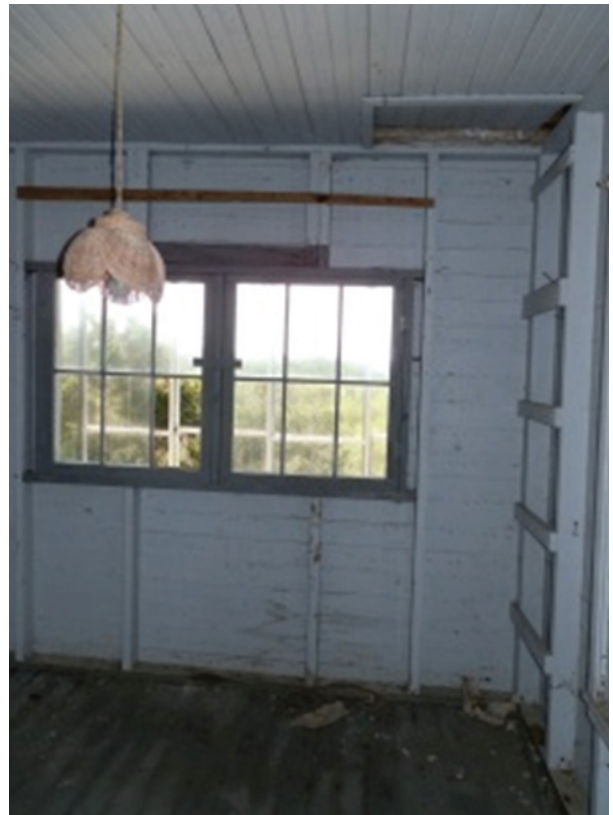
Figure 48. View west in Room 103.
