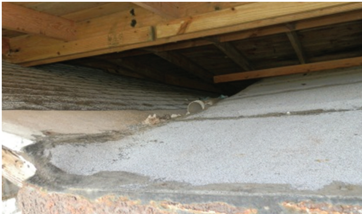
Figure 27. View of early asphalt shingles and rolled asphalt roofing present prior to construction of a new roof structure over the rear additions in the late twentieth century.
