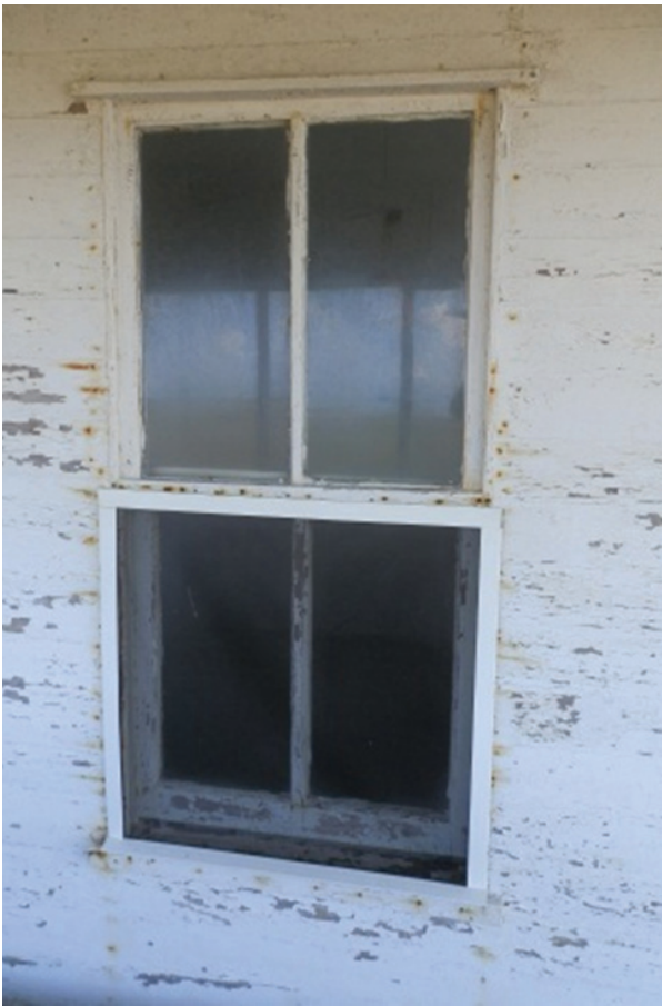
Figure 16. View of two-over-two windows typical of those used in the original house.
