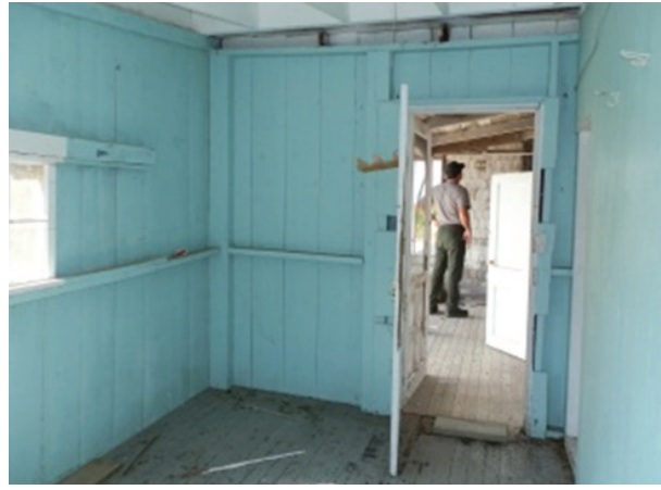
Figure 61. View northwest in Room 106.
