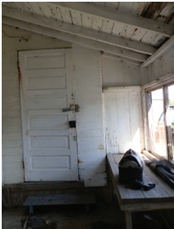
Figure 31. View of east end of rear porch showing door to kitchen.
