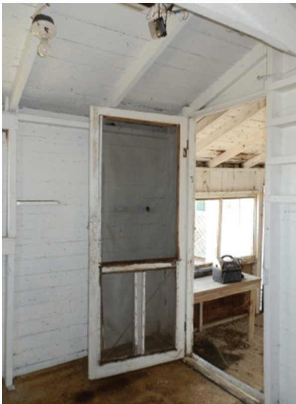
Figure 55. View southwest in kitchen.
