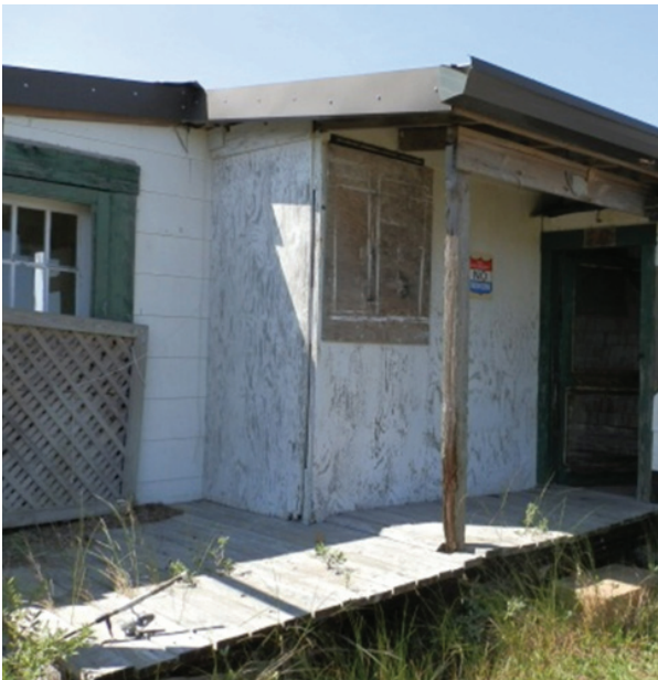
Figure 35. View of modern deck on east side of rear addition.
