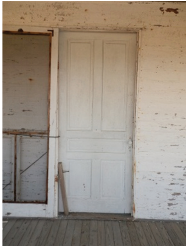
Figure 22. View of front door, typical of the five-panel doors used on the exterior and interior in the original construction.
