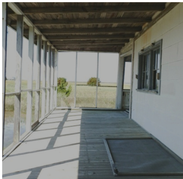
Figure 36. View north on west porch.
