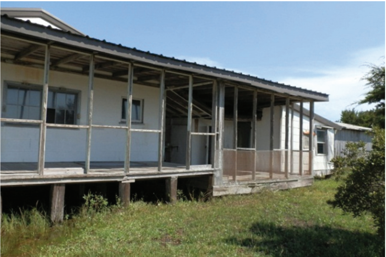
Figure 5. View of west elevation.
