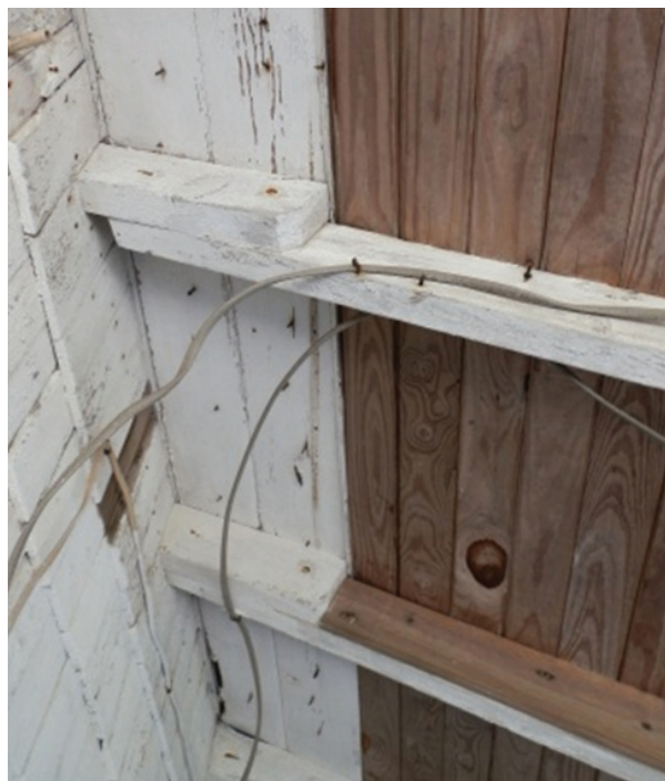
Figure 33. View of rafters for added south porch and their connection to the original rafter ends at the rear of the original house. Note the chamfered corners on the rafter ends.
