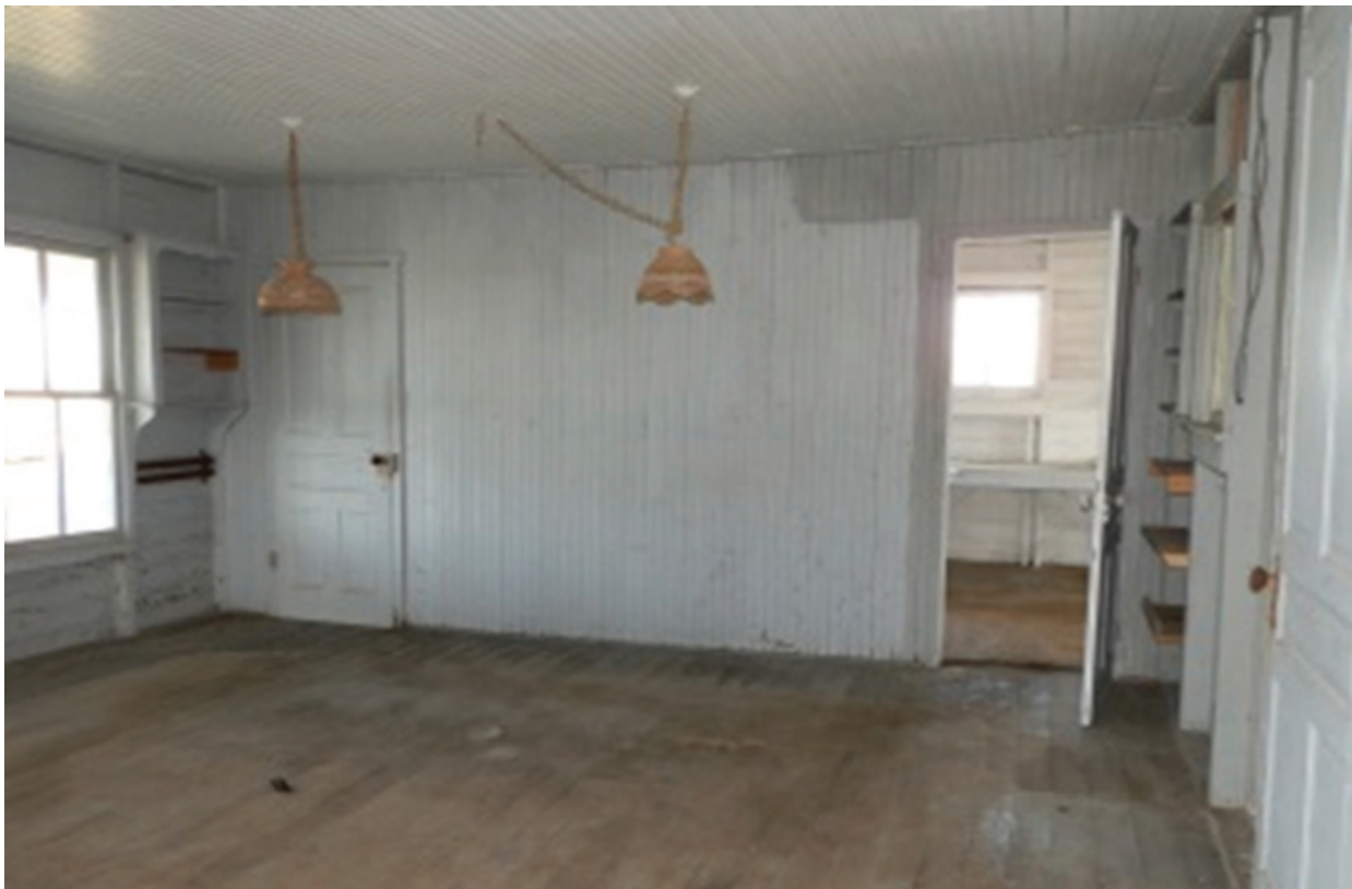
Figure 44. View northeast in Room 101.
