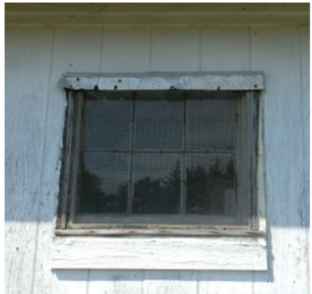
Figure 18. View of six-light sash typical used in earliest additions to the house.
