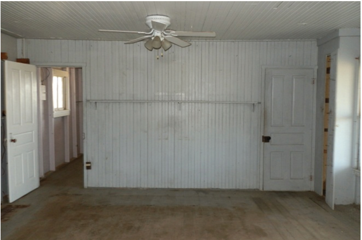
Figure 41. View west in Room 101.
