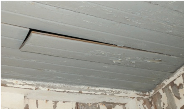
Figure 46. Typical tongue-and-grooving ceiling boards.
