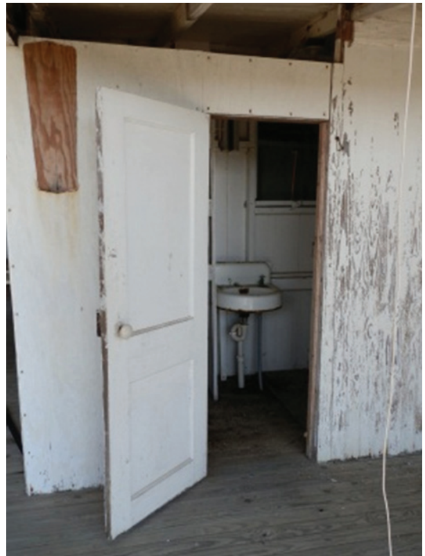
Figure 25. View of two-panel door with rim lock and porcelain knob that were part of the alterations and additions before World War II.
