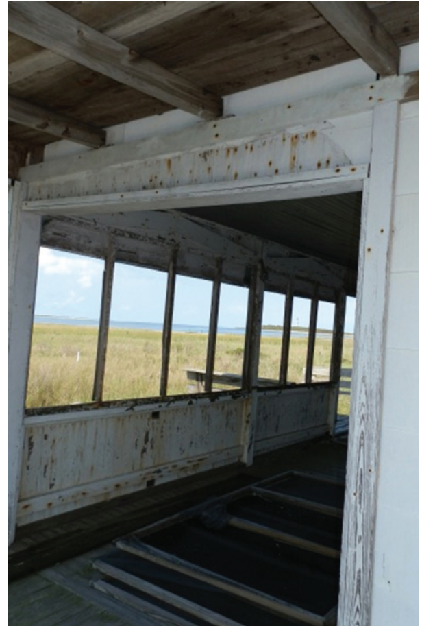
Figure 38. View at west end of front porch.
