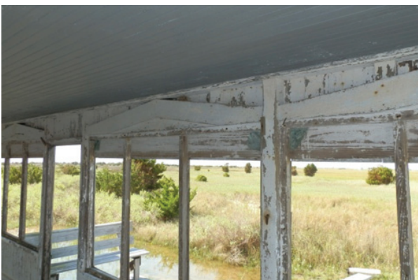
Figure 29. View of trusses and framing on front porch.
