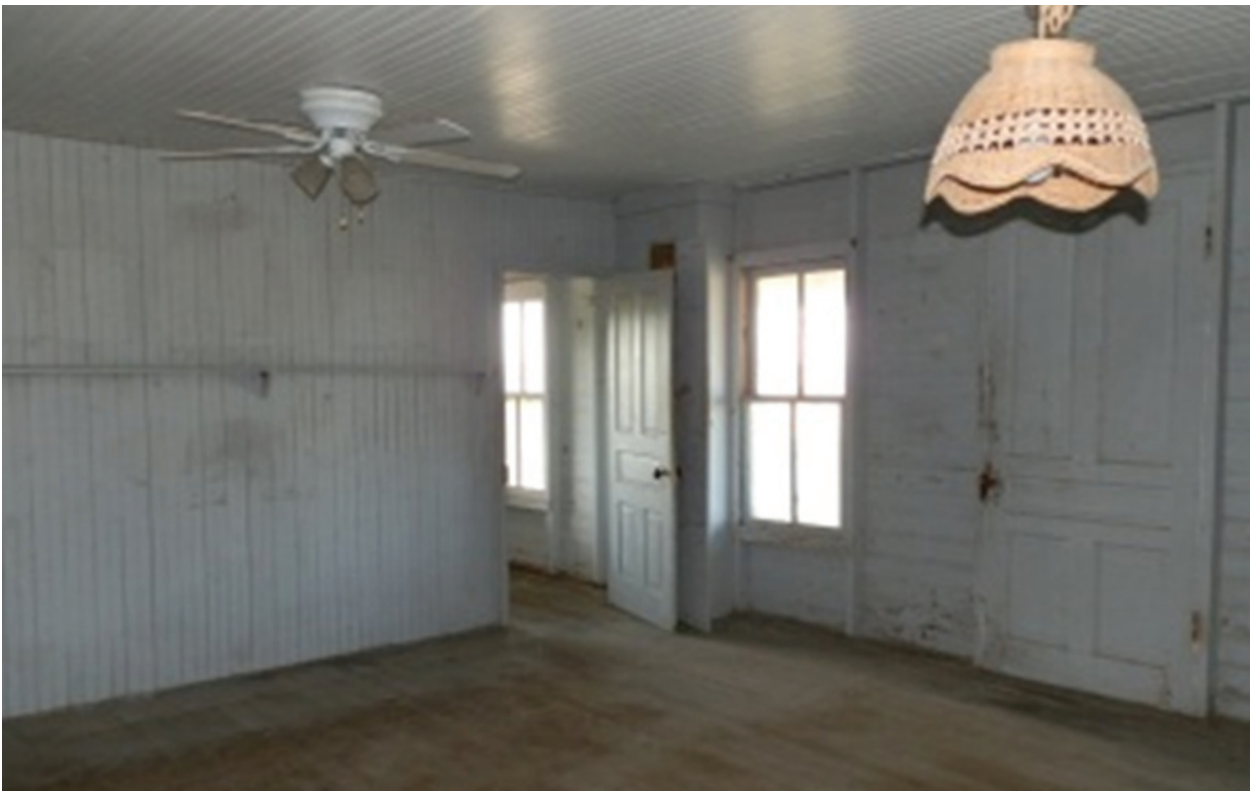
Figure 42. View northwest in Room 101.
