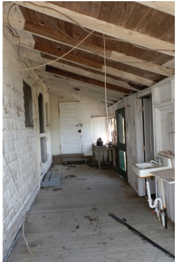
Figure 31. View east on back (south) porch.
