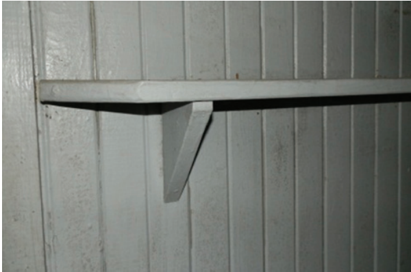
Figure 43. Detail view of shelf on west wall of Room 101.
