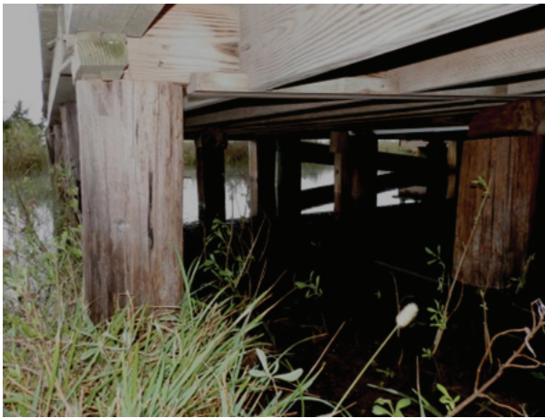
Figure 7. View of pilings from southeast corner of house.
