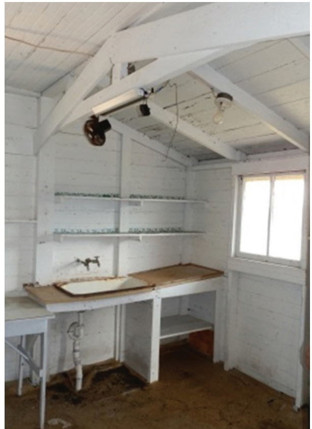
Figure 56. View southeast in kitchen.
