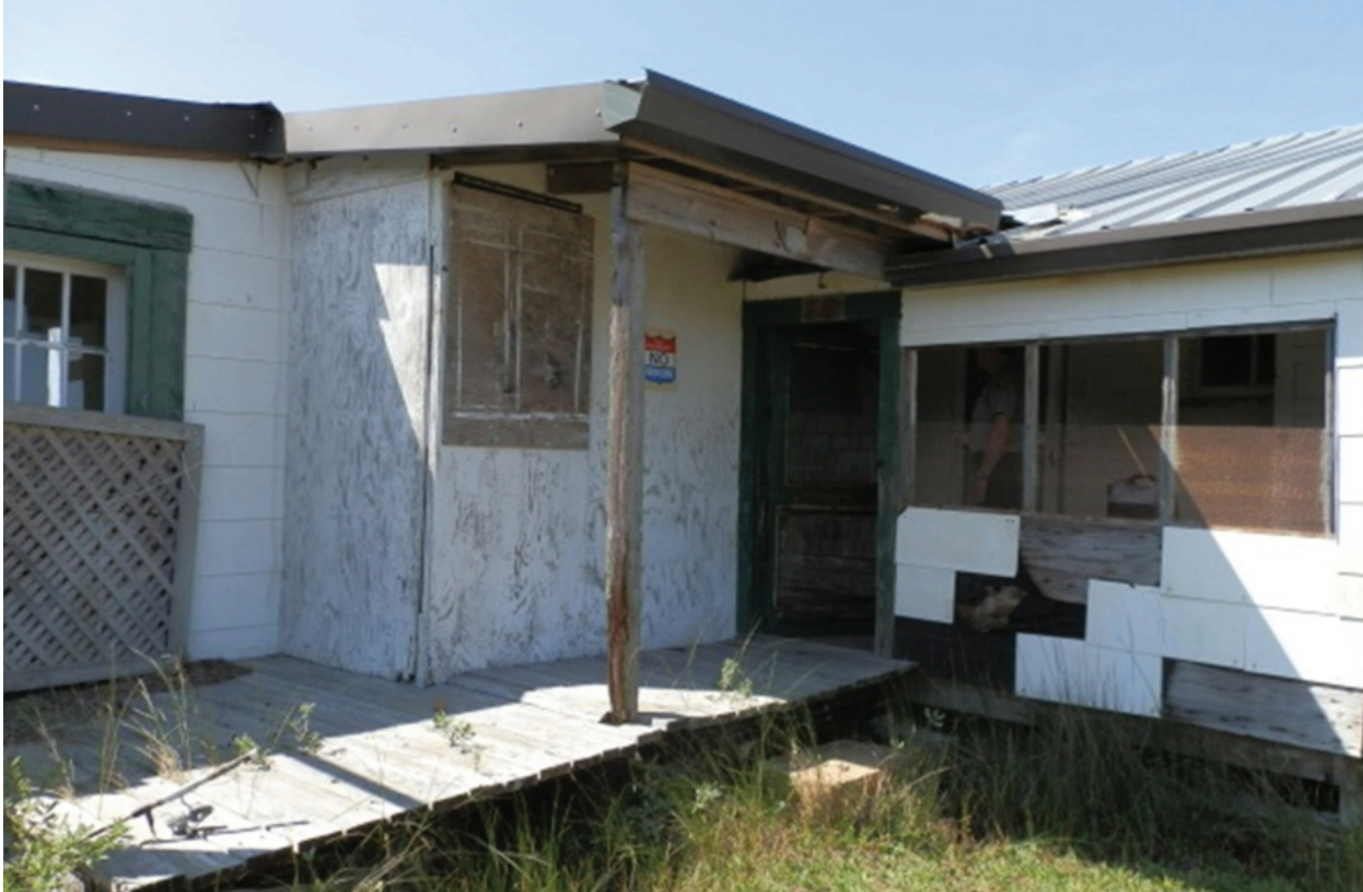
Figure 15. View of exterior finishes at rear of house. Note the plywood siding on the bathroom addition at center.
