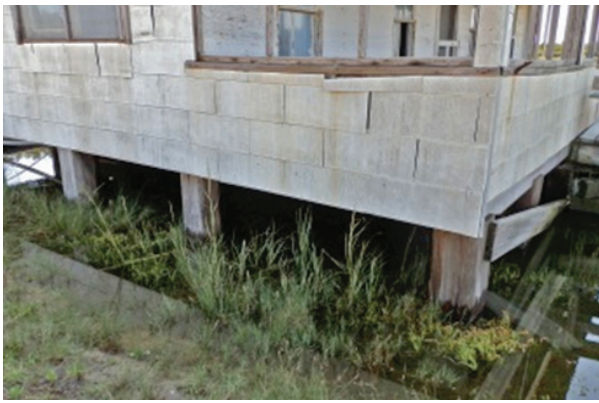
Figure 6. View of pilings at northeast side of original building.
