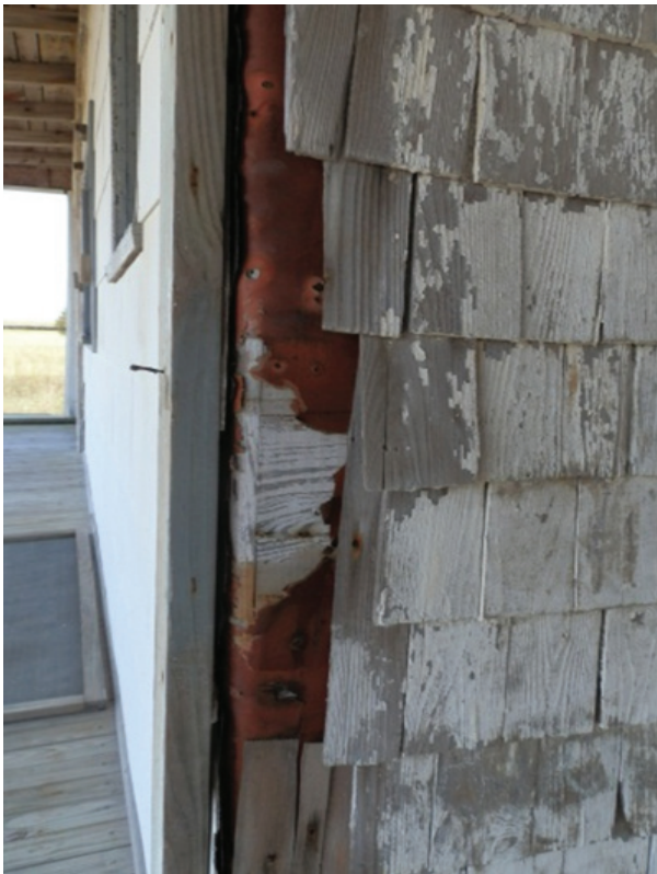
Figure 14. View of cedar shingles laid over original siding on back porch.
