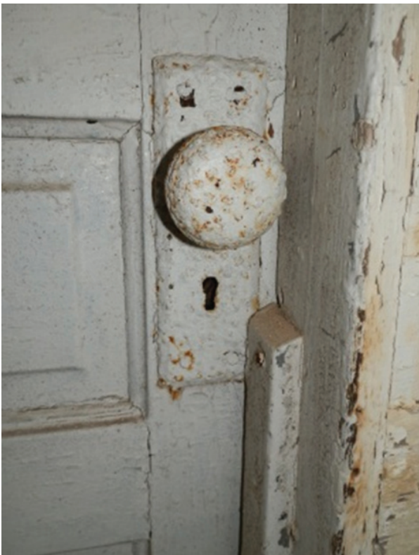
Figure 24. View of early twentieth century metal knob and escutcheon for a mortise lock.
