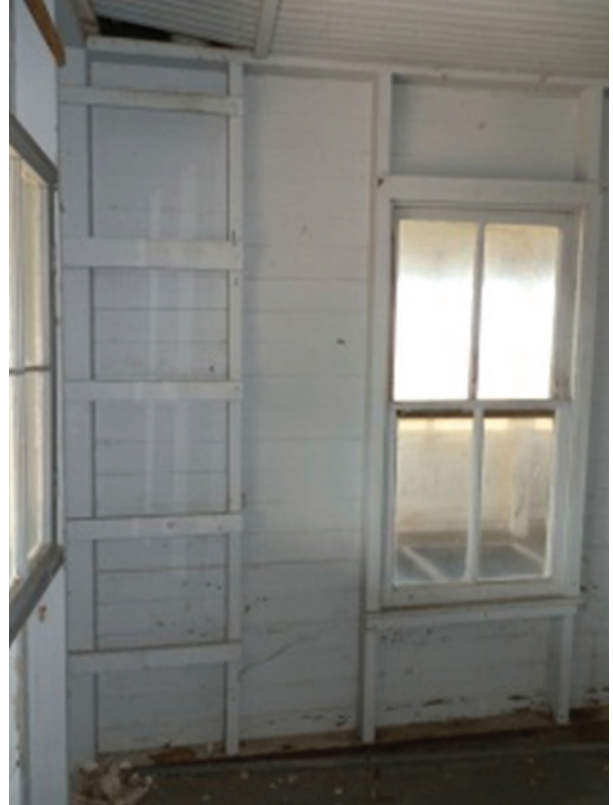
Figure 49. View of north wall of Room 103, showing ladder to hatch into attic.
