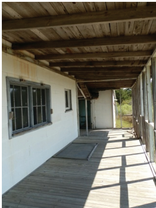
Figure 34. View south on added west porch.
