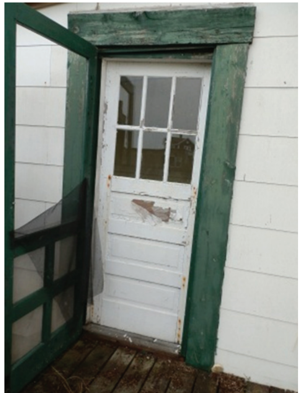
Figure 26. View of modern door installed on east side of Room 105.
