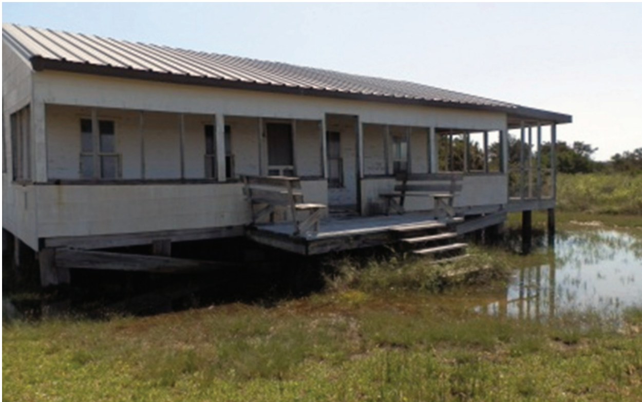
Figure 2. View of front (north) elevation.
