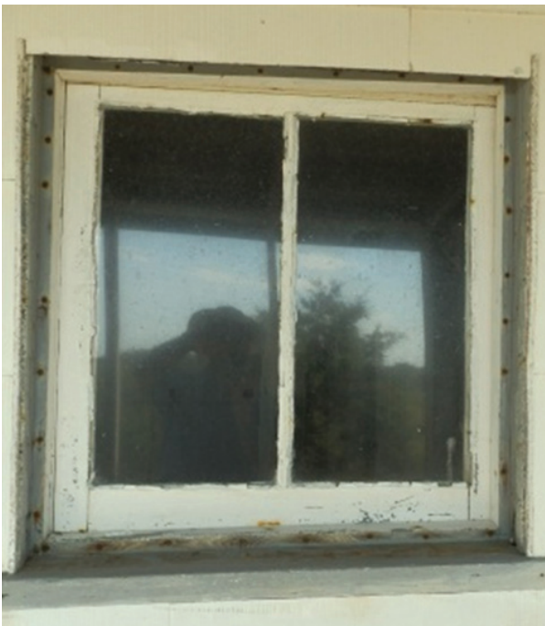
Figure 17. View of two-over-two sash, typical of those installed as casement windows in the original house.
