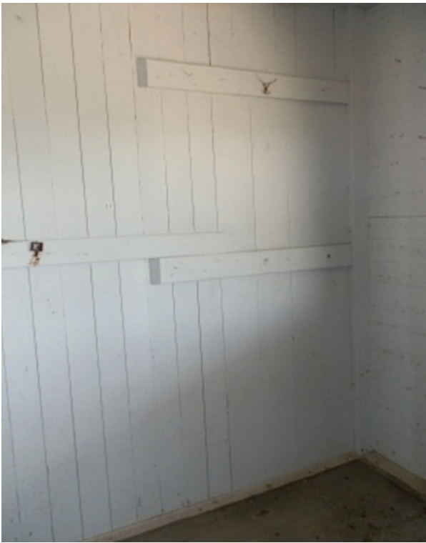
Figure 11. View of intersection of typical, unframed, interior curtain wall (left) and exterior wall (right). The horizontal members here are not structural; the vertical, tongue-and-groove paneling of the curtain wall is held in place by nailers at the floor and ceiling.
