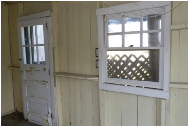
Figure 58. View northeast in Room 105
