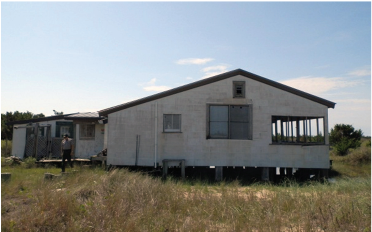
Figure 3. View of east elevation.
