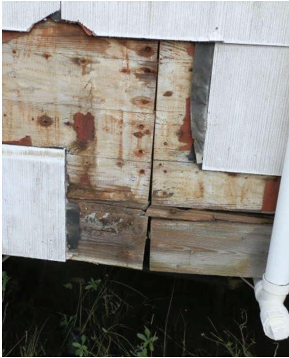
Figure 2. View of break in original siding where the south half of the present kitchen meets the main block of the house.
