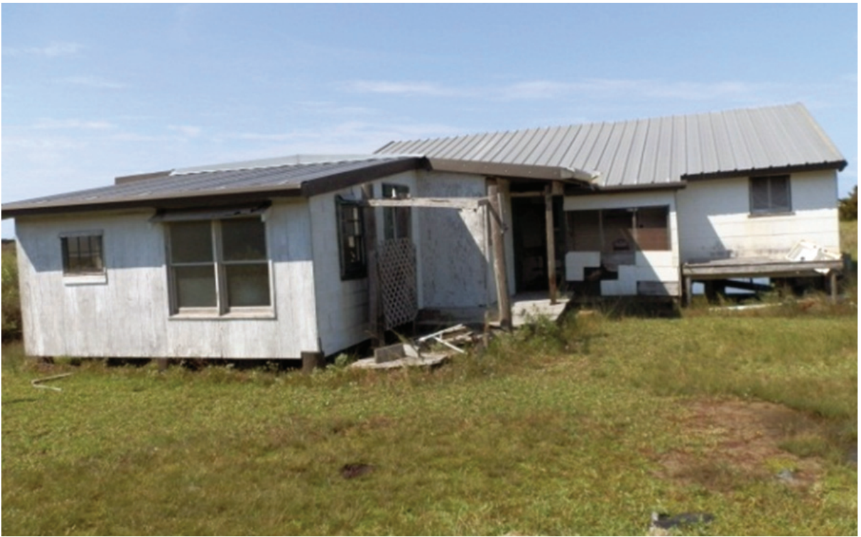
Figure 4. View of south elevation, showing rear additions.
