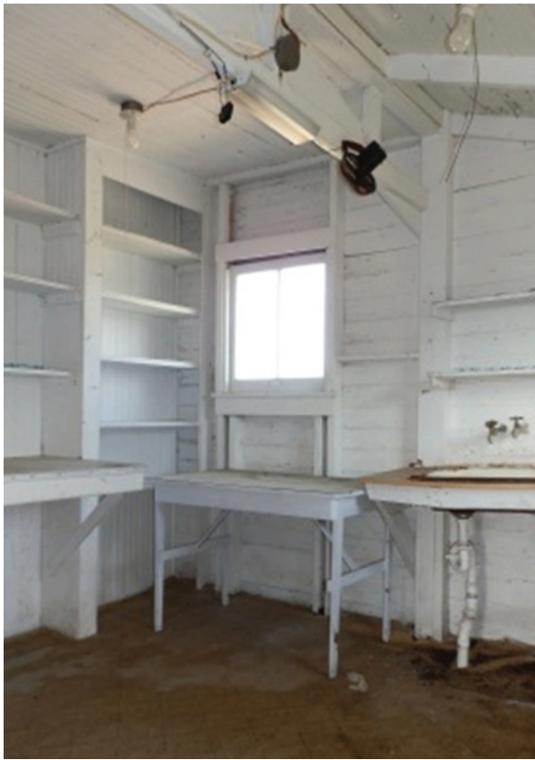
Figure 54. View northeast in kitchen.
