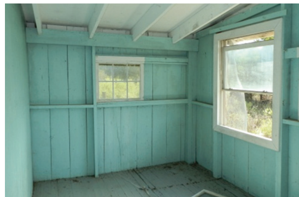
Figure 10. View of framing of Room 105, one of the modern additions to the house.
