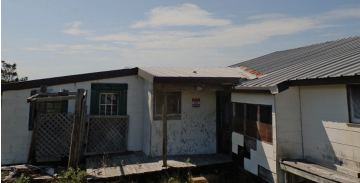
Figure 26. View of junction of added roofs and the rear shed of the original roof, now covered with modern metal roof covering.
