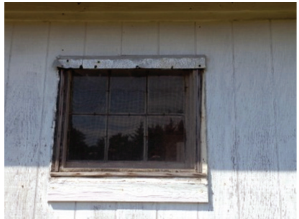
Figure 13. View of vertical siding used in the early twentieth century bedroom and half-bath additions.
