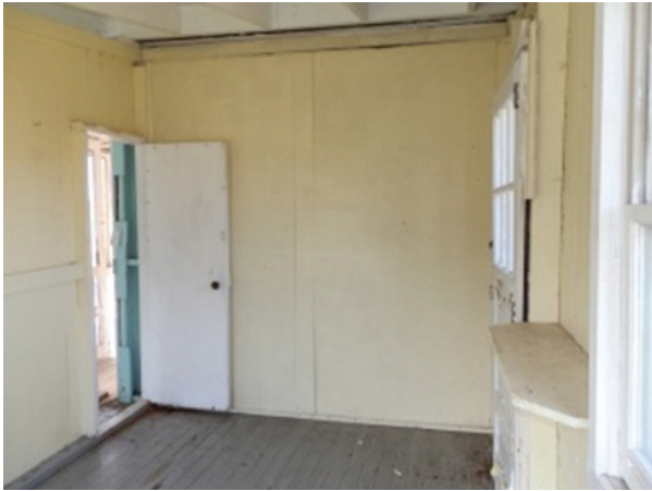
Figure 59. View north in Room 105.
