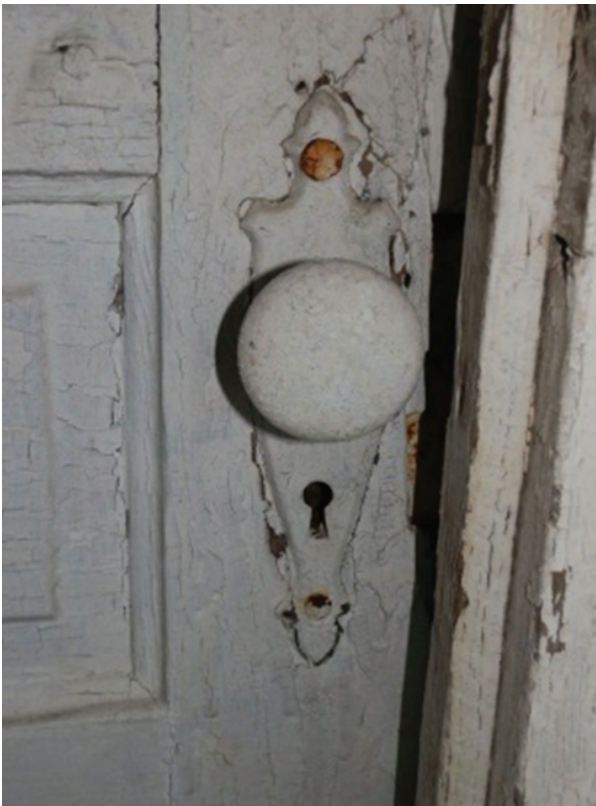
Figure 23. View of white porcelain door knob and colonial-revival escutcheon for what are presumably original mortise locks at the front and back doors.
