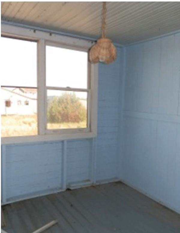
Figure 51. View southeast in Room 104.
