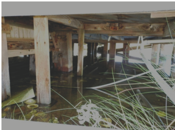
Figure 8. View of pilings at rear of house.
