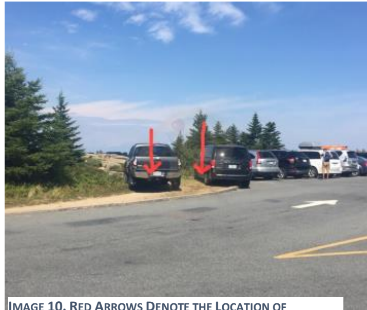
IMAGE 10. RED ARROWS DENOTE THE LOCATION OF ADDITIONAL COPING STONES
