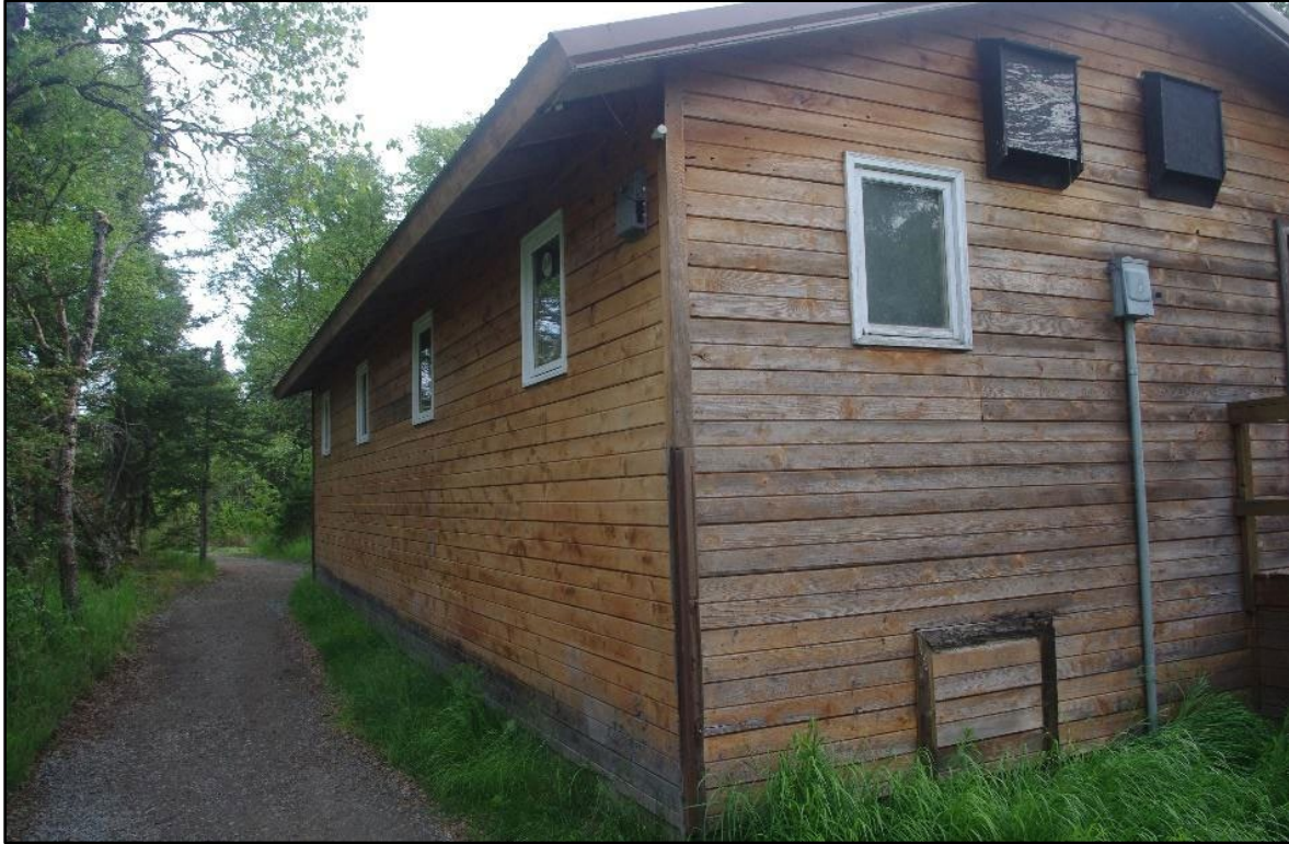
Photo showing the microphone on the structure at Brooks Camp (building corner), the location of the nearby bat houses (black boxes attached to building), and the surrounding vegetation.
