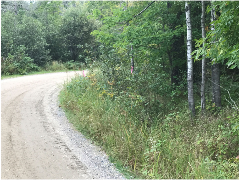
Photograph 7 (48.50097 N, -92.63843 W) – Wetland 5 view is 27° NE looking at a previously unmapped wetland habitat adjacent to an active road, Wetland 5 drains via a 12-inch culvert into Wetland 6. Photo Date 11 September 2019 – P. Sharpe.
