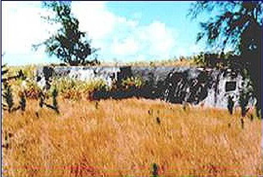
Air Raid Shelter
