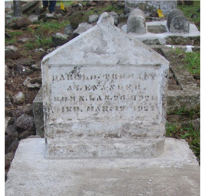
#15 After removing loose layers of paint
