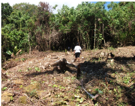
Bai er a Olilai, Ngiwal State Site Restoration Project in its clearing and cleaning stage.
