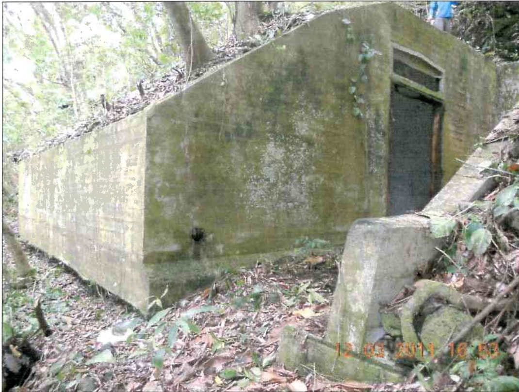
View facing Southeast
