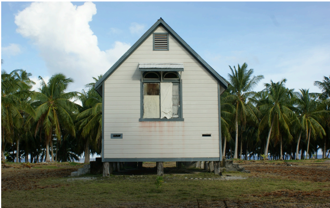
Photo 6: East side of church at Taulaga
