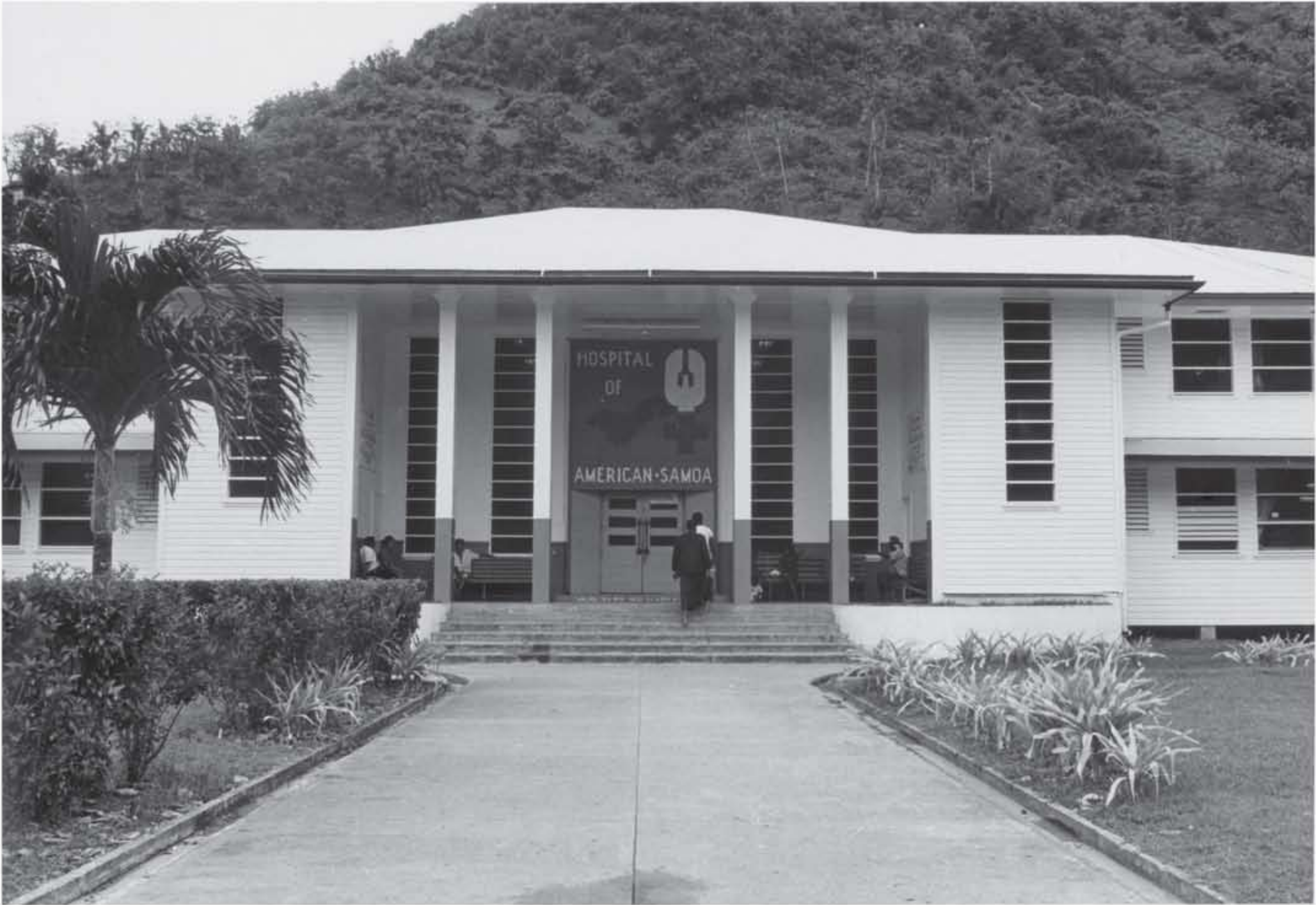
The Old Hospital of American Samoa Utulei; The A.P Lutali Executive Office Building currently occupies this site.
