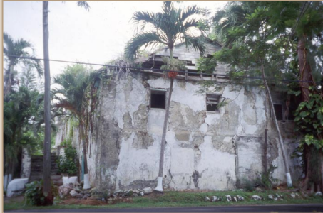
Before: Southside elevation, adjacent to Route 4.
