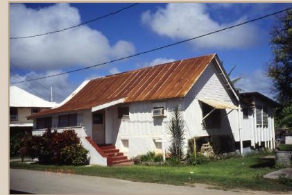
Mariano Leon Guerrero House before restoration
