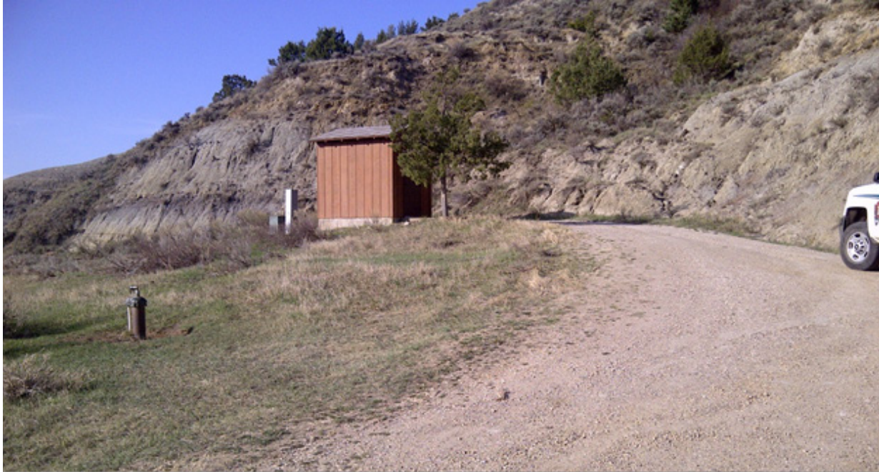
Figure 2.1. Juniper well house in the North Unit of Theodore Roosevelt National Park (May 4, 2018; photograph courtesy of William G. Eldridge, U.S. Geological Survey, Dakota Water Science Center).
