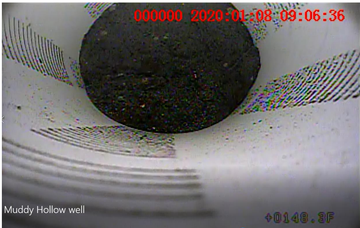
Accumulation of black sediment at the base of the well.
