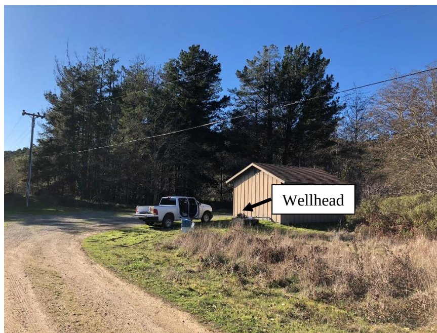
Figure 2. View of the Muddy Hollow well site with access road, overhead power lines and treatment building. Muddy Hollow wetland is immediately behind the water treatment building. View to the southwest, photo date January 9, 2020.
