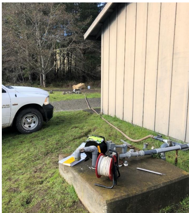
Figure 4. Test discharge was slowed by hay bales to prevent erosion (in background). Water quality parameters were measured at this location. View to the southwest, photo date January 9, 2020.
