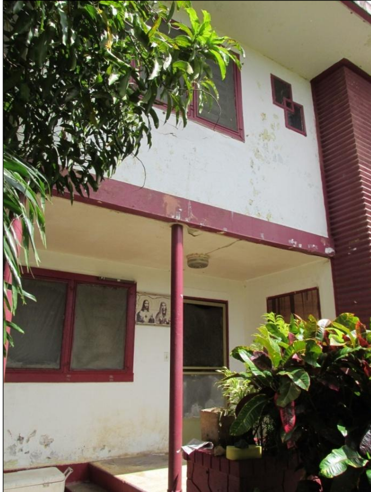
Figure 37. Herrera House, detail of north side of west facade.
