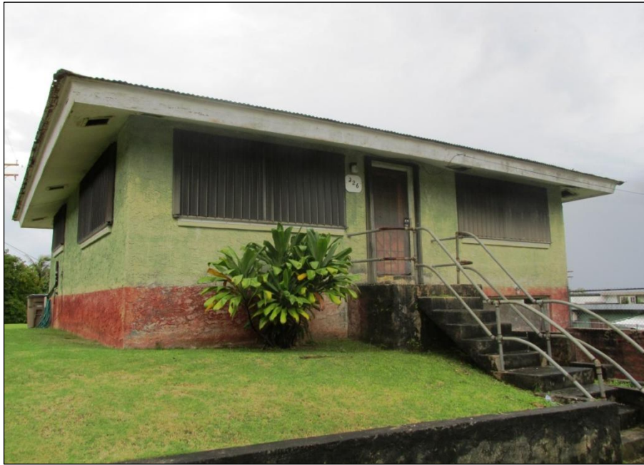
Figure 45. Property No. 8, Hopkins House, north facade with view of east elevation.
