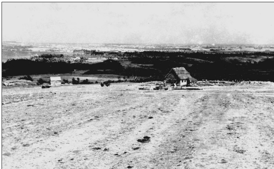
Figure 8. Beginning of construction in newly plowed Santa Rita village, 1945 (photograph on file at MARC).
