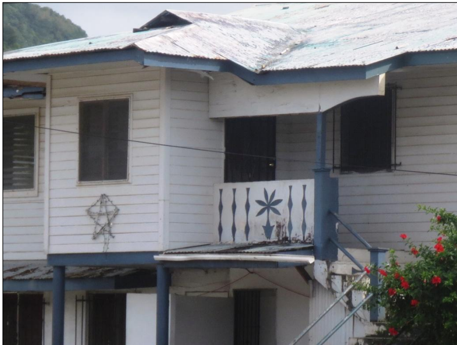
Figure 40. Sablan House, detail of second-floor duplex entry.
