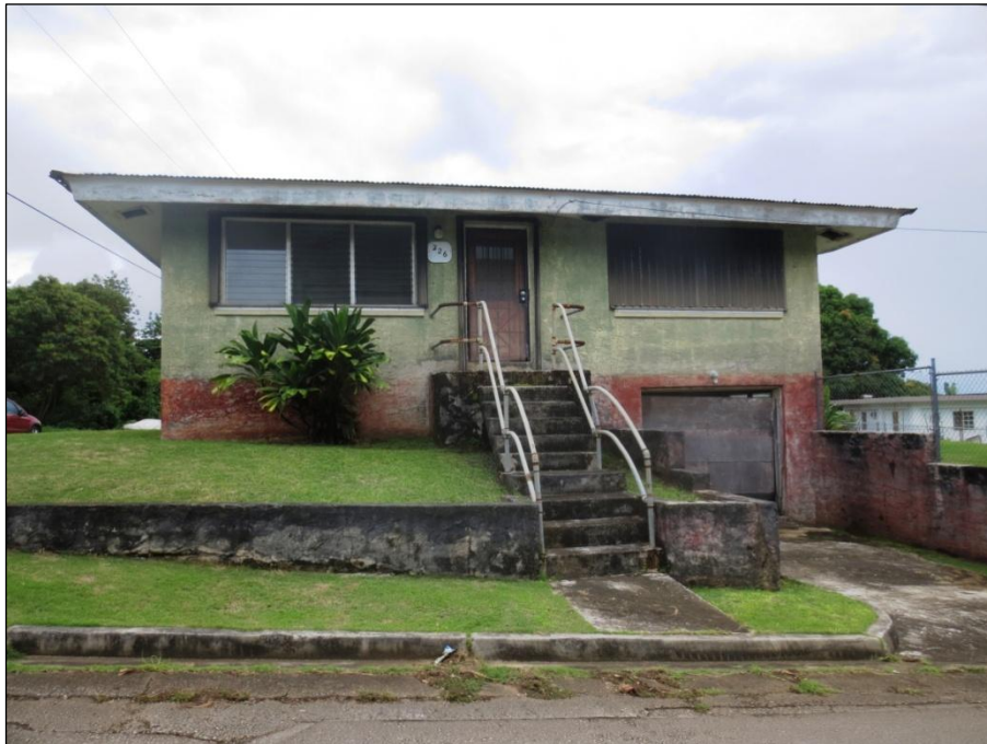
Figure 46. Hopkins House, north facade. Note cellar on the west end of the facade.
