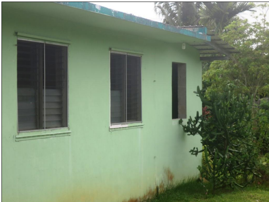
Figure 74. Mafnas House, detail of corrugated metal roof addition on west end of north elevation.
