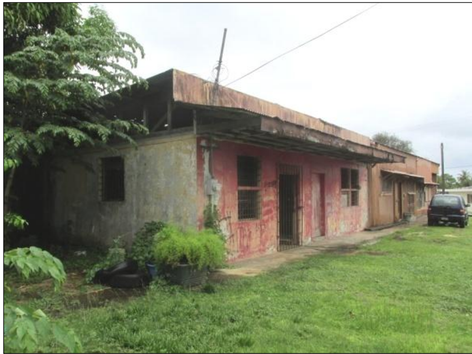
Figure 50. Kang Store; facing west.
