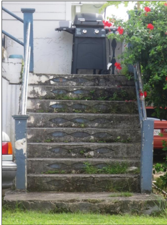
Figure 41. Sablan House, detail of second-floor stairway with steel handrails supported by square-shaped columns and folk concrete design elements.
