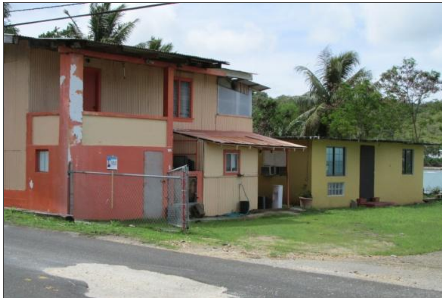
Figure 59. Tanaka House with view of massive porch and entryway, facing southeast.
