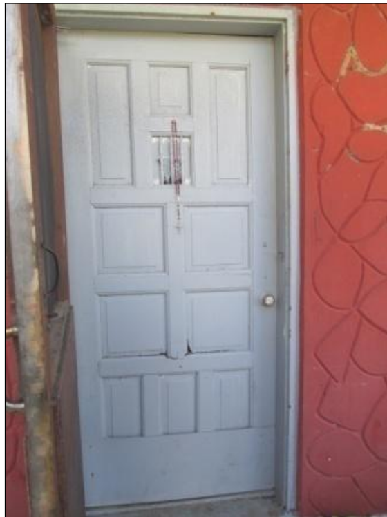
Figure 66. Traditional wood-paneled door (painted white) on Taitague Meno House.
