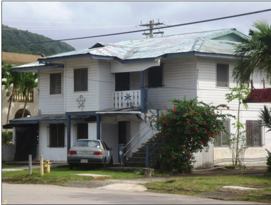
Figure 39. Property No. 7, Sablan House, north facade.
