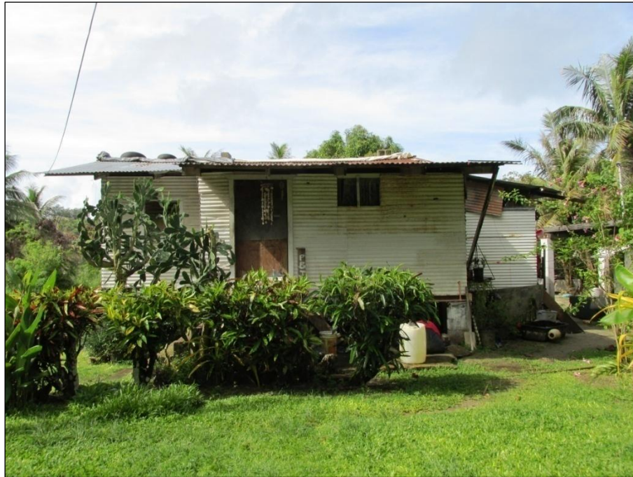
Figure 52. Property No. 11, Sanchez House, north facade.
