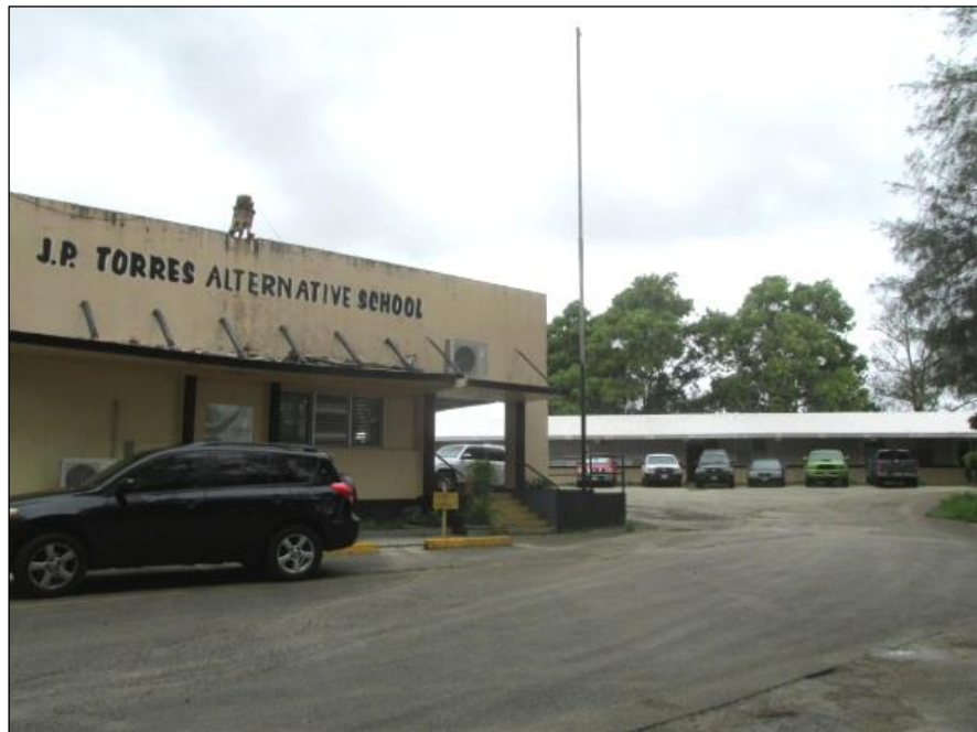
Figure 22. Administration building of J. P. Torres Alternative School with classroom building in background.
