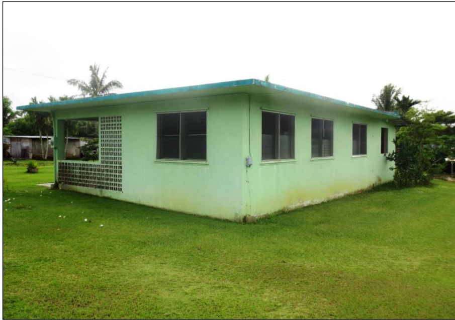
Figure 73. Mafnas House, east facade and north elevation.
