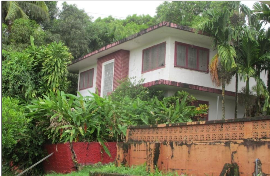
Figure 32. Property No. 6, Herrera House as viewed from Calle de los Marterres Street, facing northeast.
