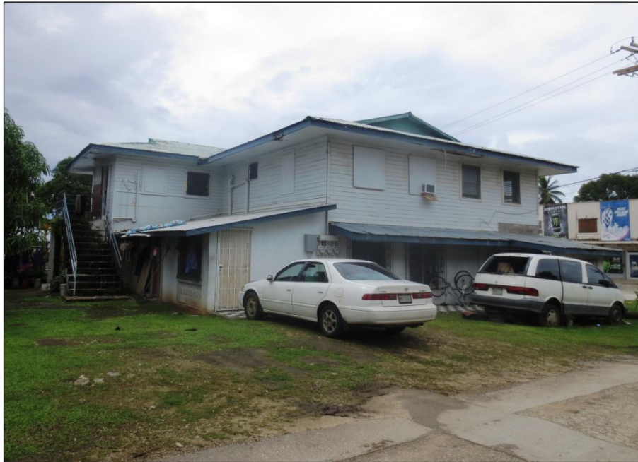
Figure 43. Sablan House, east and south elevations.
