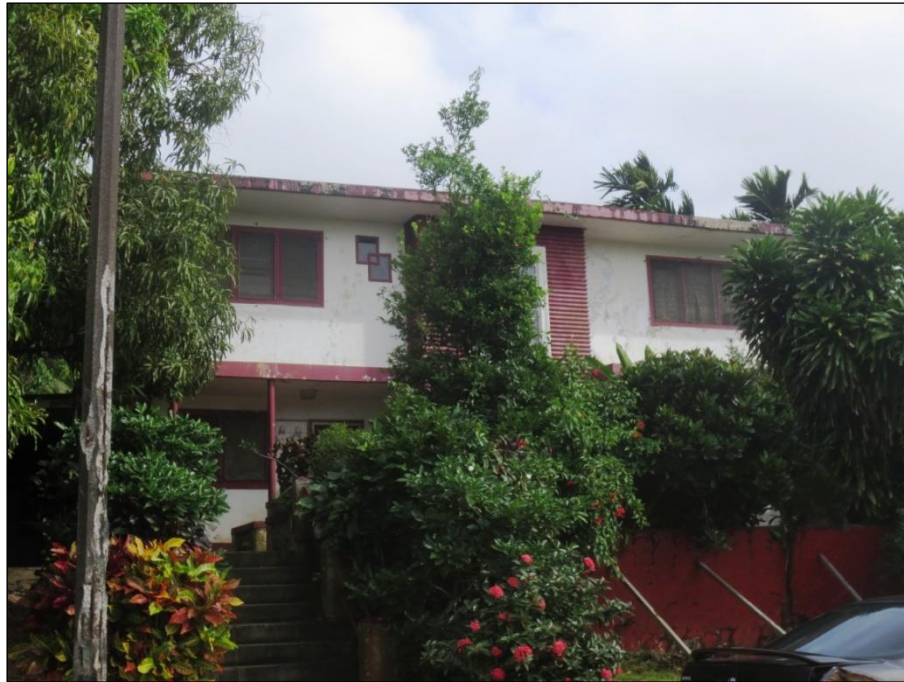
Figure 34. Herrera House, west facade with view of front porch.
