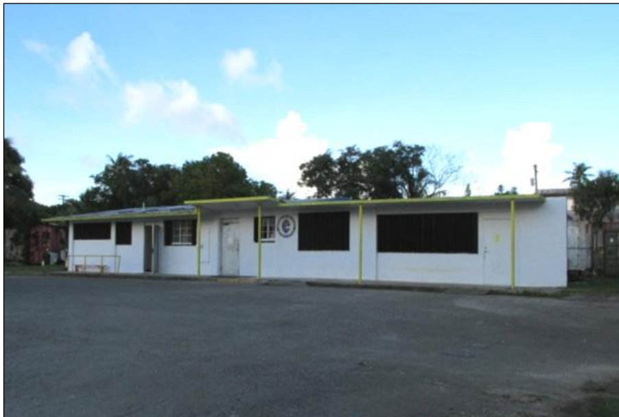
Figure 69. Property No. 20, Old Navy Dispensary/Talofofu Mayor's Office in current condition; facing east.
