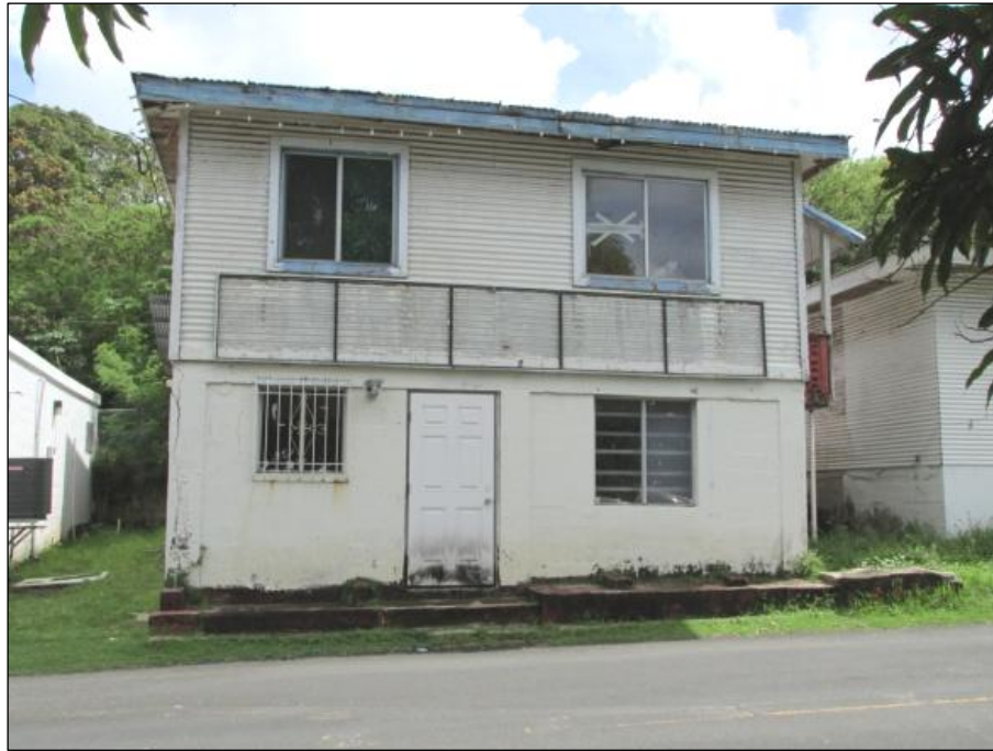
Figure 60. Property No. 13, Quinata House; facing north.
