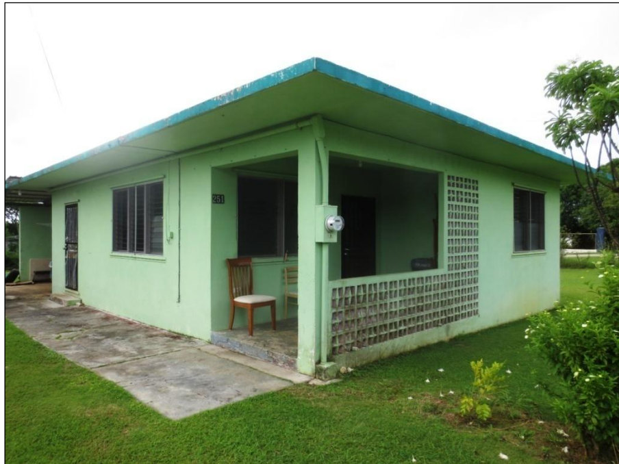
Figure 72. Mafnas House, east facade and south elevation.
