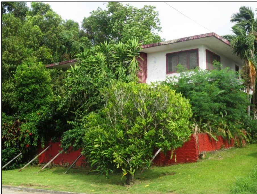
Figure 33. Herrera House, west facade and retaining wall obscured by thick vegetation.
