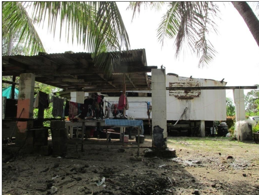
Figure 57. Sanchez House, outdoor kitchen area adjoining west elevation.
