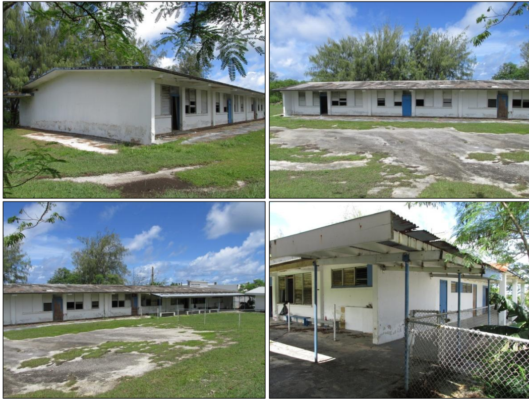
Figure 64. Property No. 17, Inarajan Elementary School. Clockwise from top left: north elevation; west elevation with classroom entry; south end of west elevation and south elevation, and west elevation (note awning on south side).
