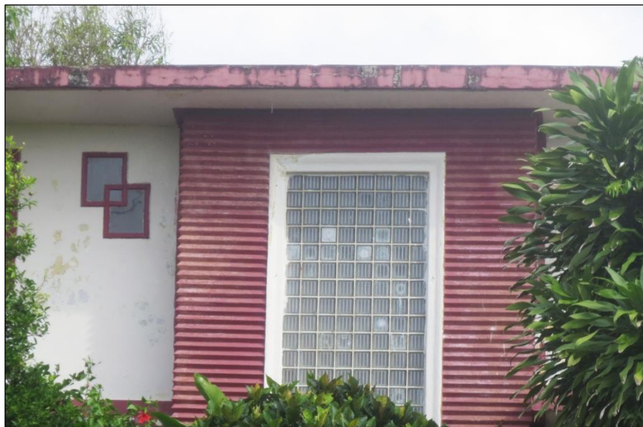
Figure 35. Herrera House, detail of west facade's concrete pilaster and window configuration.
