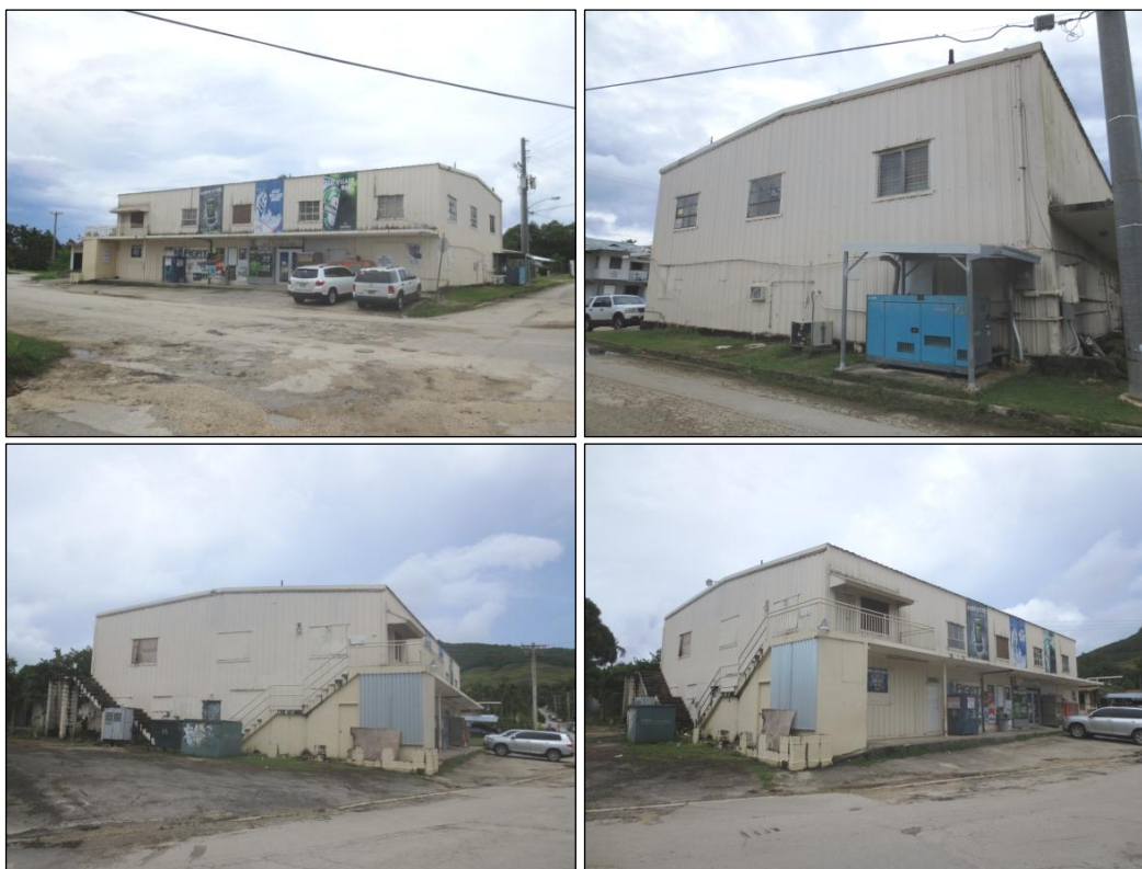
Figure 51. Property No. 10, Sablan Store. Clockwise from top left: south facade; east elevation (note replaced hopper window with louvers); west elevation and south facade; and west elevation (note boarded windows).
