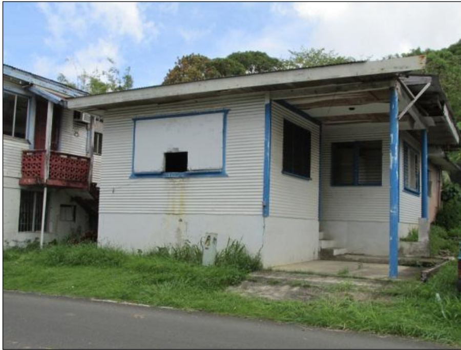
Figure 61. Property No. 14, Gofigan House; facing north.
