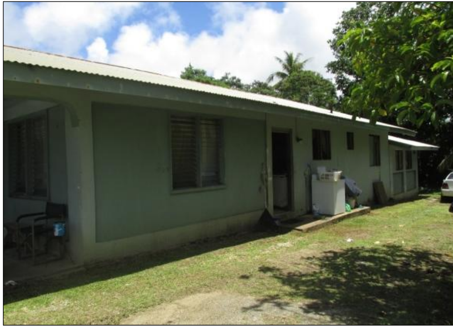
Figure 70. Property No. 21, Rabino House; facing west.
