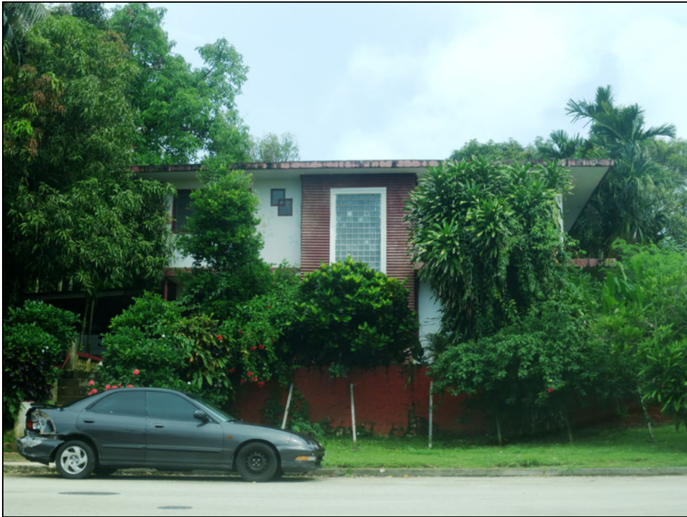
Figure 2. Herrera House, northwest elevation.
