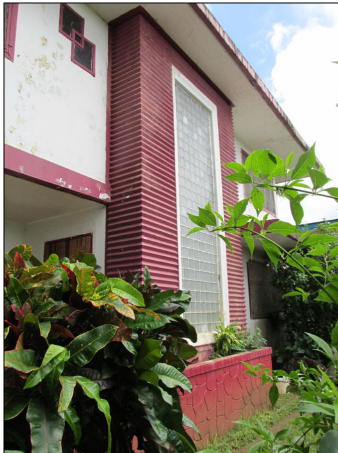
Figure 3. Herrera House with view of concrete pilaster.
