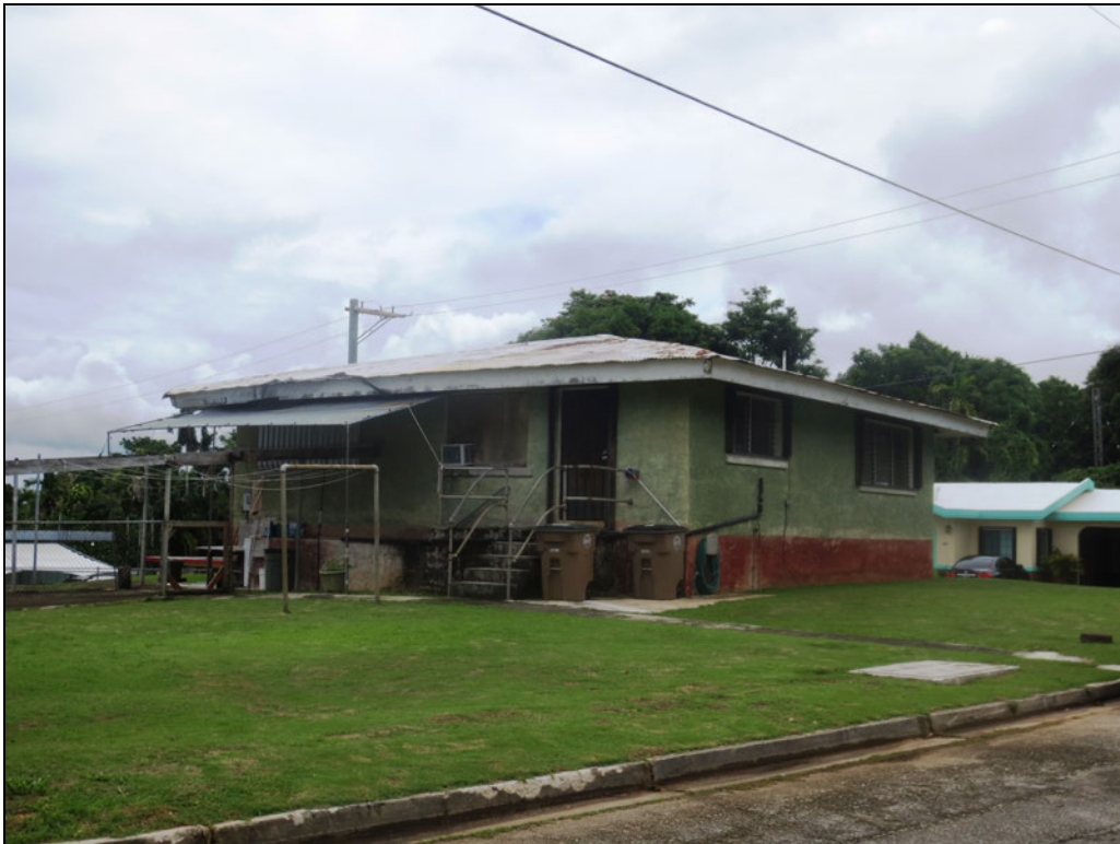
Figure 3. Hopkins House, south elevation.
