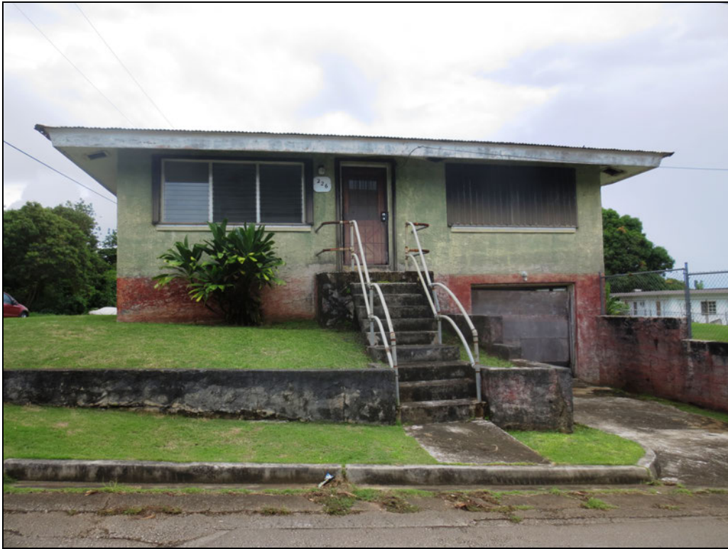
Figure 2. Hopkins House, north elevation.
