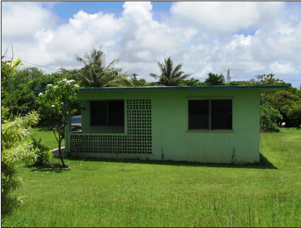
Figure 2. Mafnas House, east elevation.
