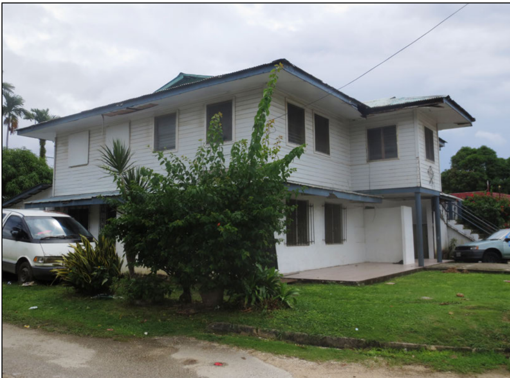
Figure 3. Sablan House, north and east elevation.
