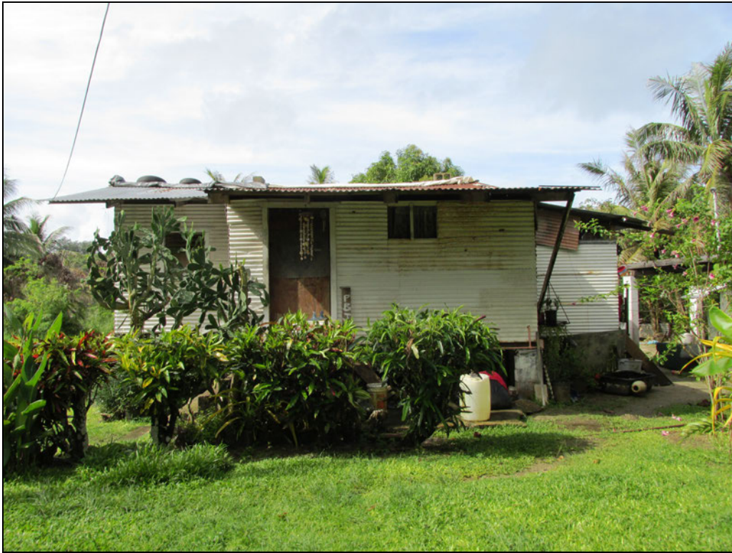
Figure 2. Sanchez House, east elevation.
