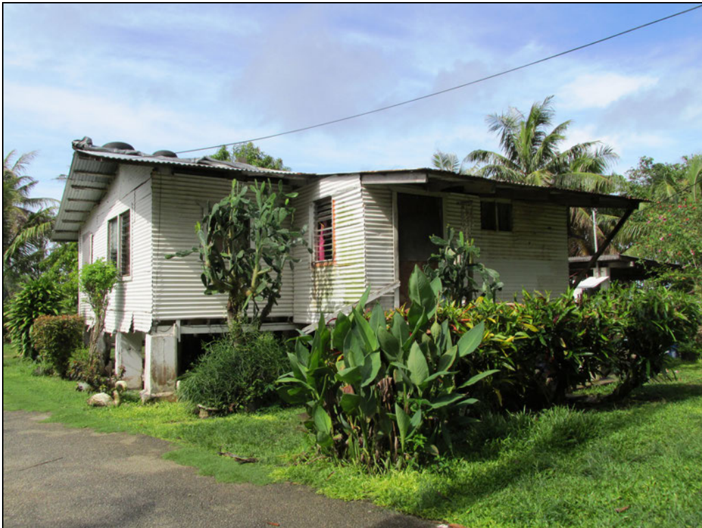
Figure 3. Sanchez House, north elevation.
