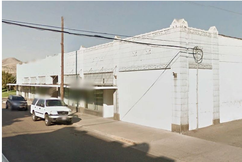
210 E. Center Street City Building and Shops
