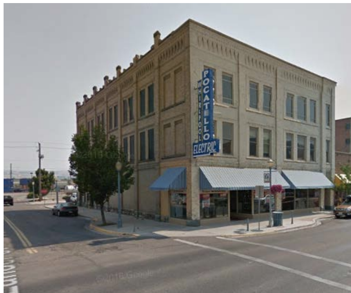
258 N. Main Street Masonic Building
