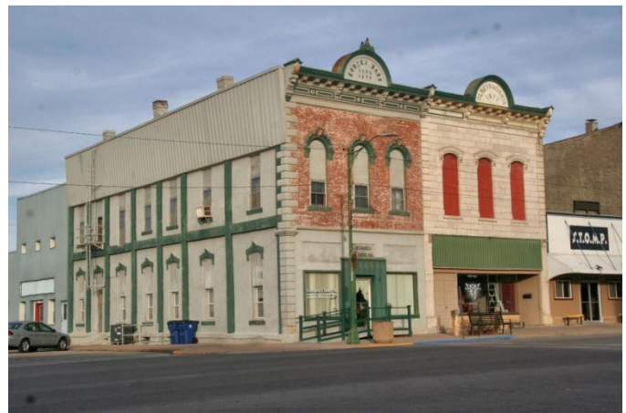
The Eureka Bank (1879) and Olney and Morris Drug Store (1877) buildings at 201-203 N. Main retain a high level of architectural integrity, both reflecting their original design and character (Spencer, 2018)
