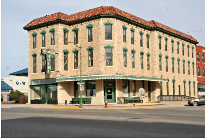
Greenwood Hotel, built 1884, expanded and remodeled in 1920s. Listed in National Register of Historic Places in 2005.
