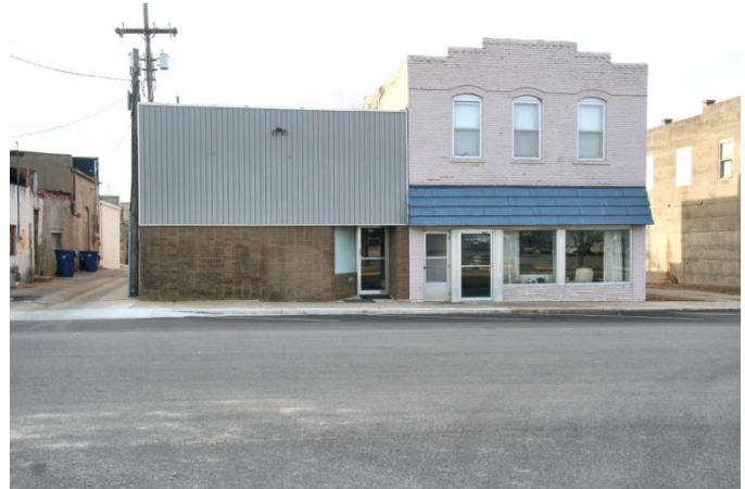
The building on the left above, located on W. Third Street originally had stamped metal siding which remains on the side and rear of the building. The existing siding covering the upper facade and the replacement storefront with minimal openings has drastically changed the historic character thereby rendering it a non-contributor to the proposed district.
