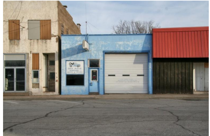
The former Hartsook Produce Co. building at 116 W. 2 nd is a one-story example of the Minimal Commercial style. This 1920s building has a mid-century replacement facade with no ornamentation and punched openings.
