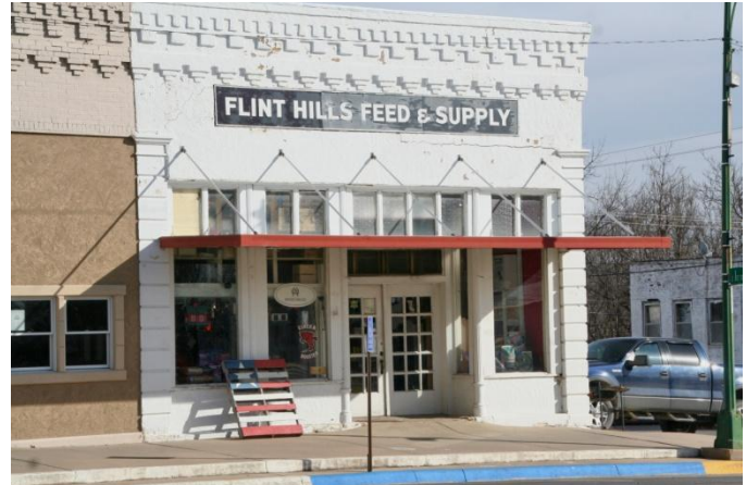
Hartsook Grain and Feed Building at 100 N. Main
