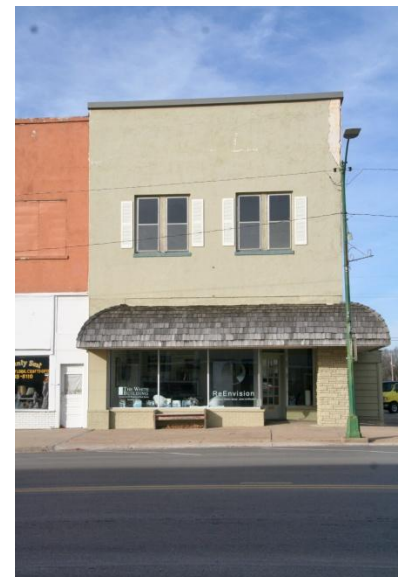
The White Building at 123 N. Main is an example of the Minimal Commercial style. Formerly a 3-story Italianate building, in 1948 the upper floor was removed, windows and storefront replaced, and stucco parging installed over the brick facade simplifying the details of the building.
