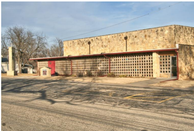
Built in 1966, Sacred Heart Catholic Church is among the younger historic resources in the survey area. Reflecting tenets of the Modern Movement, the church could be eligible for individual listing in the National Register.
