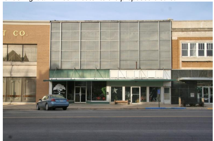
One of the most common mid-century alterations was installation of a metal slipcover on the upper facade and installation of a new aluminum-framed storefront. These types of alterations such as the slipcover seen above on a building in the 200 block of N. Main, have now gained significance in their own right. The building is now a contributor to the proposed historic district as a representative of the mid-century modernization (versus its original 1880s design).
