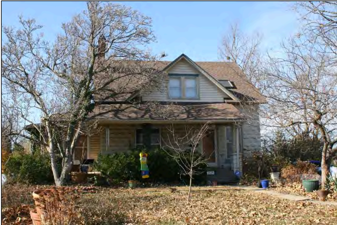
Figure 14. The 1929 Bernardo and Minnie Wegele residence at 2525 SW Western has textured concrete block cladding in the first story.
