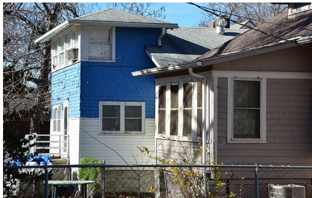
Figure 40. Raised sleeping porch at rear of 1719 SW 2nd Street, 2017.
