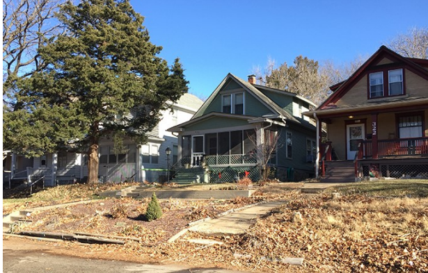
Figure 25. Single-family residences on SW Elmwood Avenue, 2017.
