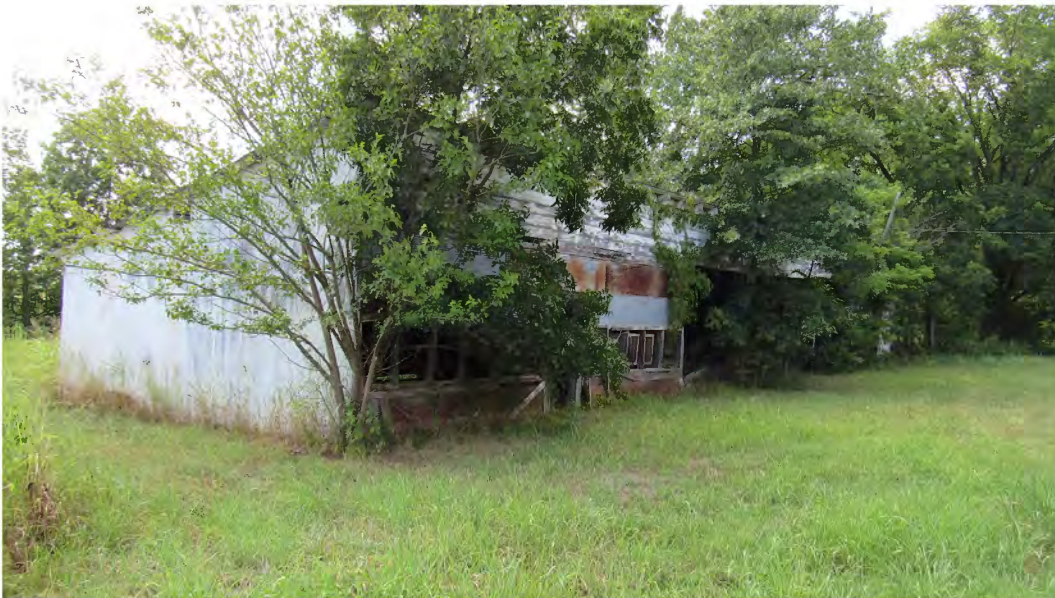
Figure 64. Wood machine shed, looking northwest.
