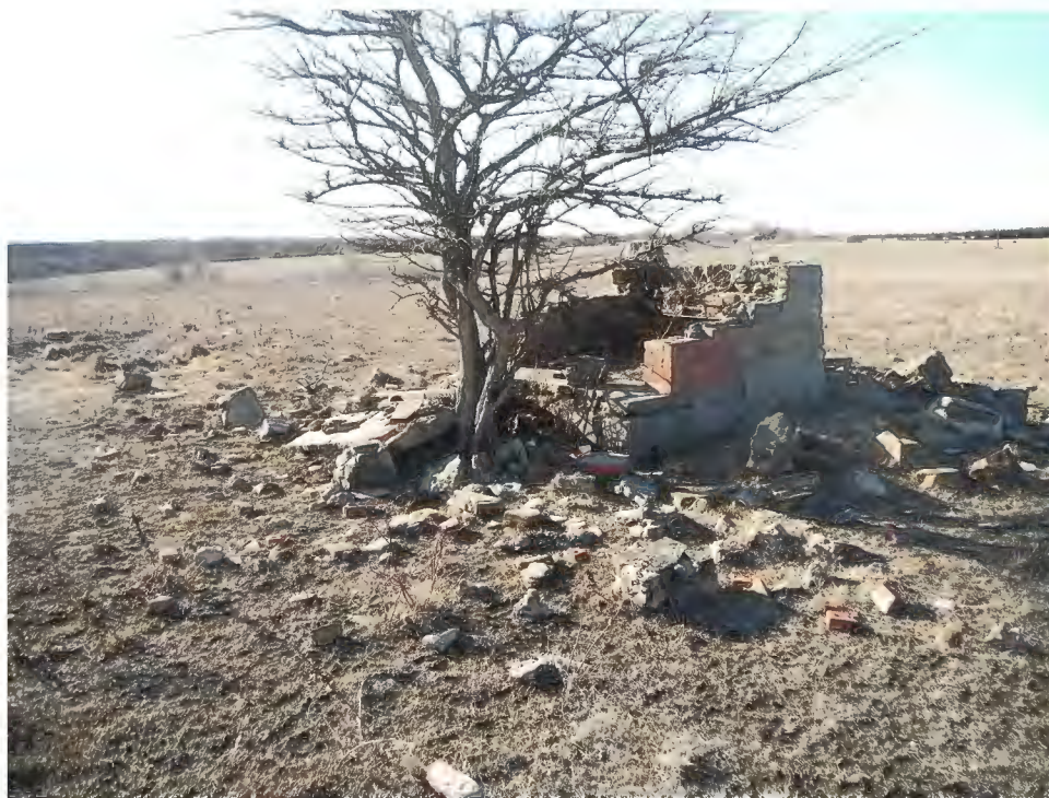
Figure 31. View northwest of brick, stone, and concrete fireplace ruin and associated footings of former education building (2012).
