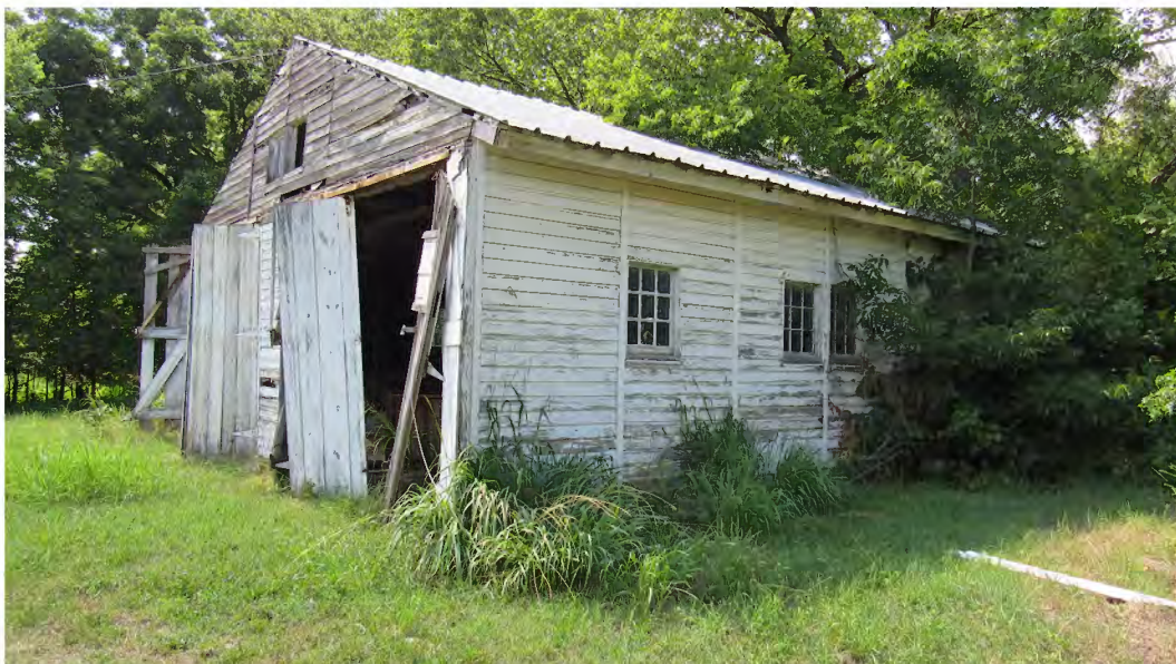
Figure 62. Wood shop building, looking northwest.
