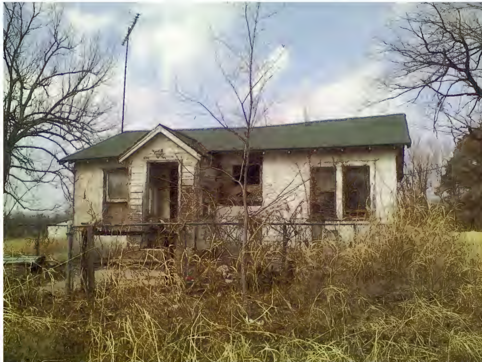
Figure 61. Former officers' quarters/American Legion post destroyed in a recent fire at the site (2009).
