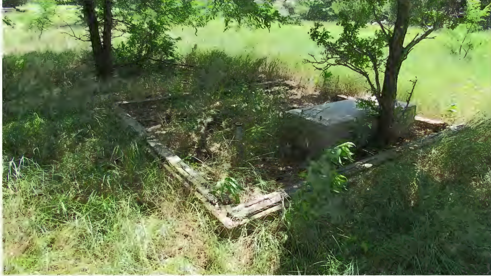
Figure 102. Location of the pump house and water tower footings in the northwest corner.
