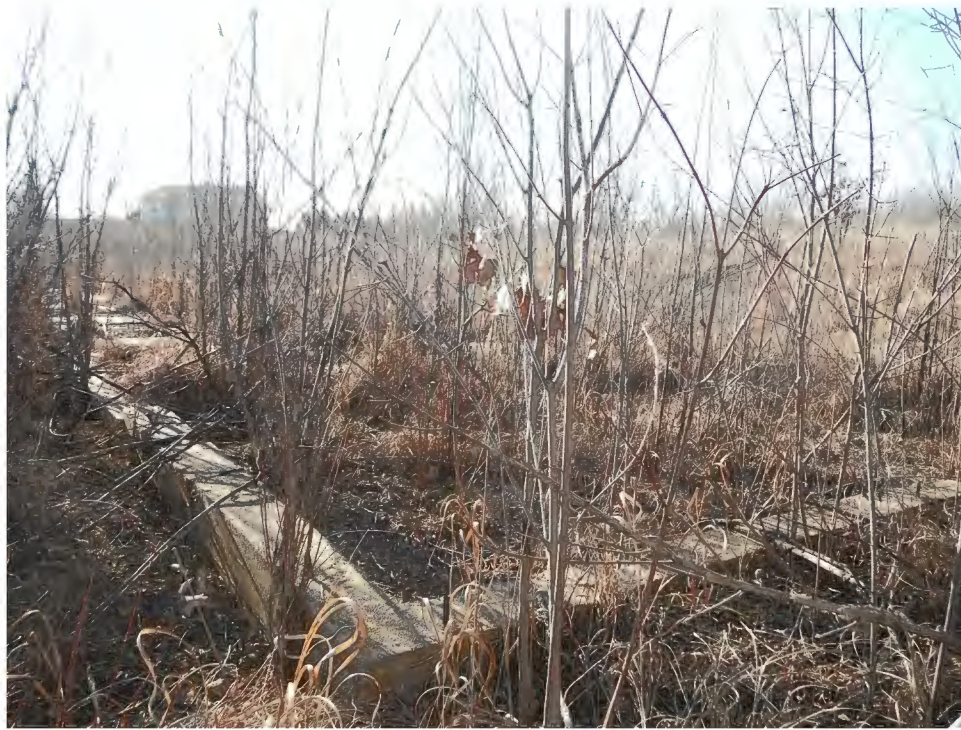
Figure 27. View west of concrete foundation and floor of bath house (2012).
