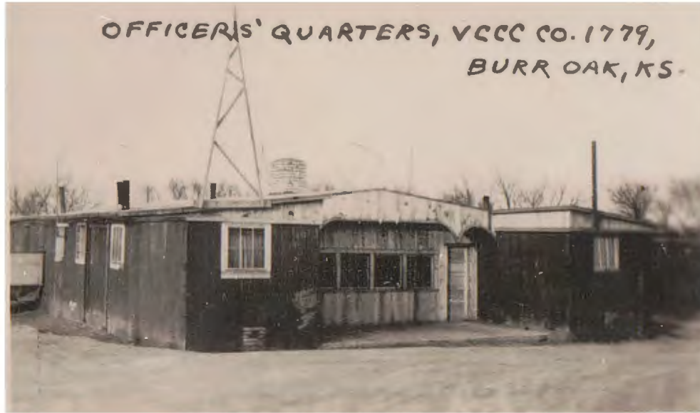
Figure 43. Period photograph of officers' quarters showing chimney feature(Crawford Co. Genealogical Society).
