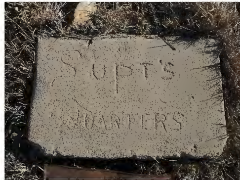
Figure 30. Concrete stoop inscribed “Supt’s Quarters” (2012).
