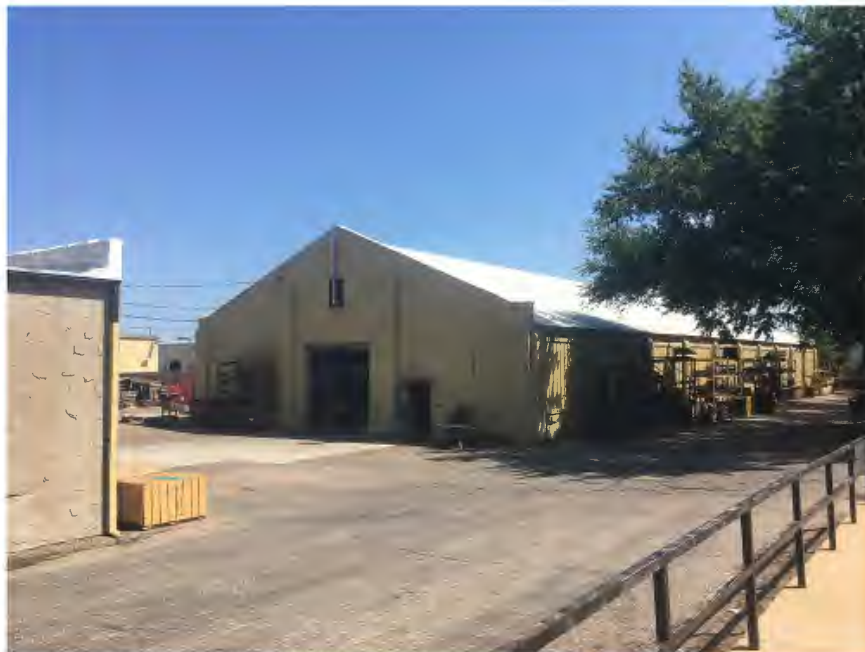
Figure 92. Faux stone cinderblock building, looking northeast.
