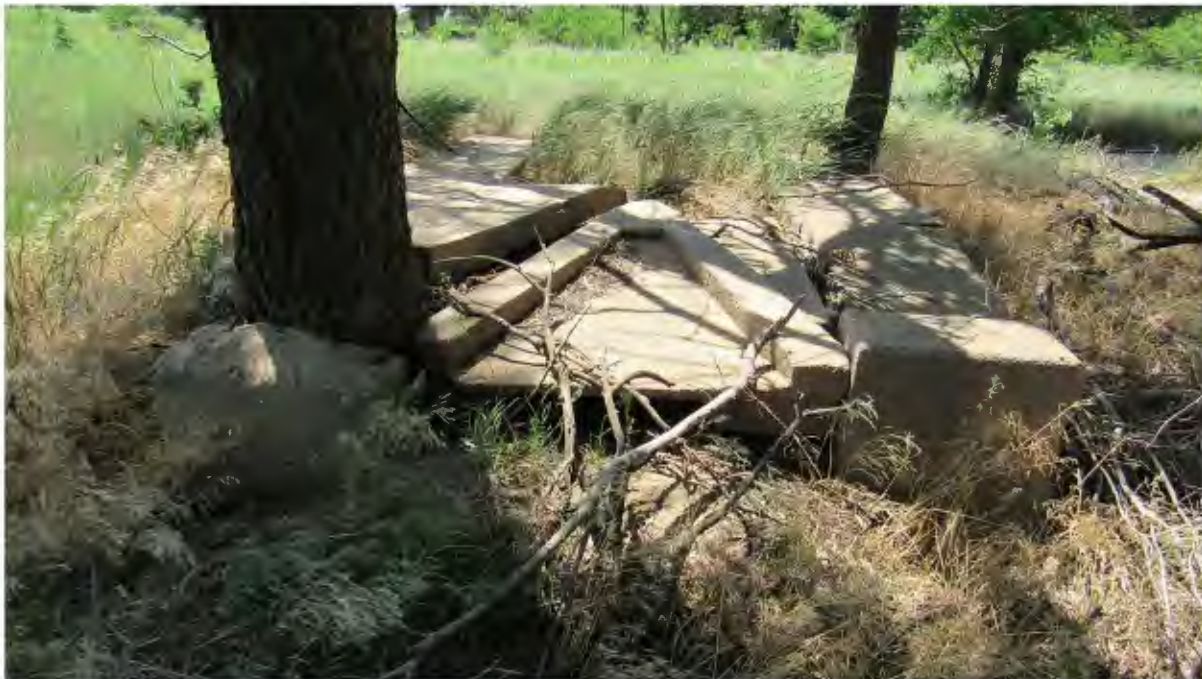
Figure 97. Concrete floor/foundation features including garage related ruins in a cluster along the east side of the site.
