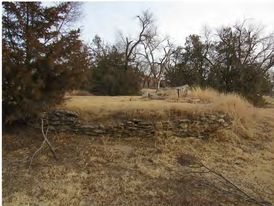
Figure 39. Dry laid stone retaining wall and earth fill flagpole platform (2017).
