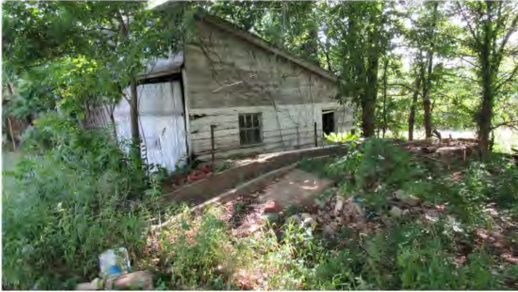
Figure 60. Concrete and limestone service rack located on north side of a maintenance building for the camp, looking southwest.
