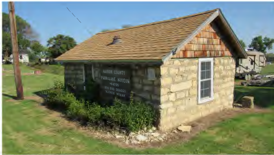
Figure 83. Small one-story mortared limestone structure. Looking southeast.
