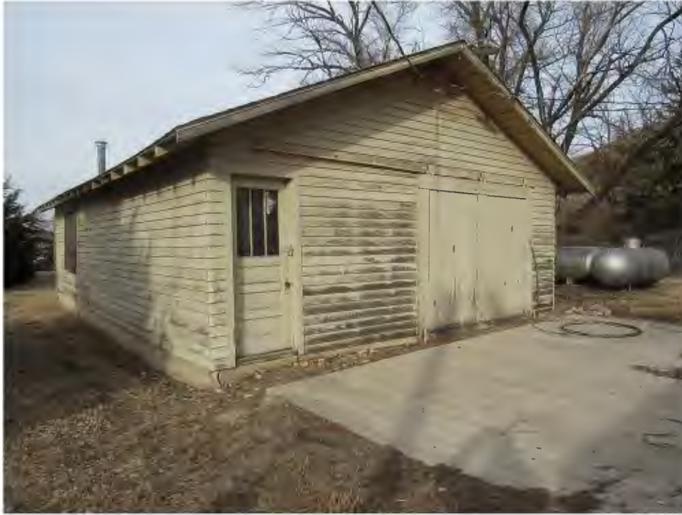
Figure 40. View northeast of wood frame utility building relocated to the present location from elsewhere in the camp (2017).
