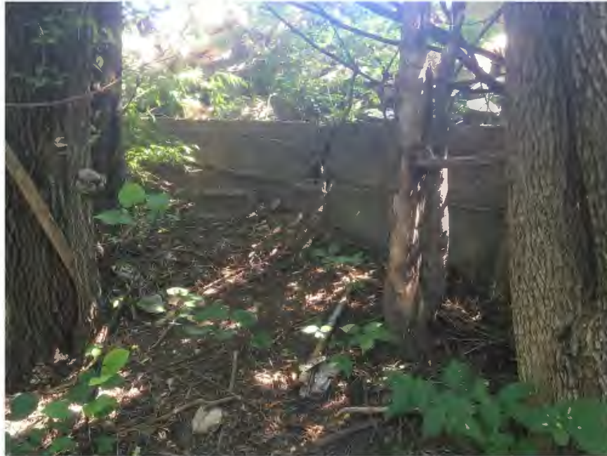
Figure 91. Concrete floor and foundation ruin on east boundary of Lions Park.
