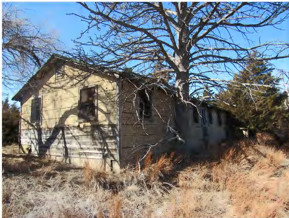
Figure 69. Former foremen's quarters, looking west (2017).
