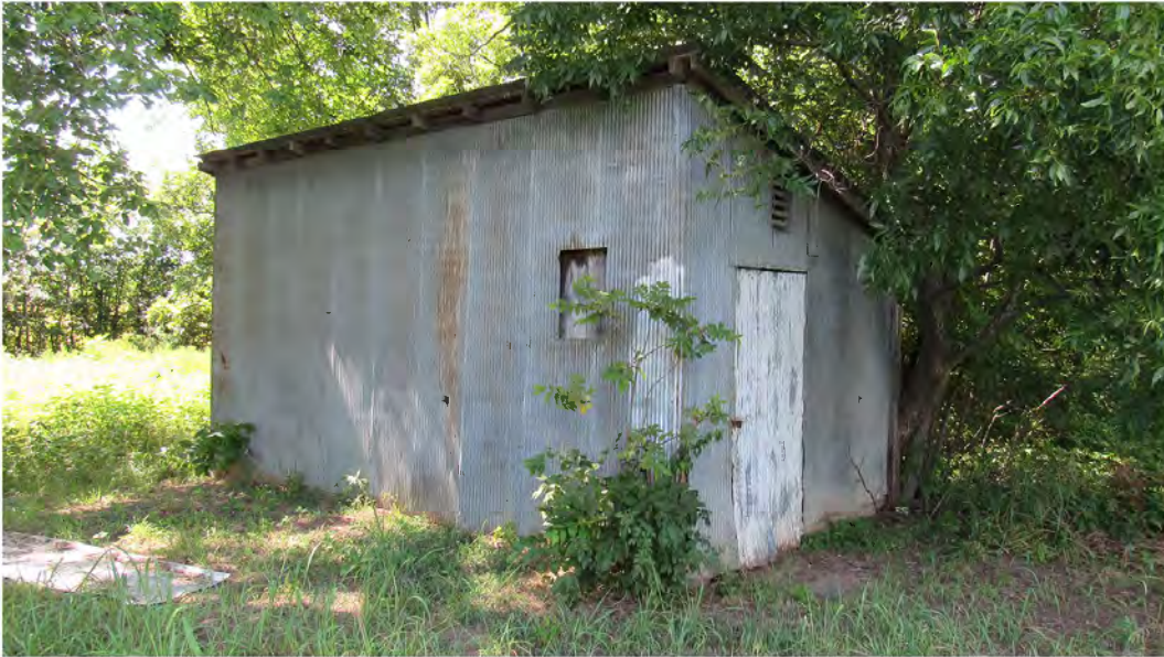
Figure 63. Small lean-to shed, looking northwest.
