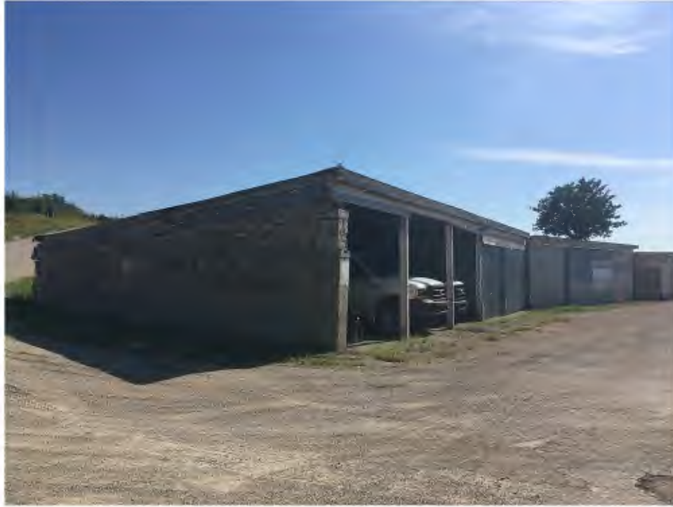
Figure 80. Vernacular stone machine shed, looking south.
