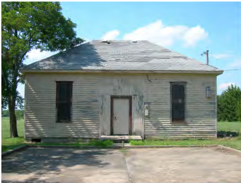
Figure 54. Frame building with adjoining concrete floor/foundation, facing north.
