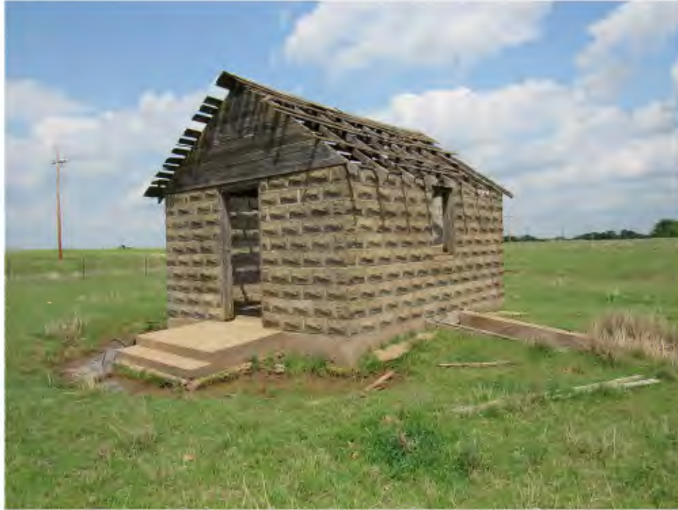
Figure 88. Faux stone cinderblock building, looking northeast.
