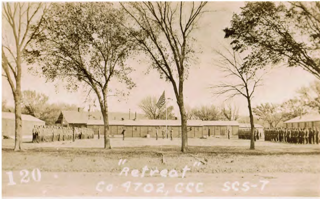
Figure 73. Camp John Redmond at retreat. Note roofline of railroad depot behind camp building in center of photo.
