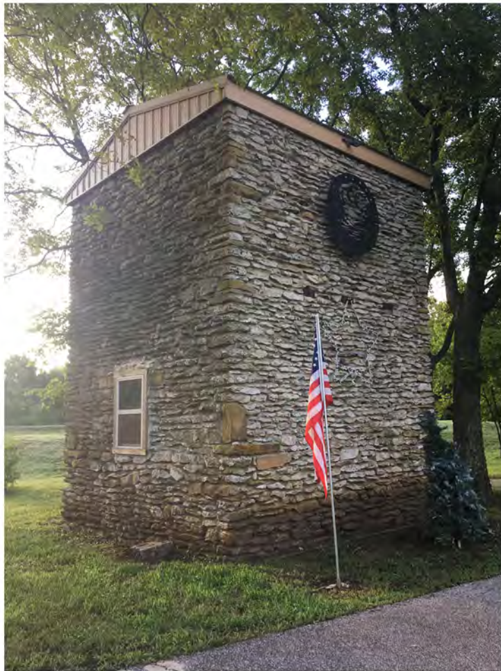
Figure 22. View southeast of mortared limestone water tower base.
