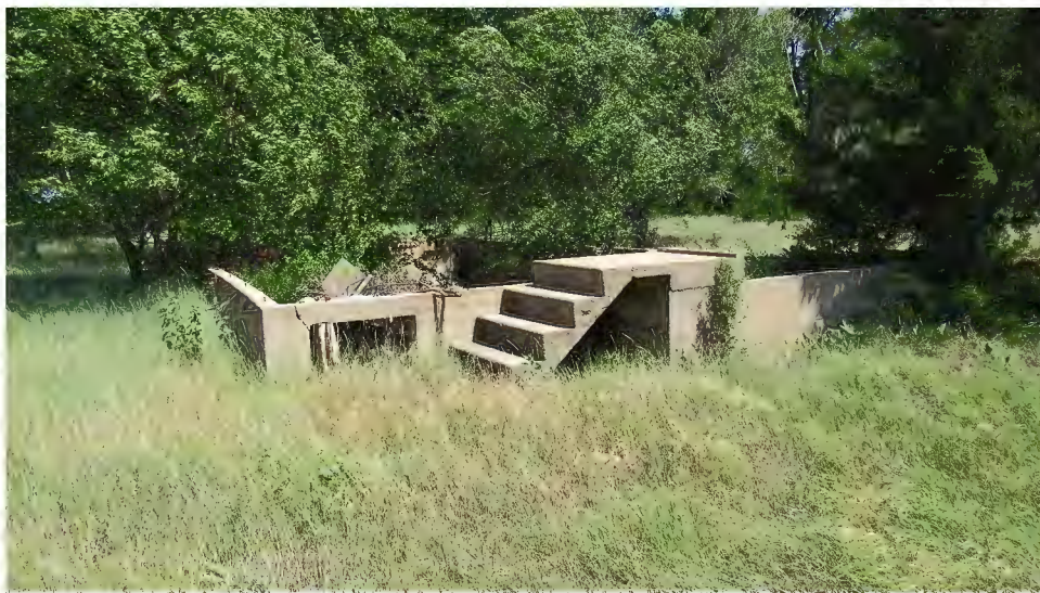
Figure 101. Concrete foundation and basement with stairways, likely location of leadership quarters.
