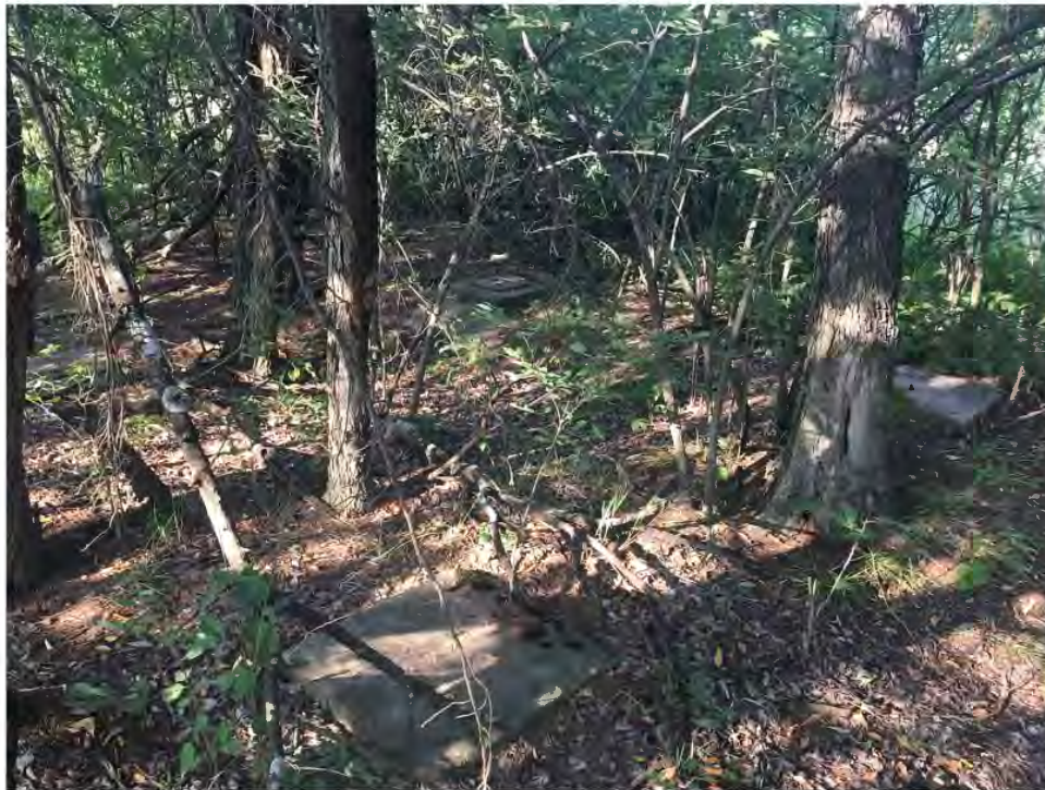
Figure 47. Concrete footings for water tower located in dense cover.
