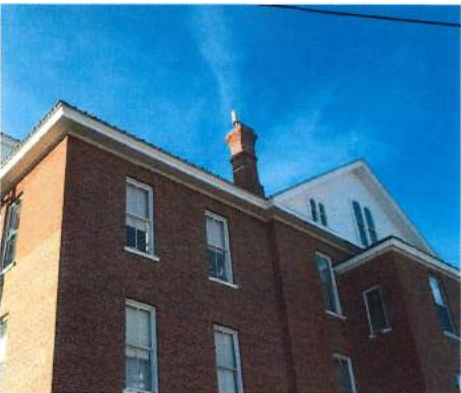
Photo 2- East Gable and Chimney
