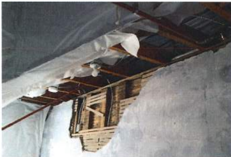
Photo 23 - Attic wall showing plaster over wood stud framing; Ceiling joists above
