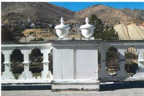
Photo 10 - Existing 3rd Floor Porch Railing Detail
