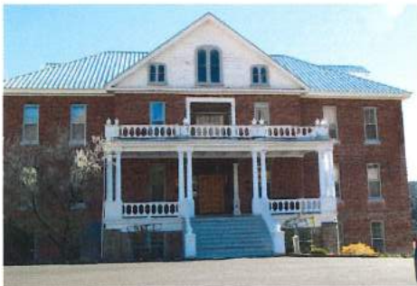
Photo 20 - Main Stairs on West (front) Elevation
