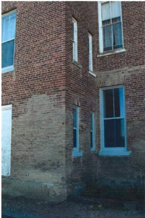
Photo 18 - East elevation showing parge coat on first story brick
