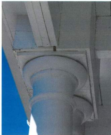
Photo 6 - Existing Column and Beam Framing 3rd Floor Porch
