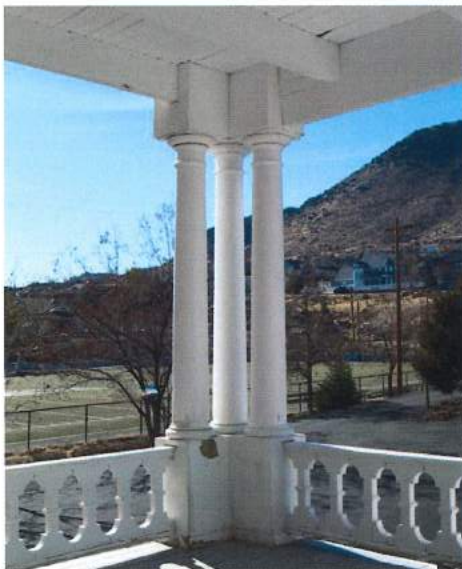
Photo 14 - Second Floor Porch Columns, Railing and Ceiling
