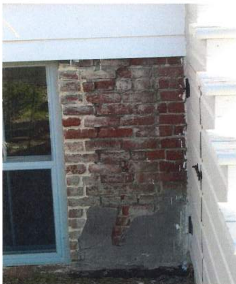
Photo 19 - West Elevation, north of main stairs
