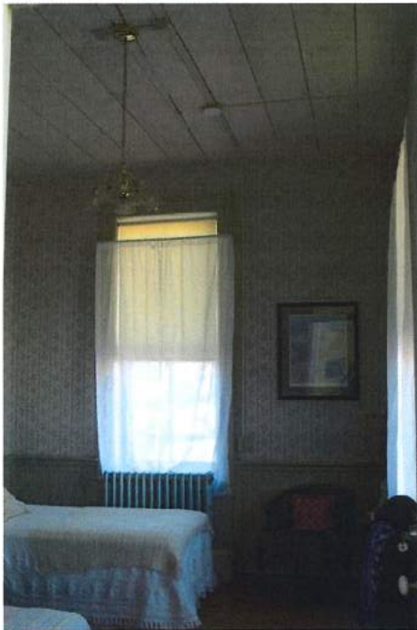
Photo 31 - 2nd Floor Bedroom showing exposed 1x deck boards as the ceiling finish.
