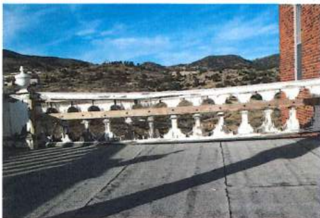
Photo 9 - Existing 3rd Floor Porch Railing
