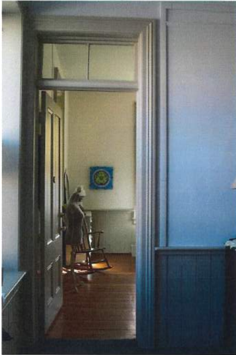
Photo 29 - 2nd Floor Hallway showing chair rail and high rail looking into a bedroom
