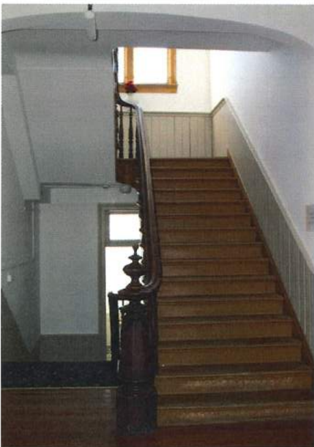
Photo 25 - Main Stair Interior, 2nd Floor Landing
