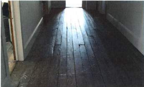
Photo 27 - 4th Floor (Attic) Floor
