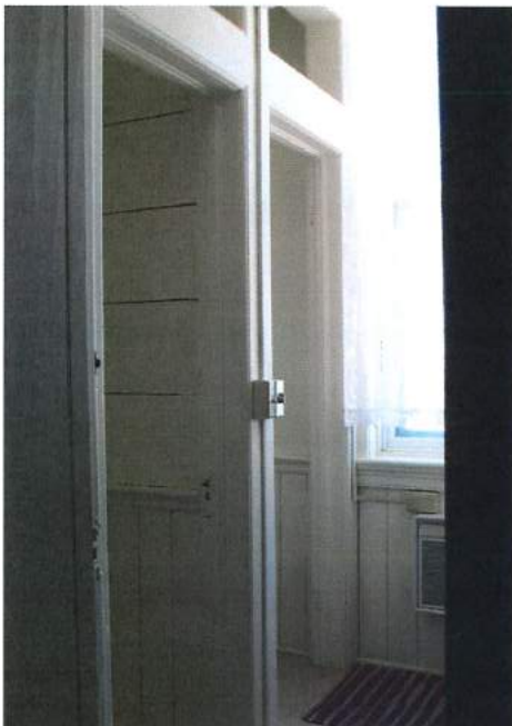
Photo 26 - Toilet Room showing separate water closet stalls.
