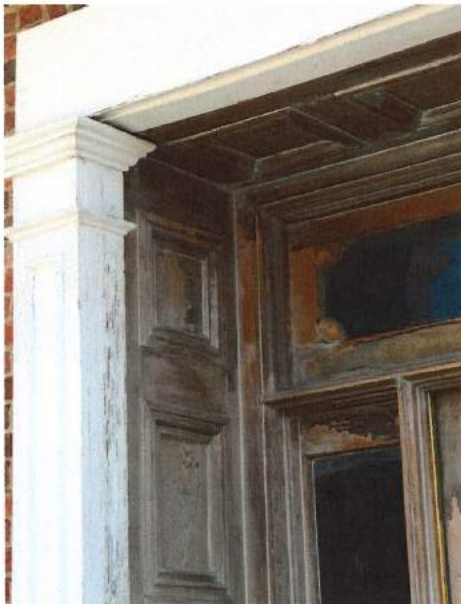
Photo 11 - Existing 3rd Floor Porch Door Corner Detail
