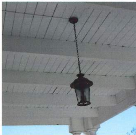
Photo 7 - 2nd Floor Porch Ceiling
