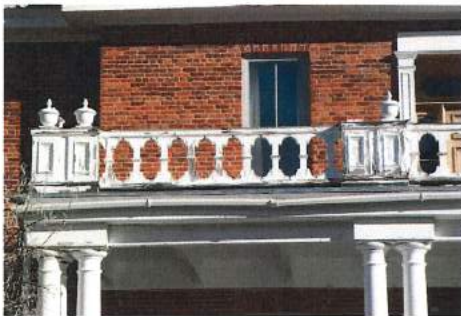
Photo 8 - Existing 3rd Floor Porch Railing
