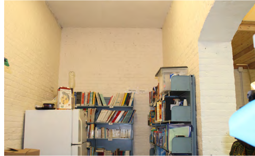
Photo 110: Room 008, looking west
