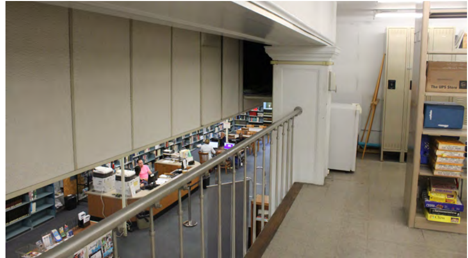
Photo 62: The steel balustrade with original square columns The stairs to the second floor with marble balustrade
