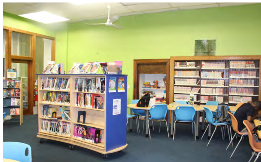
Photo 22: The wood enclosure to the left is an original dumb waiter used to move books
