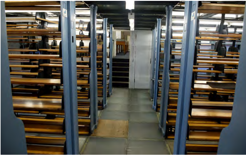
Photograph #5 – Cracked Glass Floor Pane and Plywood Panel
