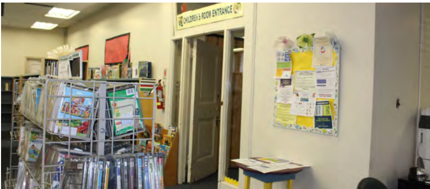
Photo 117: An original door and transom remain
