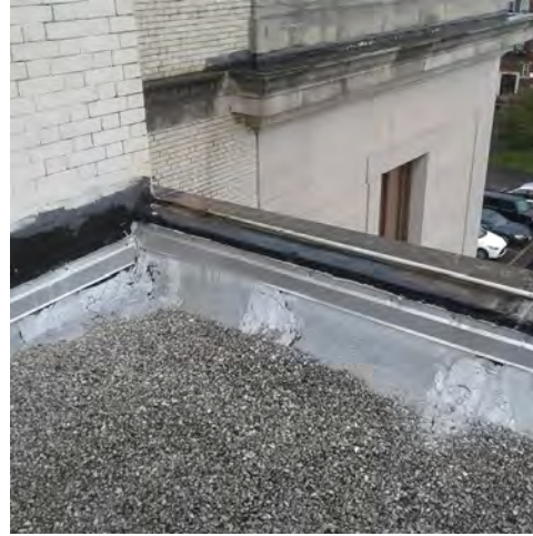
P98: Typical roof conditions.
