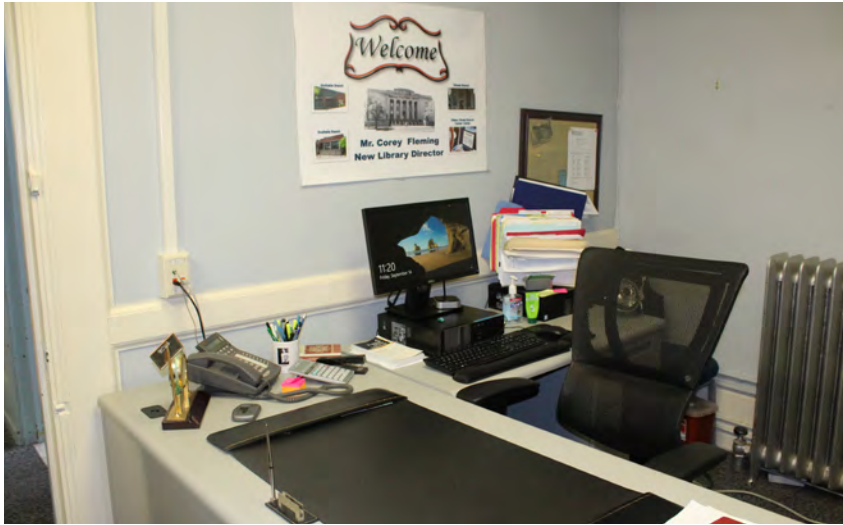
Photo 87: NE corner, Room 210. The chair rail is original
