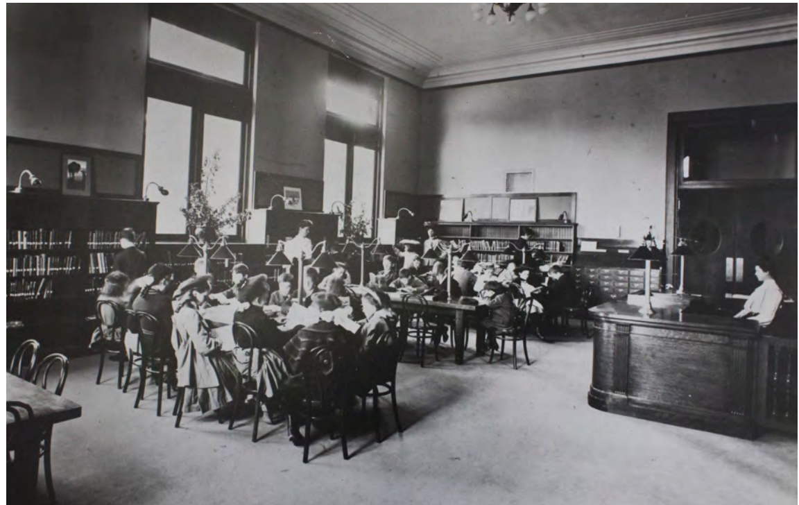
Figure 12: The children's room was originally located in the northeast corner, today's technical services room
