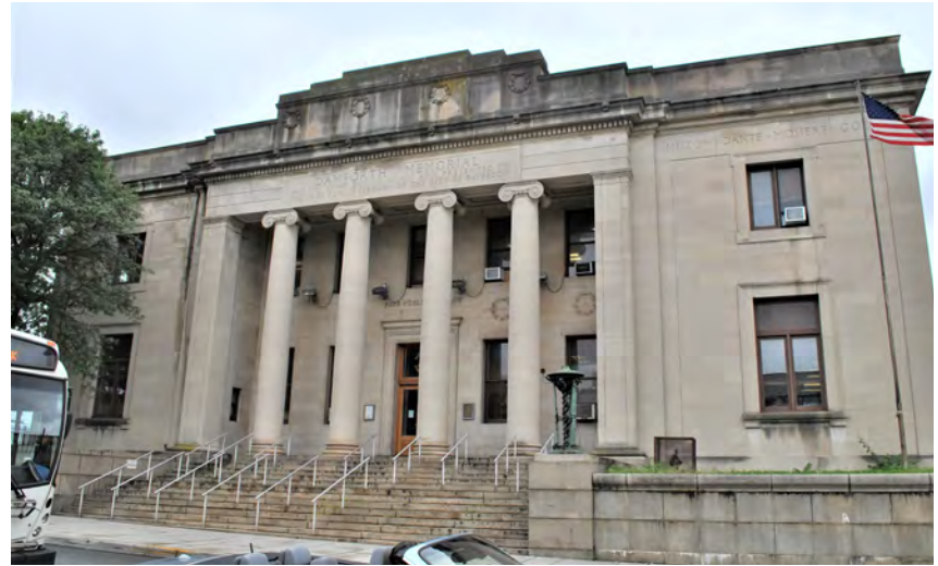
Main Entry from Broadway - North Elevation
