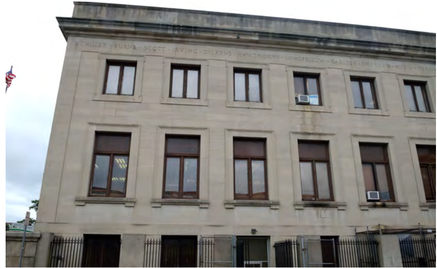
Photograph #6 – Limestone Cladding Typical Condition
