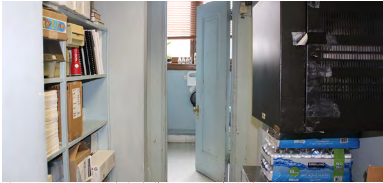
Photo 82: Room 209 includes halls, storage and a bathroom
