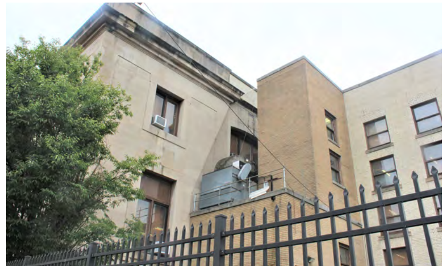
Rear Elevation Showing the Stair Addition
