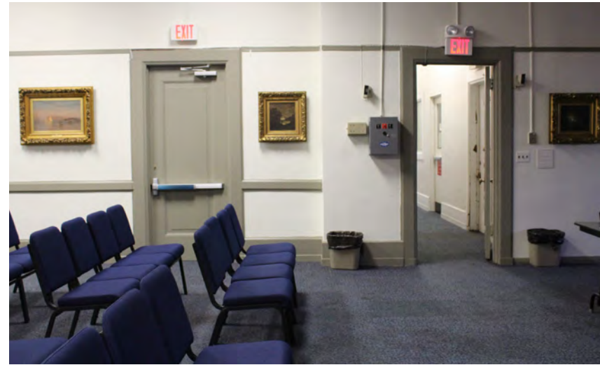
Photo 75: The chair rail and tall baseboard survive where the original assembly room existed. The short baseboards and no chair rail are in the location of the original cataloging room, to the east of the door
