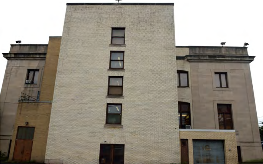
Photograph #7 – Brick Cladding Typical Condition
