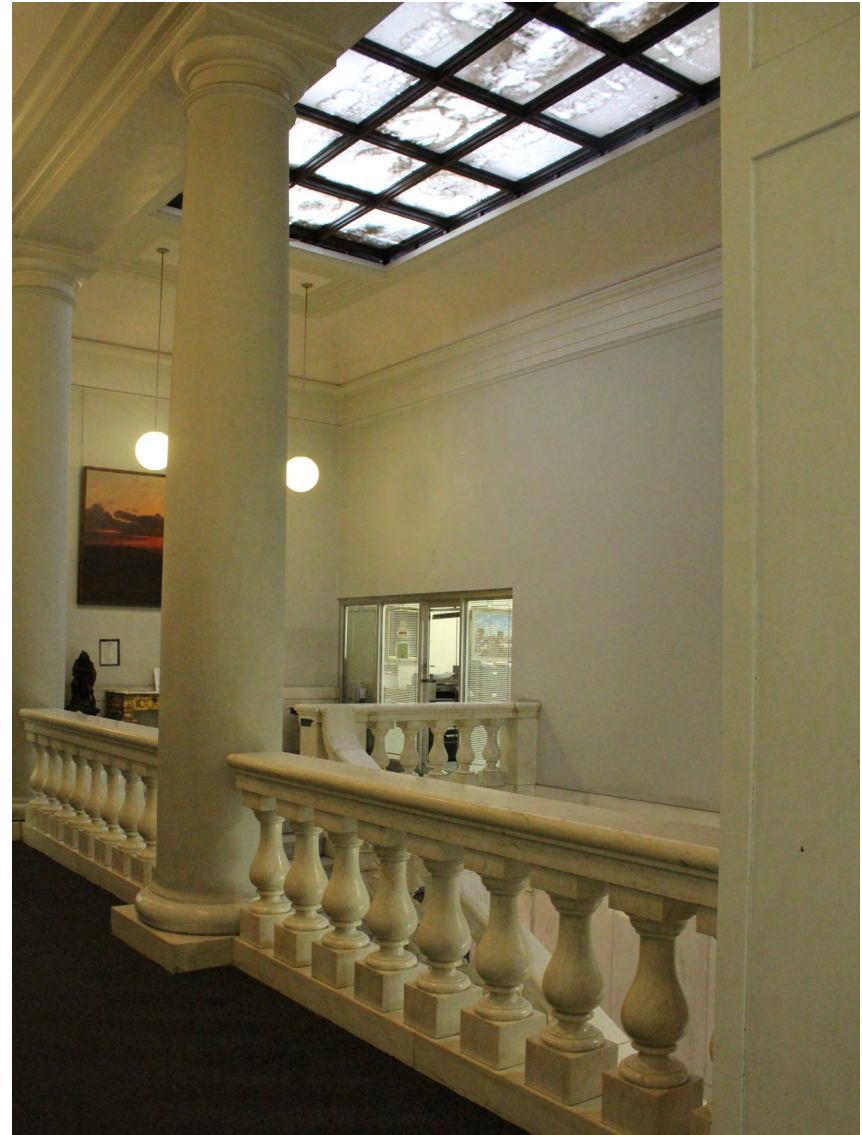
Photo 44: Original marble balustrade, plaster columns and laylights make this a grand space
