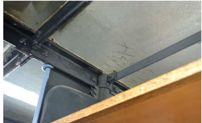
Photograph #4 – Library Stack Structure
