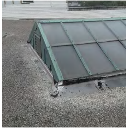
P122: Existing skylight over the main entry hall and stairs; blocked from below.
