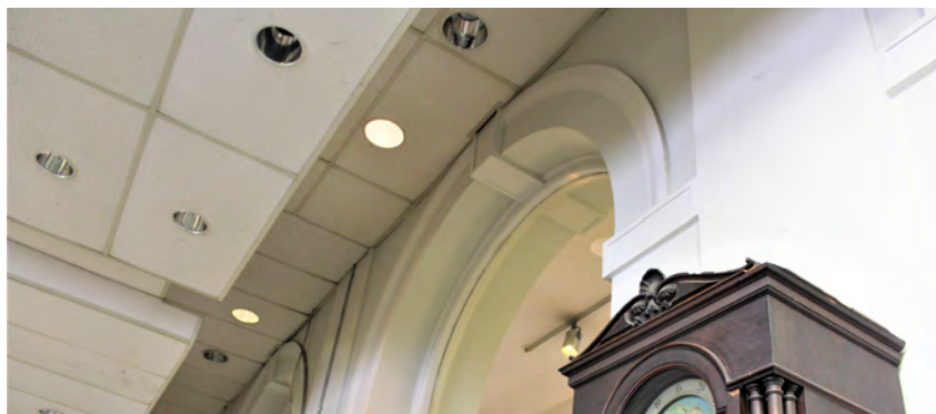
Photo 12: The drop ceilings obscure much of the original architectural details
