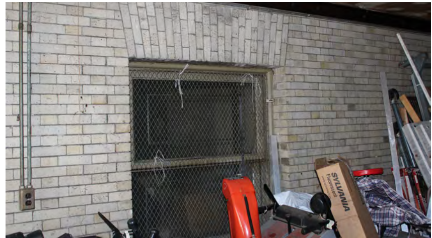
Photo 126: This is likely an original window
