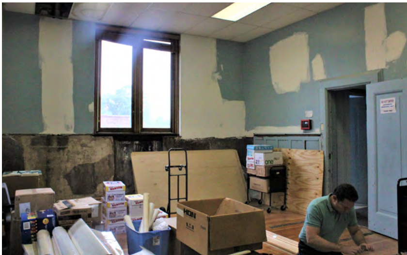
Photo 76: Room 208 is under construction
