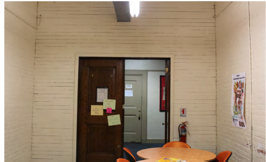
Photo 106: Room 005, looking south to the hall
