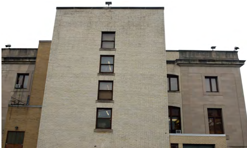
South Elevation Facing South and Van Houten Street
