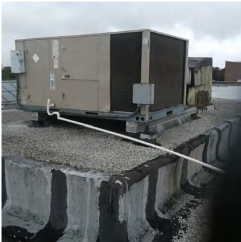
Pro6: Rooftop equipment.
