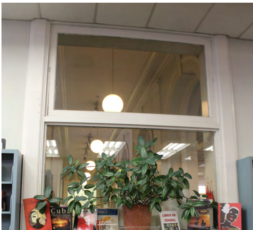
Photo 14: This interior window is original. It was originally at the end of the corridor but now divides circulation spaces
