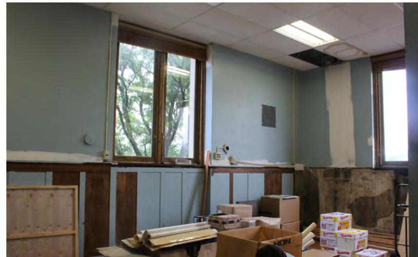
Photo 77: It retains original wainscot. Some of the paint has been removed
