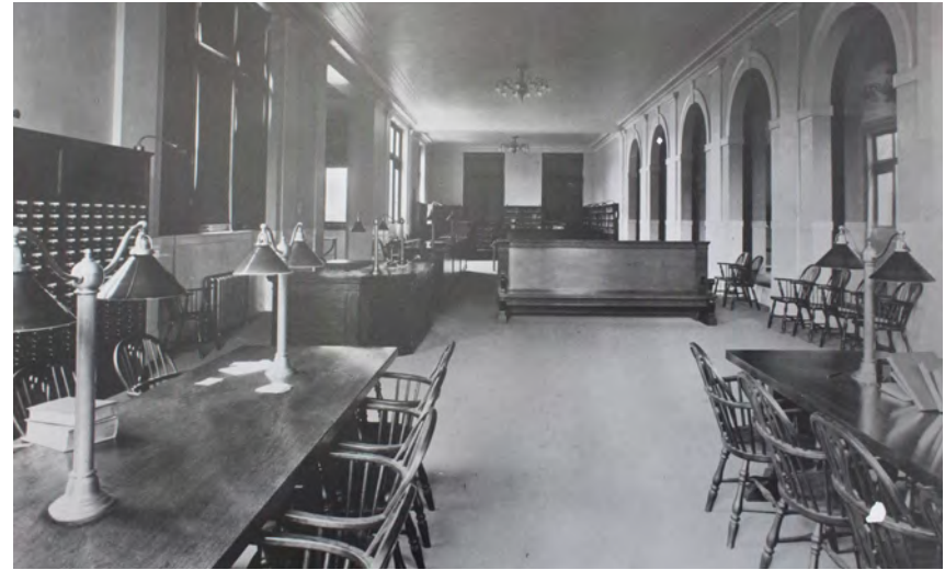
Figure 14: Today's circulation room (looking west) was originally called the delivery room and card catalogue
