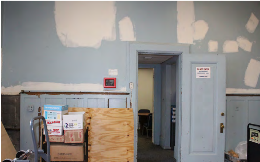
Photo 78: The doors and door surrounds are original
