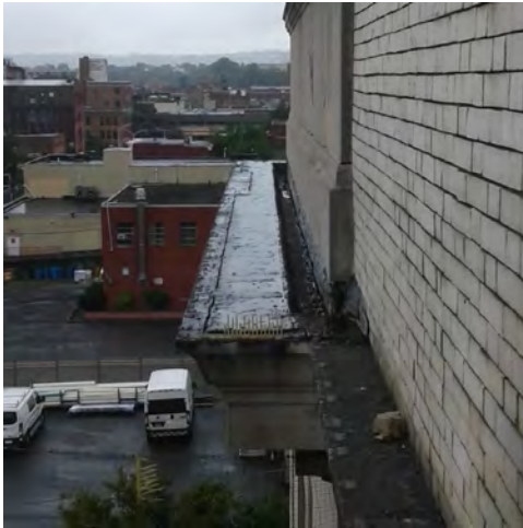
Pro3: View of top of cornice at SW corner.
