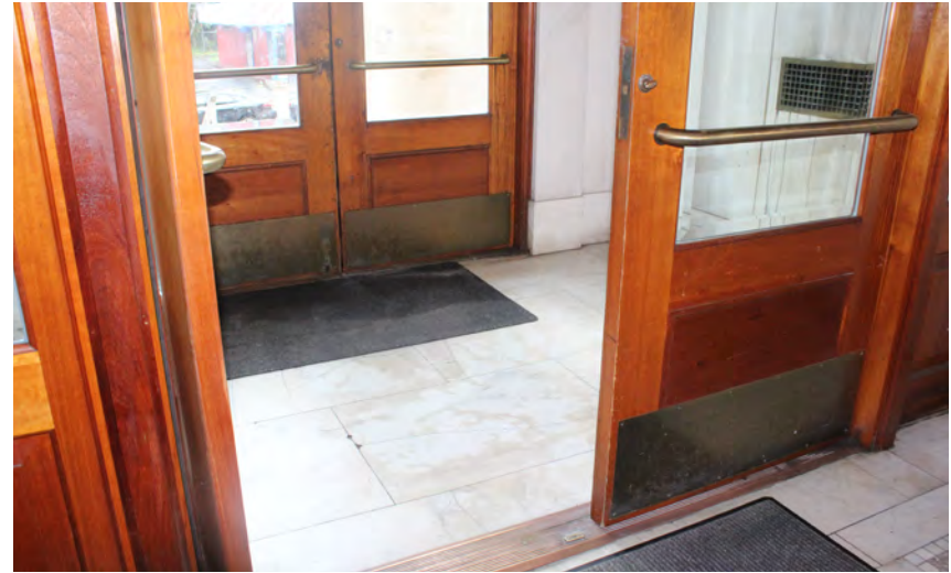
Photo 2: The original marble flooring remains. It has some cracking but generally is in good condition
