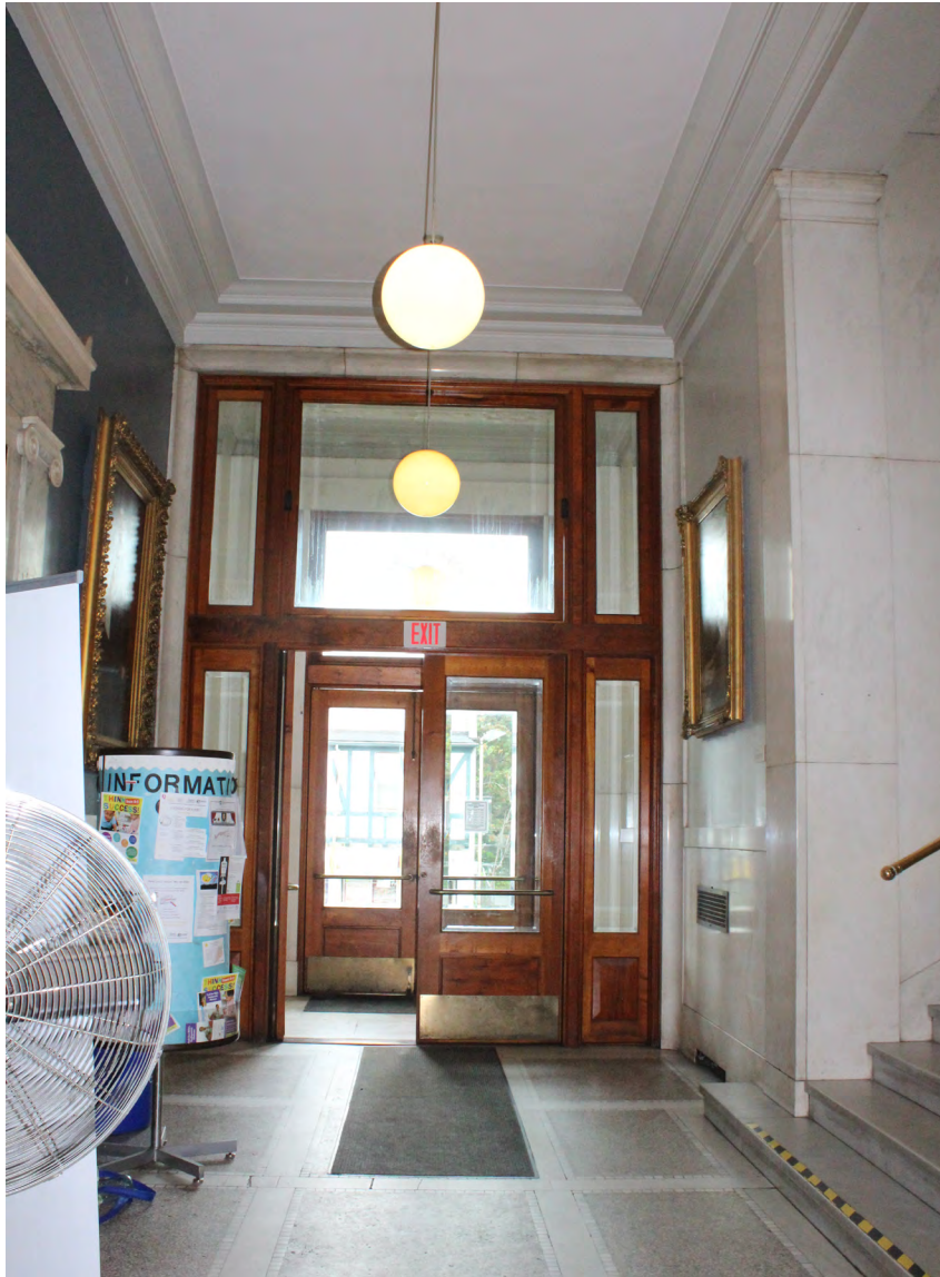
Photo 1: The wood and glass entry doors, sidelights and transom date to 2007. They are in good condition
