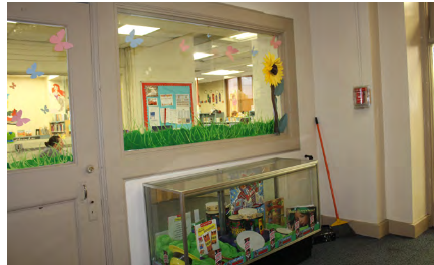
Photo 104: The door to the children's department, 005, has glass in the upper panel and an interior window
