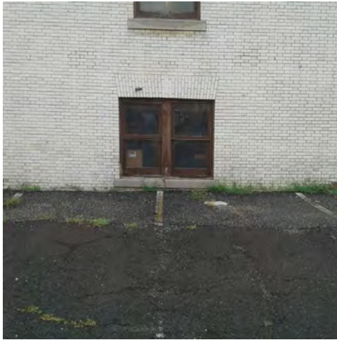
P91: Previous entry removed, S elevation, center of the rear wing.
