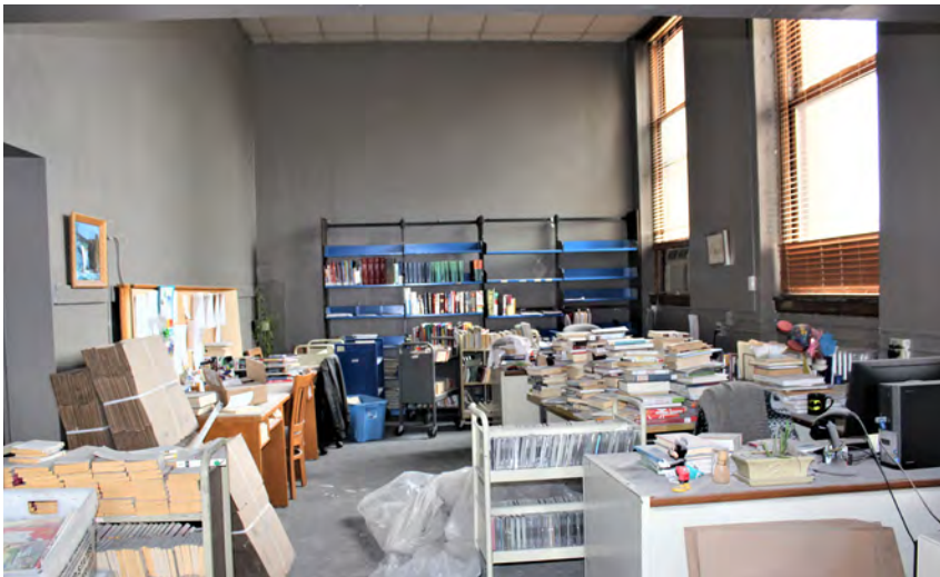
Photo 37: The room to the west. The hung ceiling remains in place
