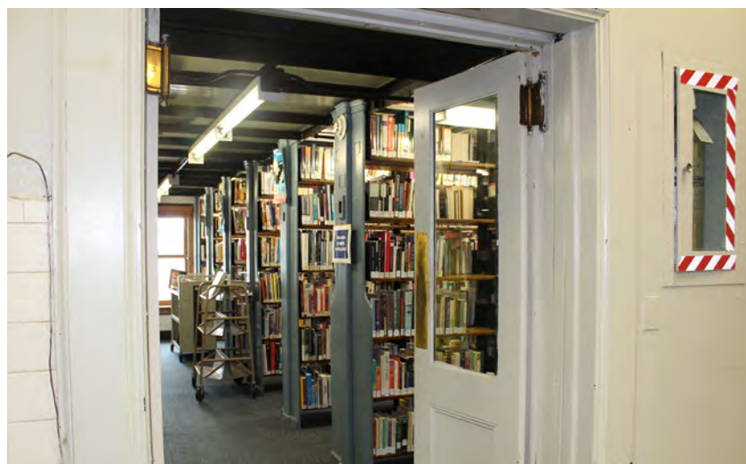
Photo 26: The original doors remain in situ
