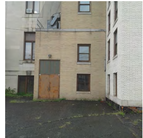
P96: Egress stair addition on the W side of the rear addition.
