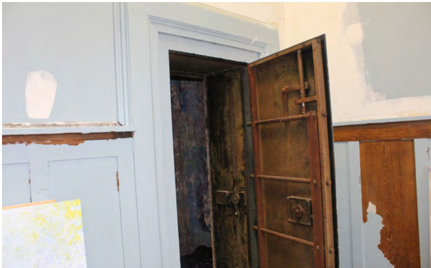
Photo 80: There is an original safe in the NW corner
