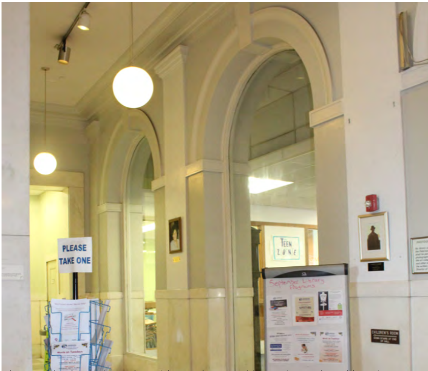
Photo 6: The decorative arches with run plaster moldings, piers and marble wainscot are intact and an important character defining feature of the library
