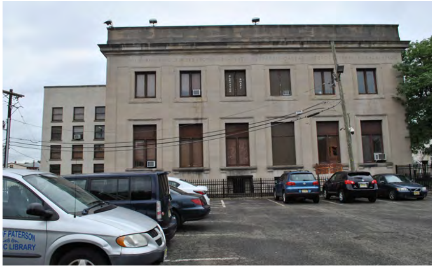
East Elevation facing Summer Street
