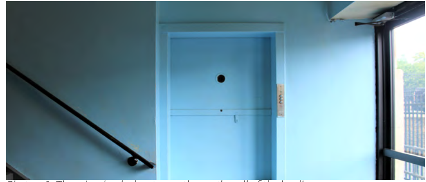
Photo 96: There is a book elevator on the north wall of the landing
