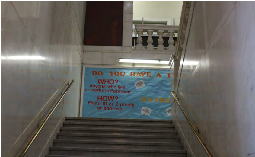
Photo 39: The stairs going up are remarkably intact
