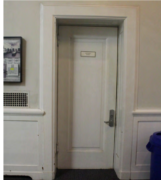
Photo 48: An original door and surround leading to 207. Originally the finish on both was clear as was the wainscot. Restoration of the finishes of this space should be a long term.
