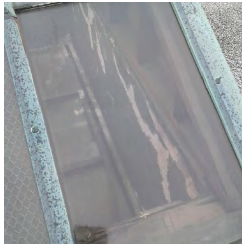
P125: Replacement glass in the skylight.
