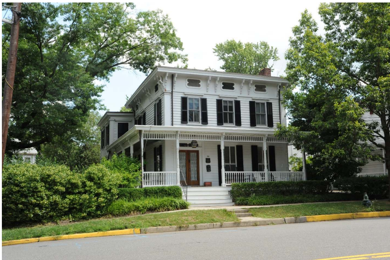
Plate 3-3: 39 S. Main Street, looking east.
