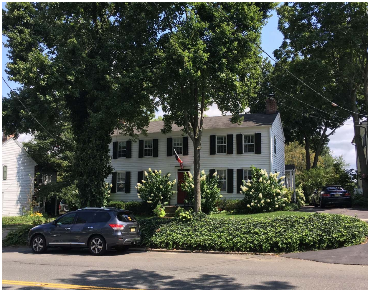
Plate 3-2: 45 S. Main Street, looking east.
