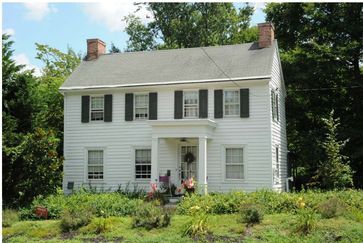
Plate 3-1: 43 S. Main Street, looking east.
