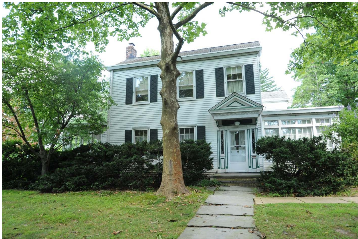
Plate 3-9: 1 S. Main, looking east.
