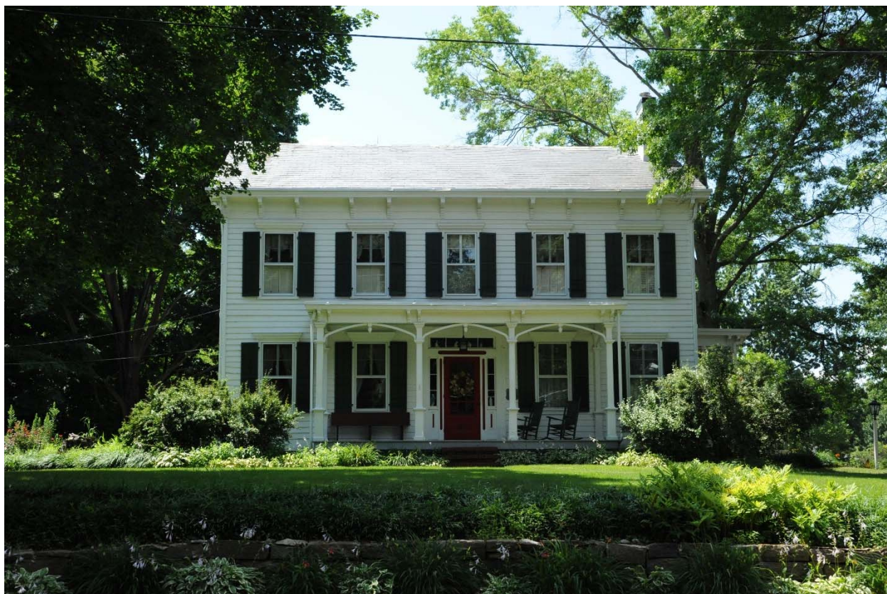
Plate 3-4: 40 Station Road, looking south.
