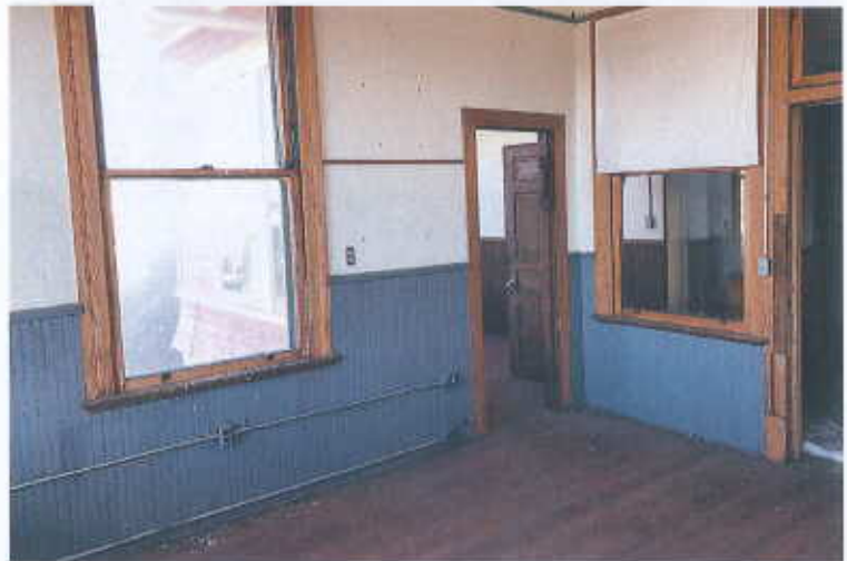
211. Room 206, historic woodwork (floor, wainscoting, 1/1 wood windows, interior door frame and transom).
