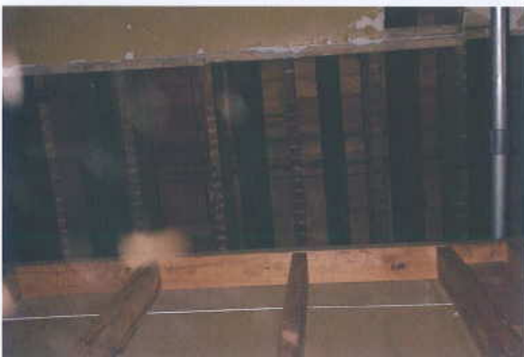
109. Room 102, original ceiling height is above the current finished ceiling.
