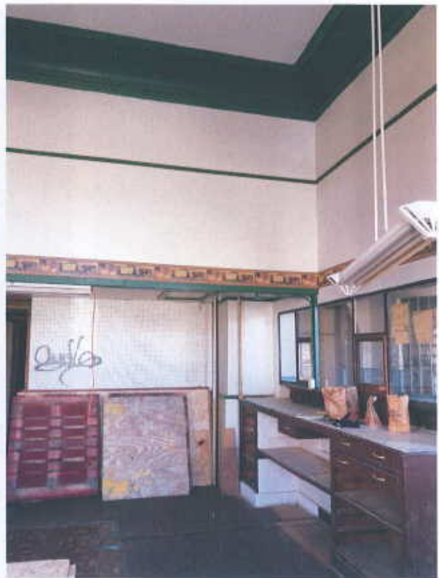
120. Room 103, non-historic ticket counter.
