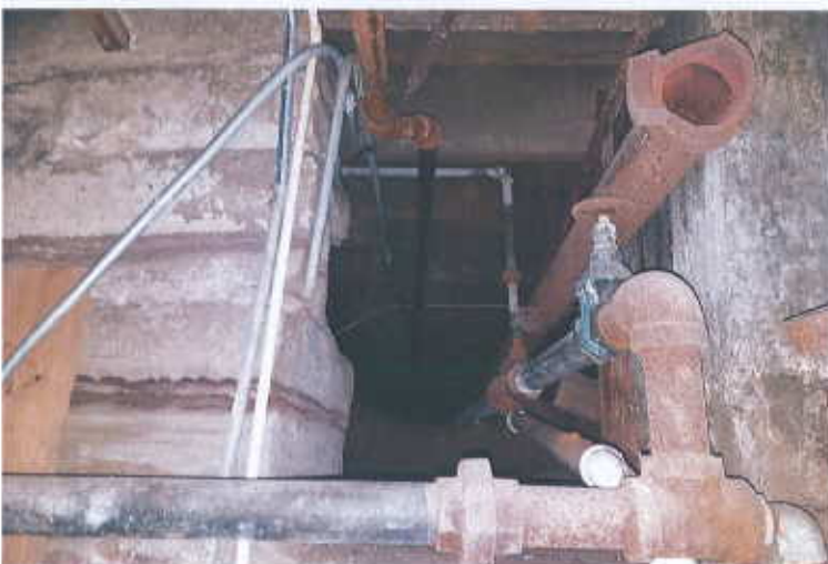
403. Basement, looking south.
