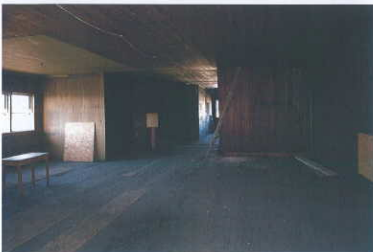
303. Attic, beadboard ceiling and walls, wood tongue and groove flooring.
