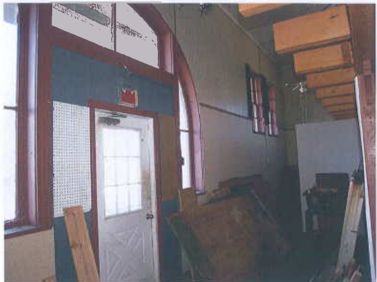
124. Room 106, infilled original arched door opening.
