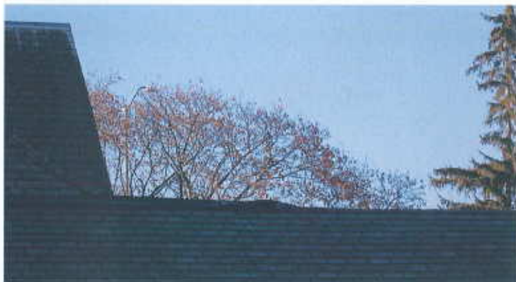
8. Bent ridge at canopy roof, east elevation.
