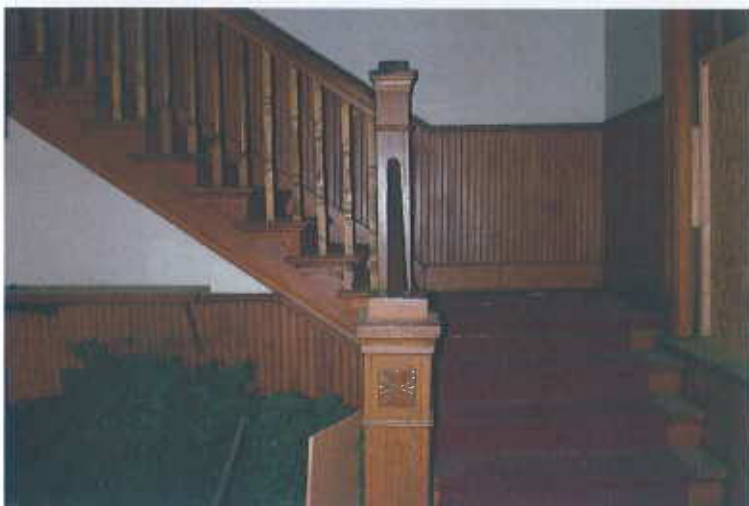
103. Room 107, historic staircase and wainscoting.
