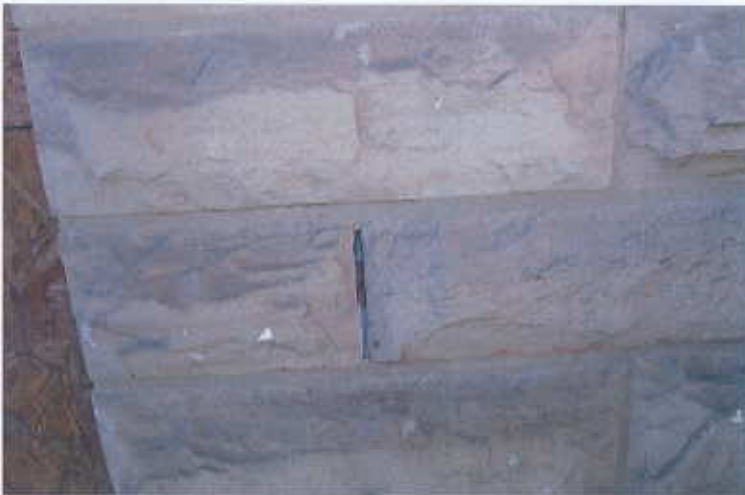
14. Detail, east elevation. Open masonry joint.
