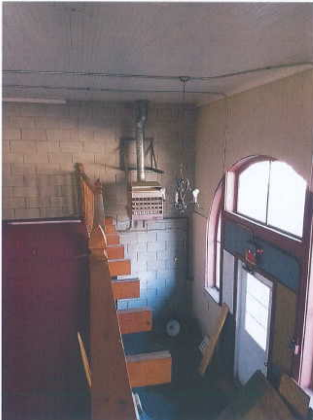
126. Room 106, infilled original arched door opening.
