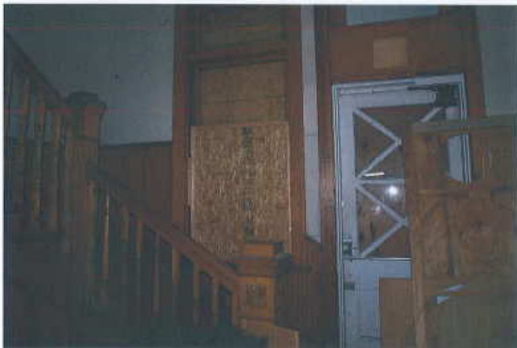
102. Room 107, boarded door and window, and historic staircase.
