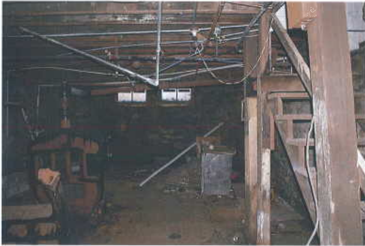
401. Basement, looking west.
