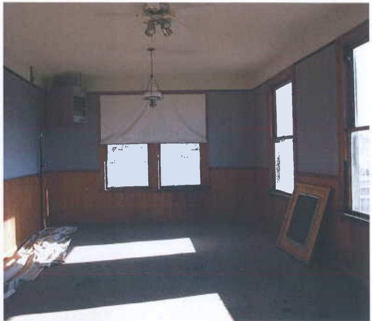
202. Room 201, historic 1/1 wood windows and wainscoting.
