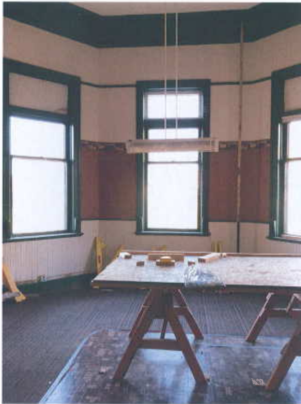
119. Room 103, historic wood base, wainscoting, trim, and cornice.
