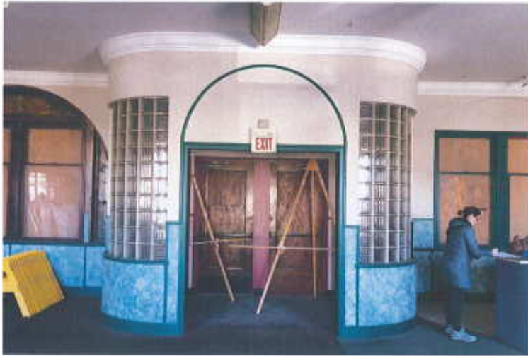
107. Room 102, looking into room 110.
