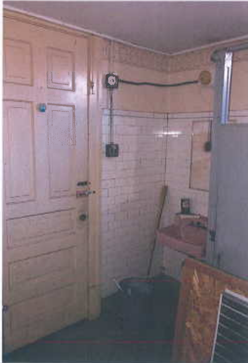
122. Room 104, historic tile wainscoting and wood door.
