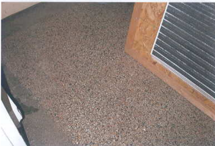
121. Room 104, historic terrazzo flooring.
