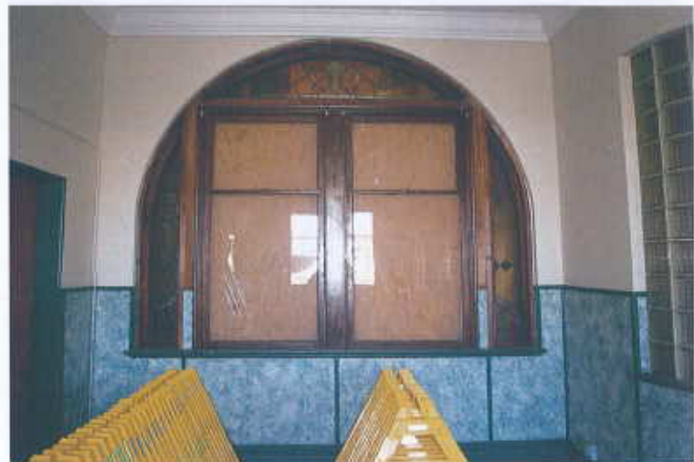
106. Room 102, historic window and stained glass sidelights and transom.
