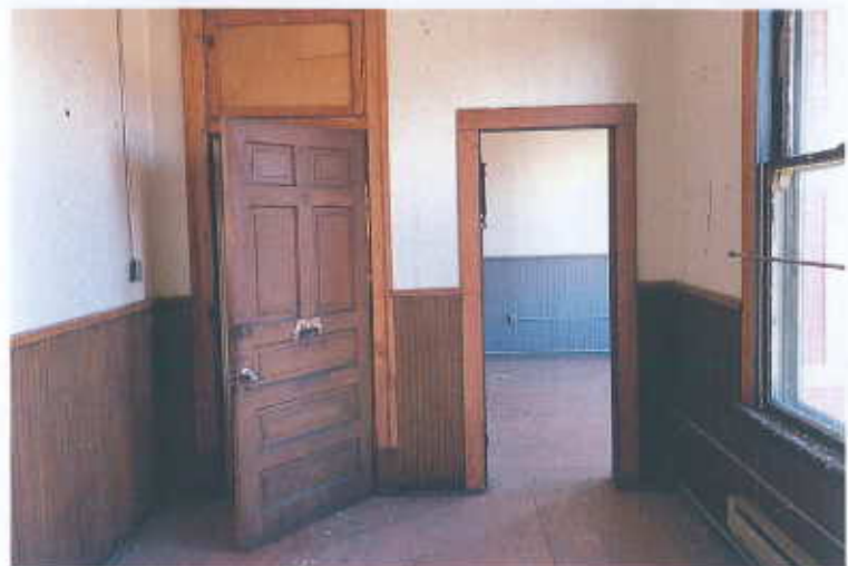
212. Room 207, historic woodwork (floor, wainscoting, 1/1 wood windows, interior doors and transom).
