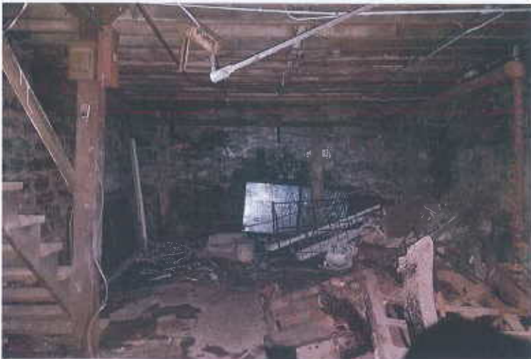
402. Basement, looking east.
