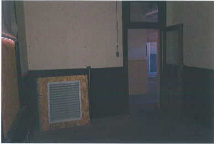
213. Room 209, historic woodwork (floor, wainscoting, interior door and transom).
