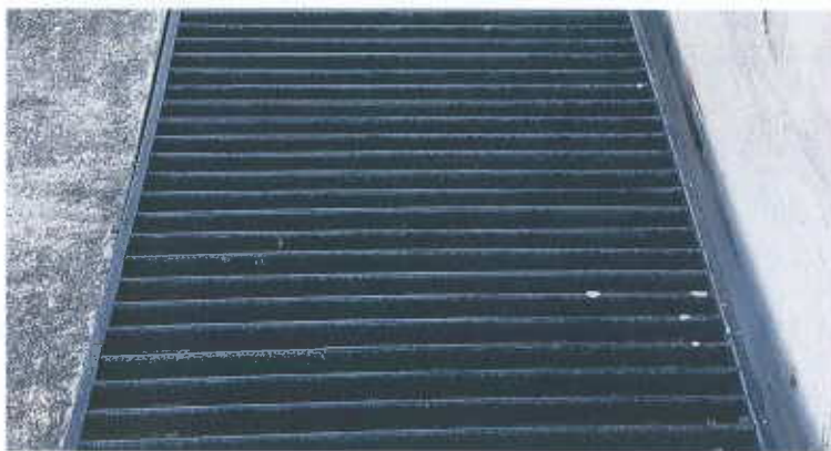
19. Detail, grate at west elevation.
