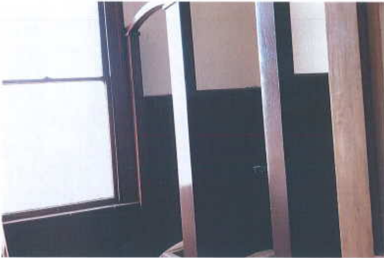
207. Room 203, historic woodwork.
