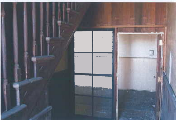
209. Room 205, historic woodwork.
