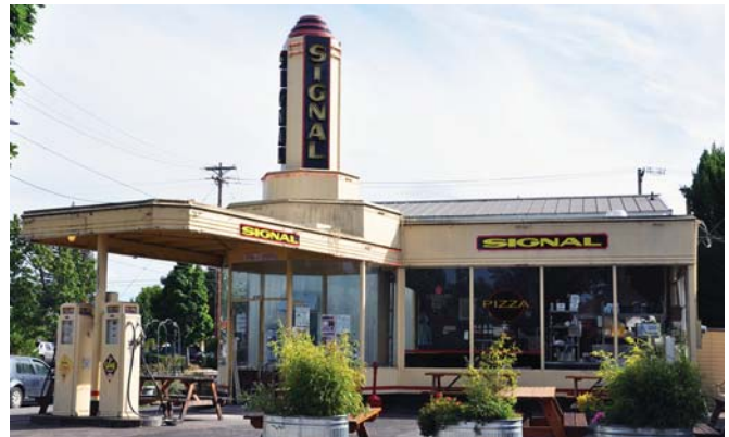
The adaptively reused Signal Station, in North Portland
