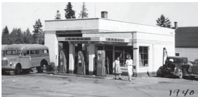
1940 image of the station, showing the rear addition
