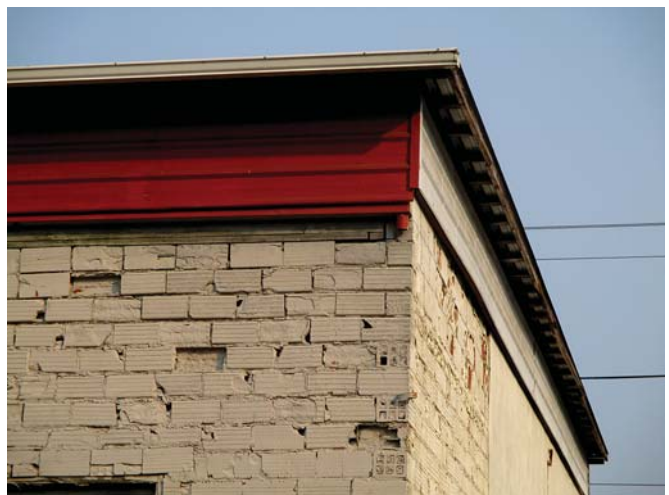
The metal sidewalls and metal roof structure at the SE corner
