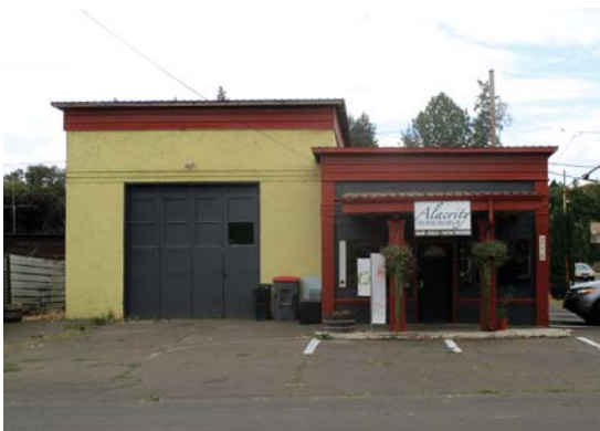
The north elevation with the garage at left, the office at right
