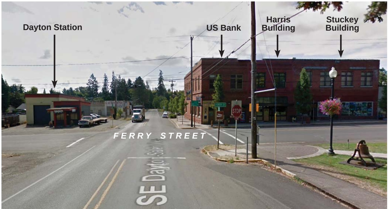
View looking down 3rd Street to buildings enfronting Ferry Street
