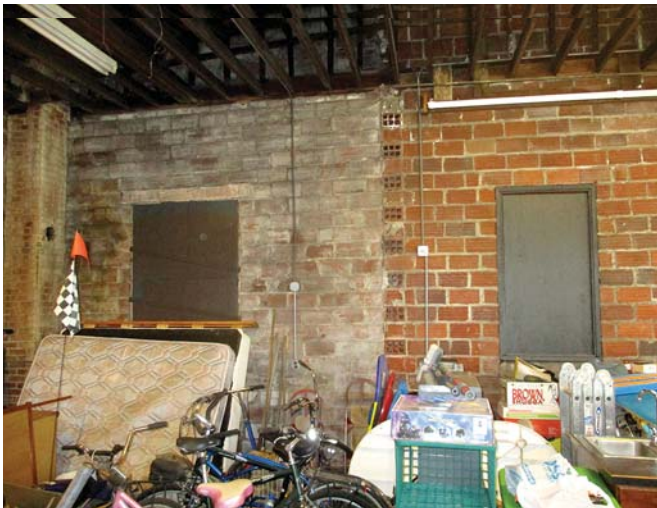
The pre-1940s addition (left) and the original garage wall (right)
