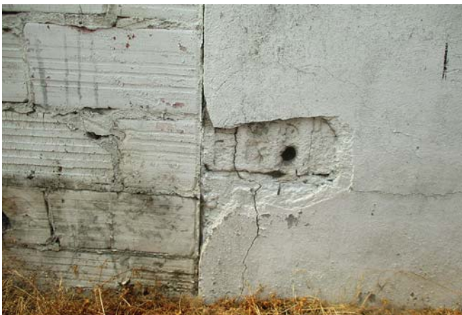
The joint between the addition and the garage, with its parge coating
