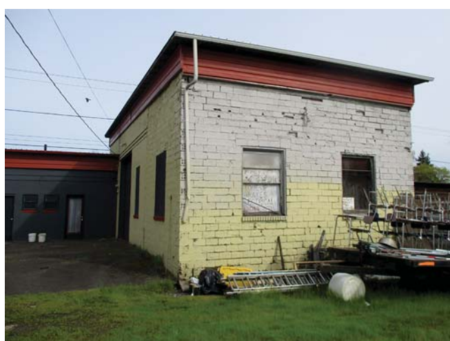
The south elevation of the garage, showing the pre-1940 addition
