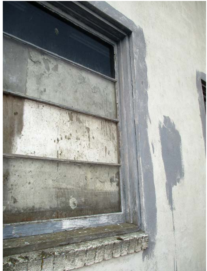
One of the east windows of the garage
