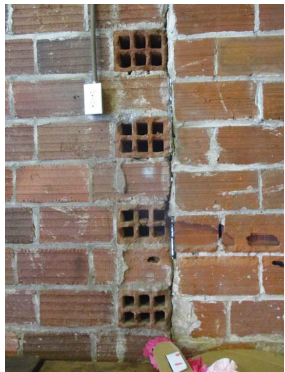
The cut south wall of the garage, and the joint with the addition
