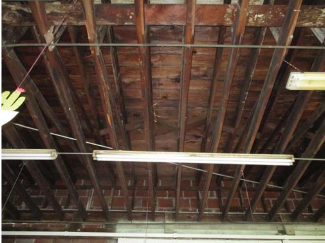
The roof framing of the garage
